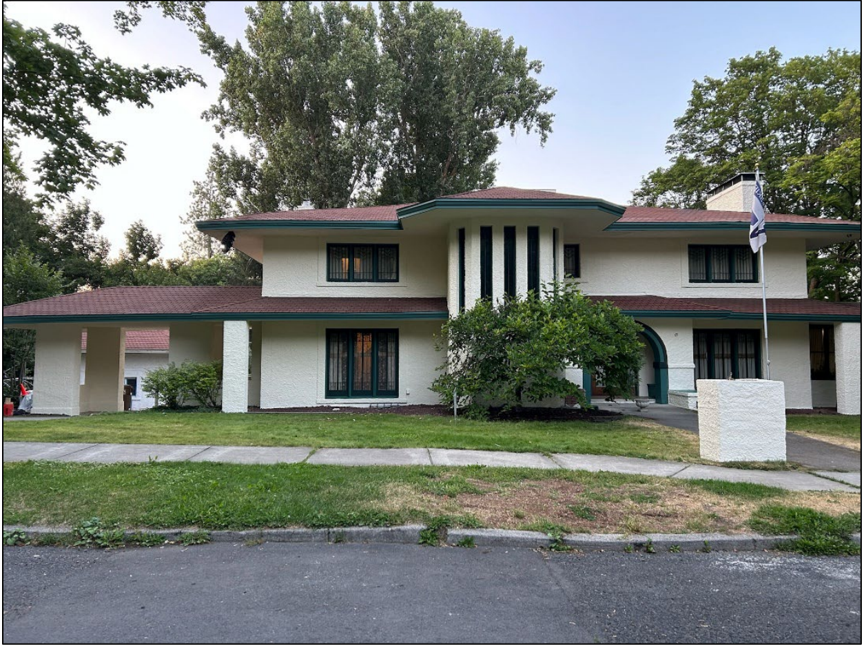
Photo 1 of 32: Front (south) façade, looking north
