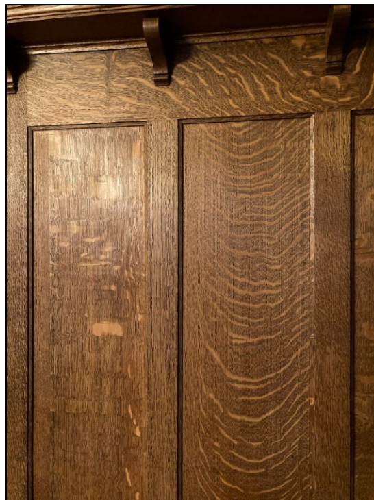
Photo 29 of 32: Detail of quarter sawn oak paneling, showing tiger stripes
