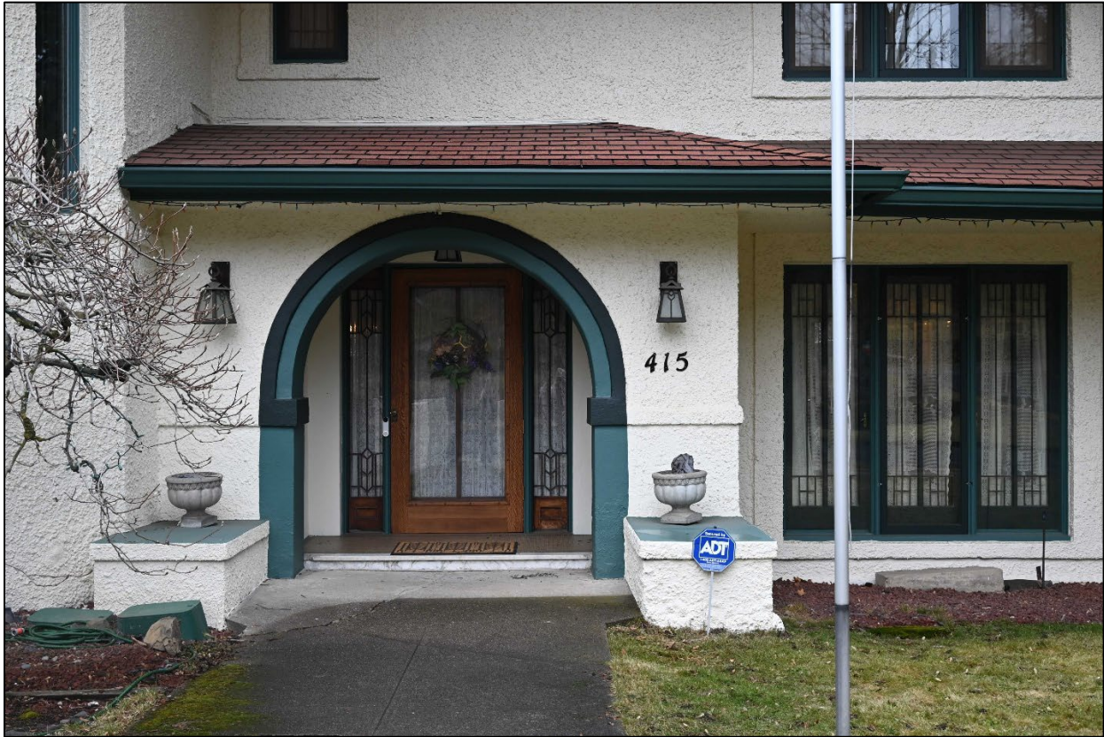
Photo 4 of 32: Front door showing mosaic, sidelights, oak storm door, looking north
