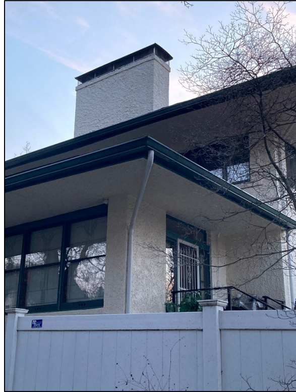
Chimney on east side, looking west
