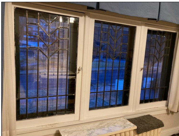
Windows showing Prairie Style leading
