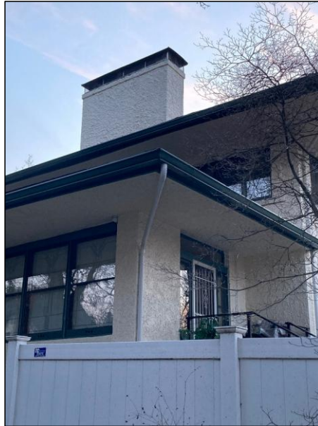
Chimney on east side, looking west
