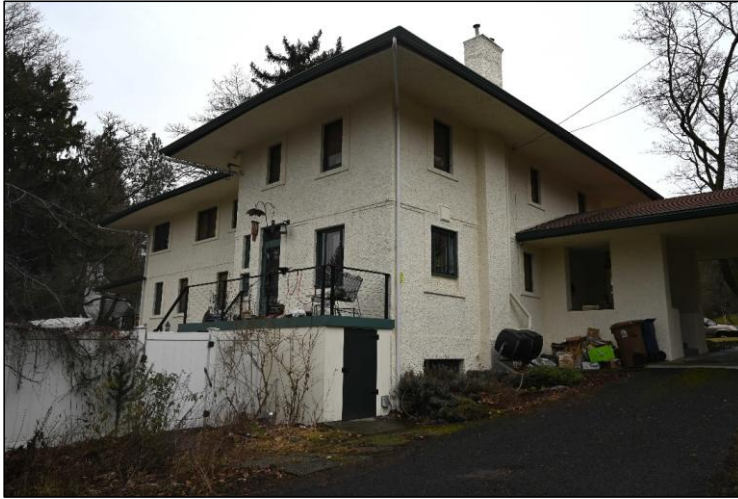
Rear (north) elevation, looking southeast
