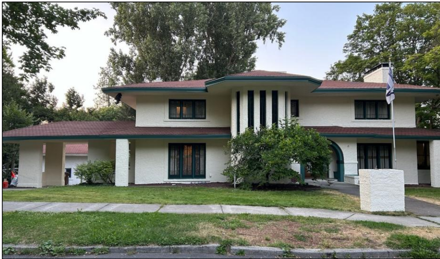
Front (south) facade of house, looking north
