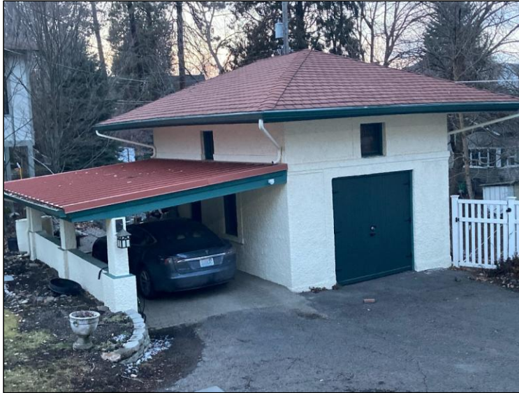
Garage and carport, looking northwest
