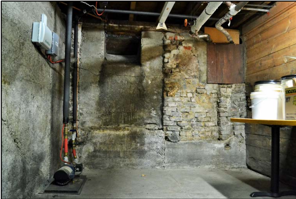
Figure 40. Residence, basement: Cutter & Malmgren Cellar (Rahn Basement) with coal chute in upper east wall; note combination of concrete and brick wall construction. View to the northeast.
