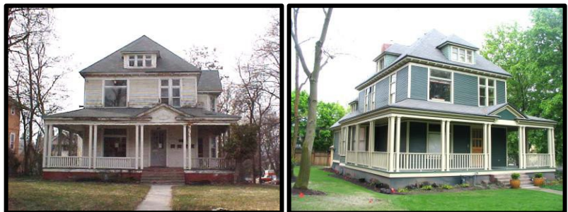
Thomas J. Graham House before and after rehabilitation.
