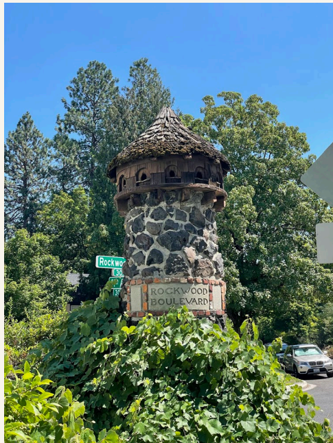
Design for entrance gate to Rockwood Boulevard addition. The piers and buttresses are to be built of rustic rock.
