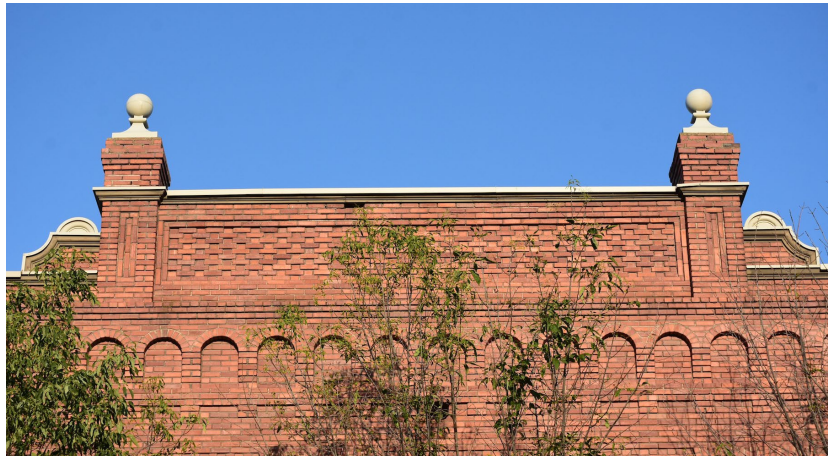
Figure 5: Parapet terminating east elevation
