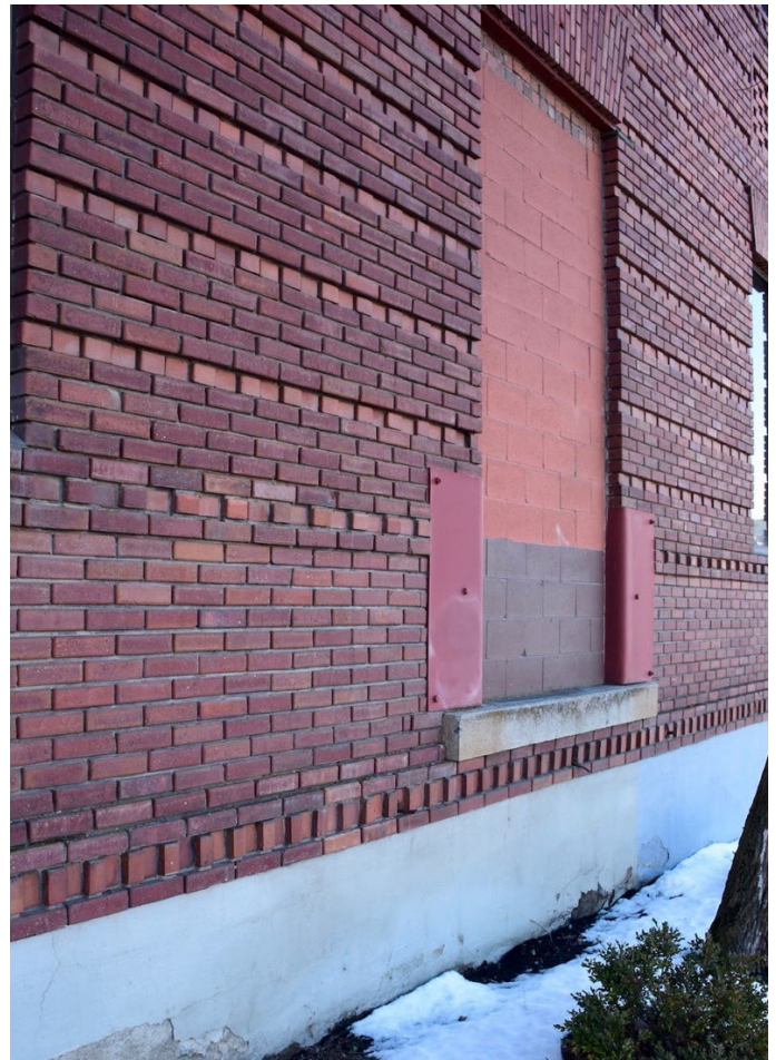
#8. Detail of east facade brickwork, looking southwest
