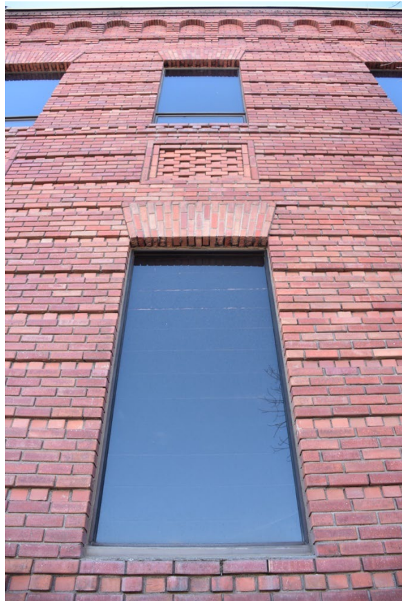
#6. Wall and parapet detail at southeast corner, looking west
