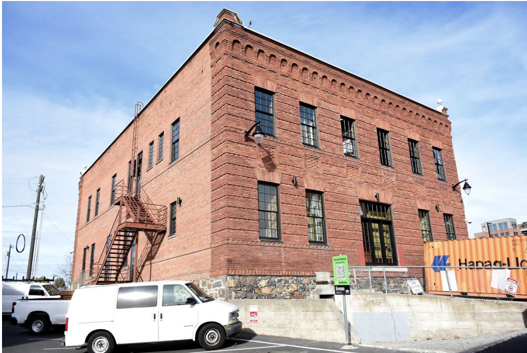
11. Southwest corner - looking northeast
