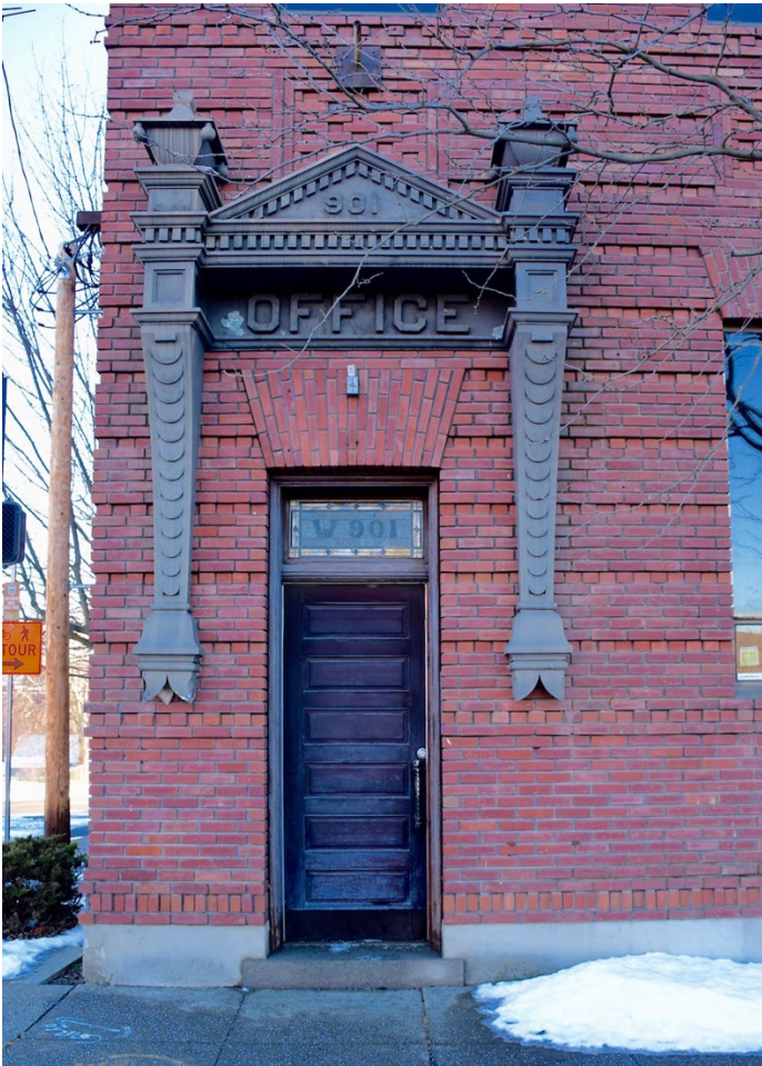
#7. Front Entry, original, looking south
