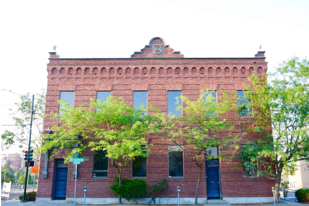
#1. Front (north) facade, looking south
