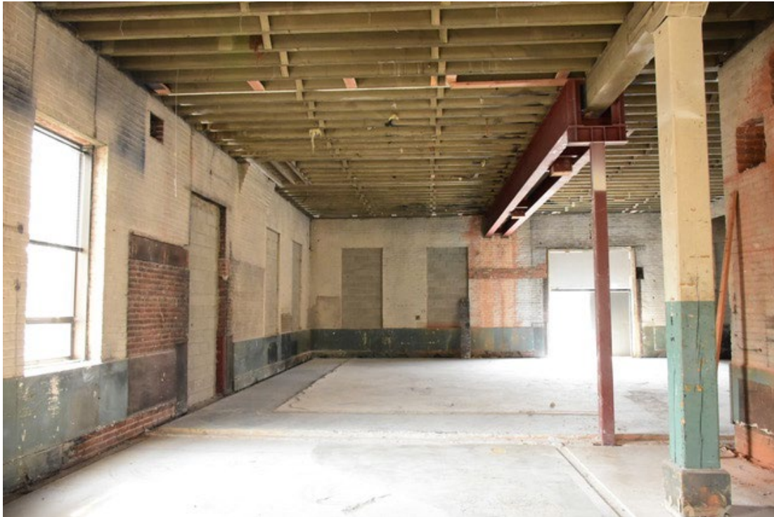
11. First floor, looking south along east walls-blocked-in windows
