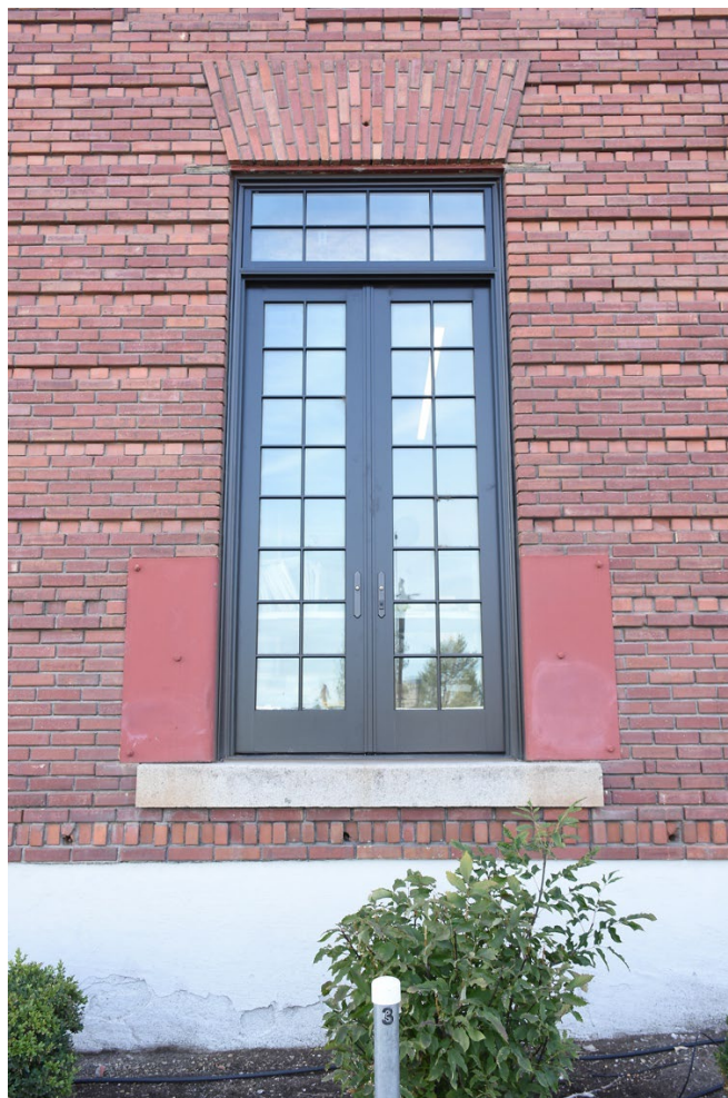
6. East facade, loading door reopened - Looking west
