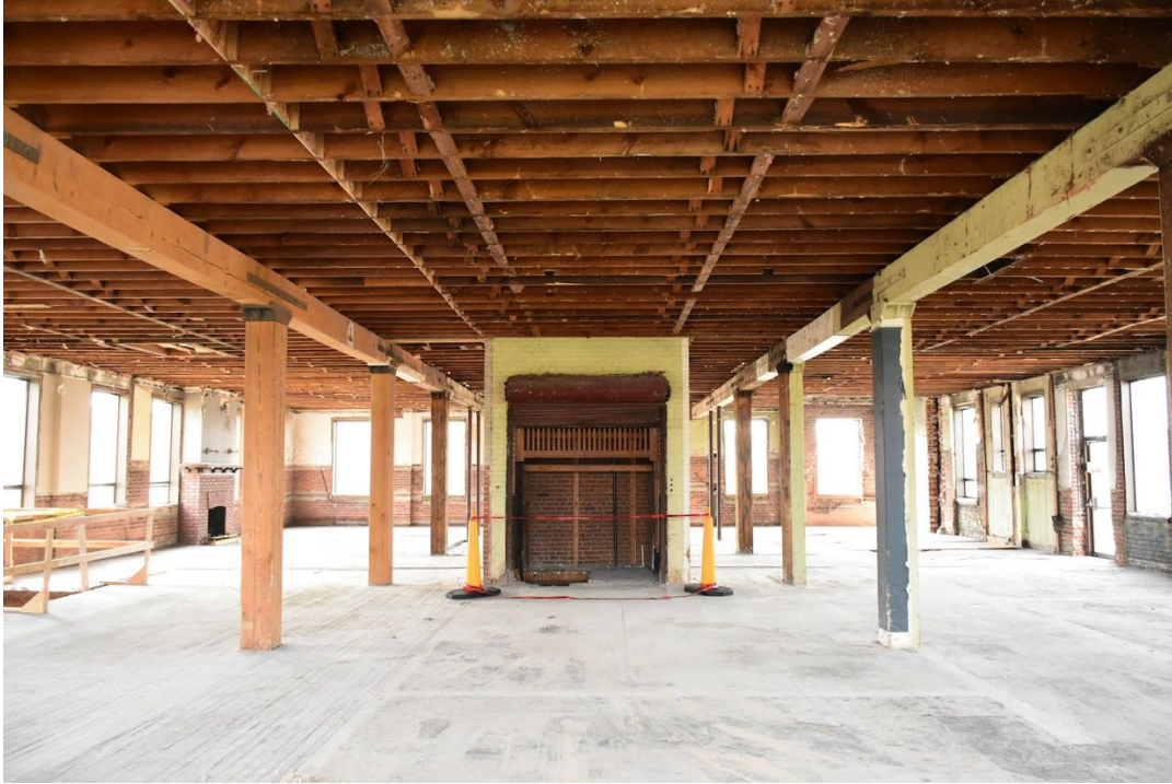
15. Second floor, looking south across room (freight elevator) from north wall
