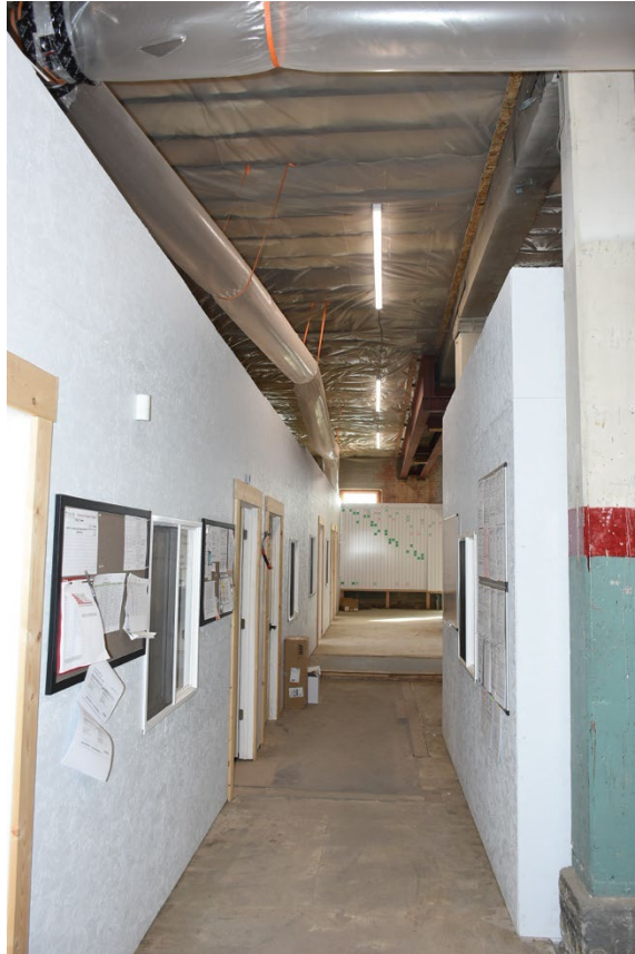
15. Construction offices (temporary) looking south along east side
