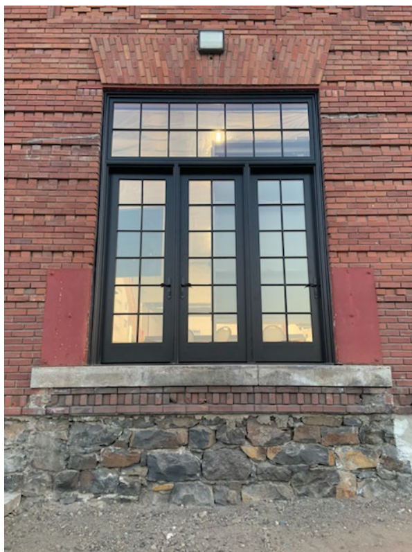
10. Rear loading door (dock removed, doors replaced)- looking north
