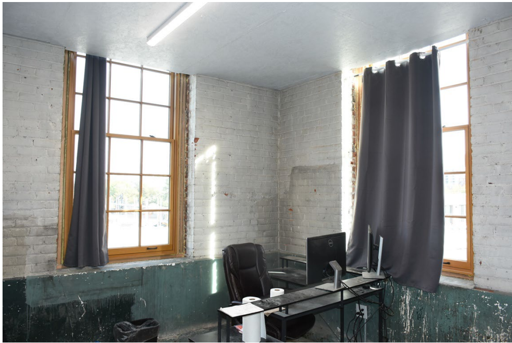
13. Interior First floor, southeast corner (concrete blocks replaced) - looking southeast
