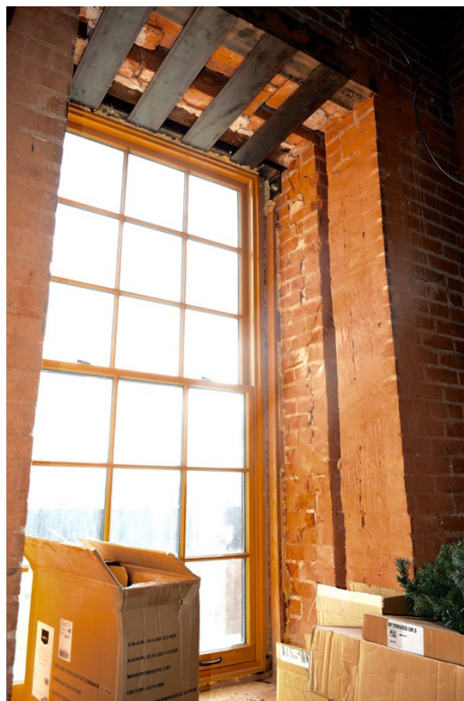
14. First Floor - West end window reopened (brick wall cut to open) - looking southwest
