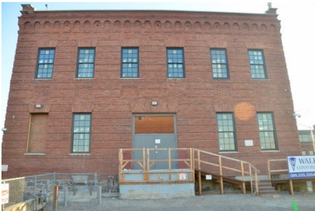
9. South Facade - work in progress - looking north
