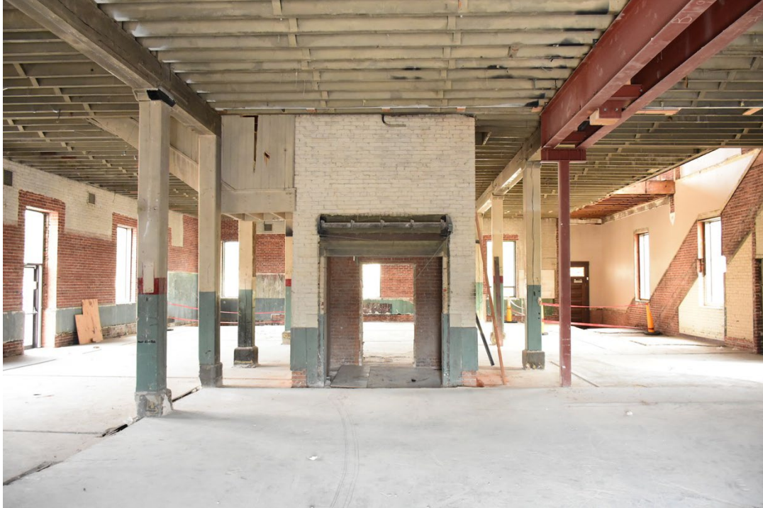
9. First floor, looking north from south wall
