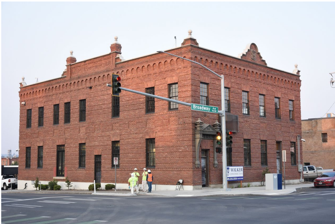
2. Northeast corner - looking southwest
