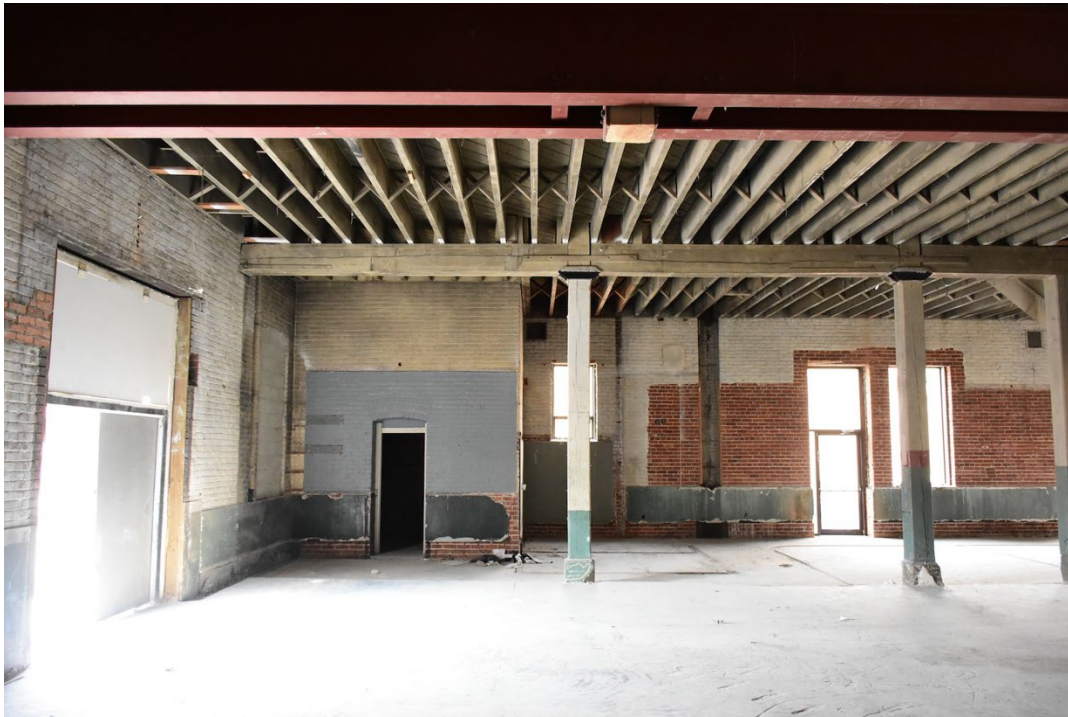
10. First floor, looking west at southwest corner
