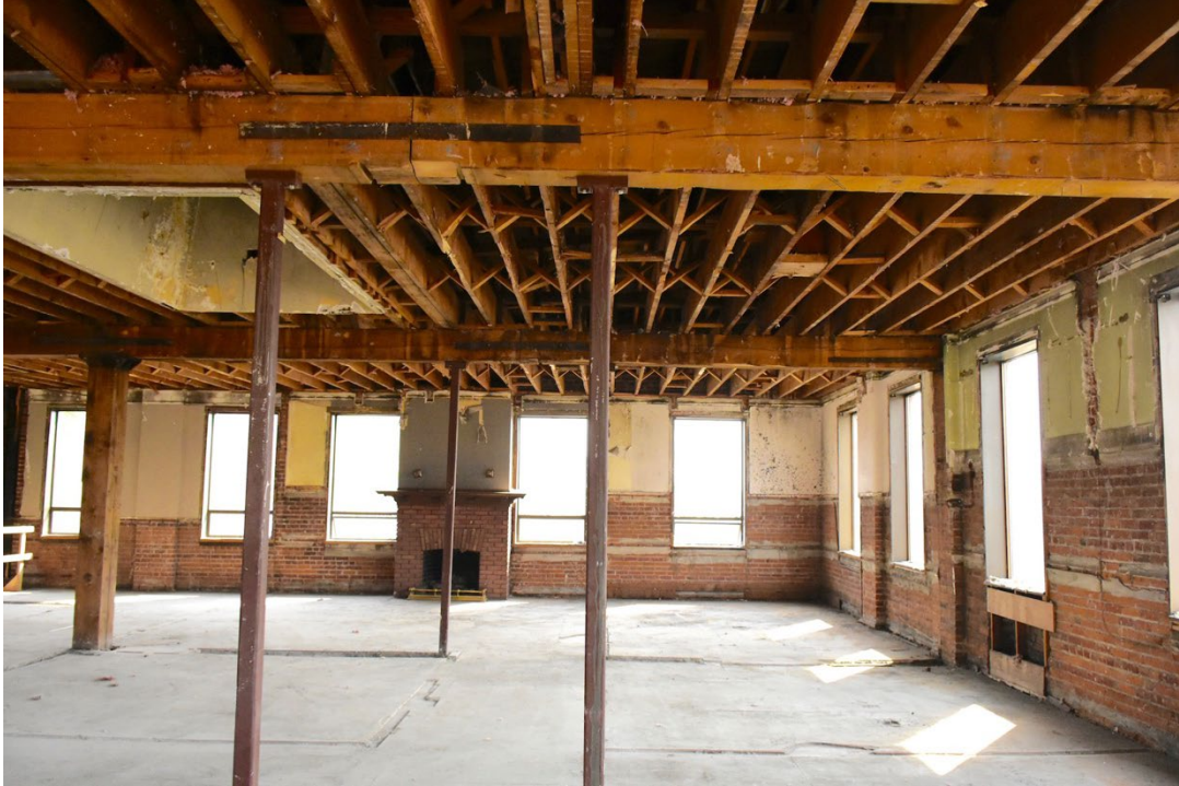
13. Second floor, looking east at southeast corner and fireplace
