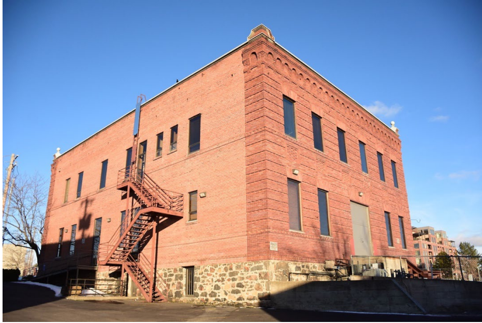
5. Southwest corner - south and west facades, looking northeast
