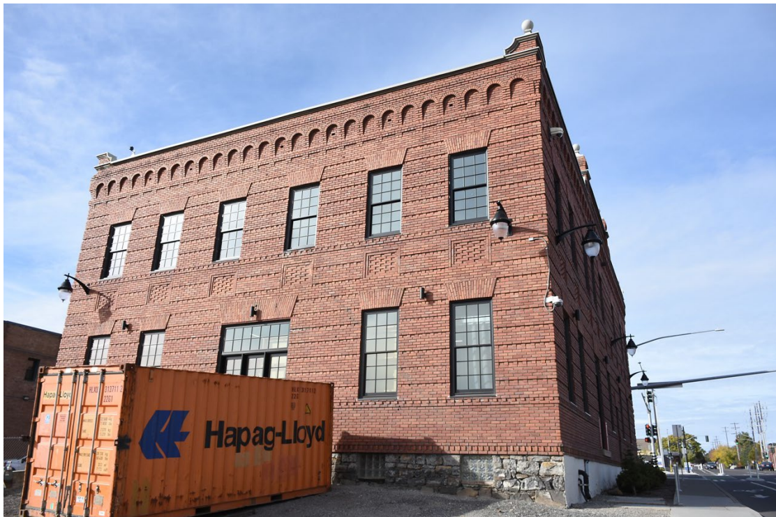
8. Southeast corner - looking northwest
