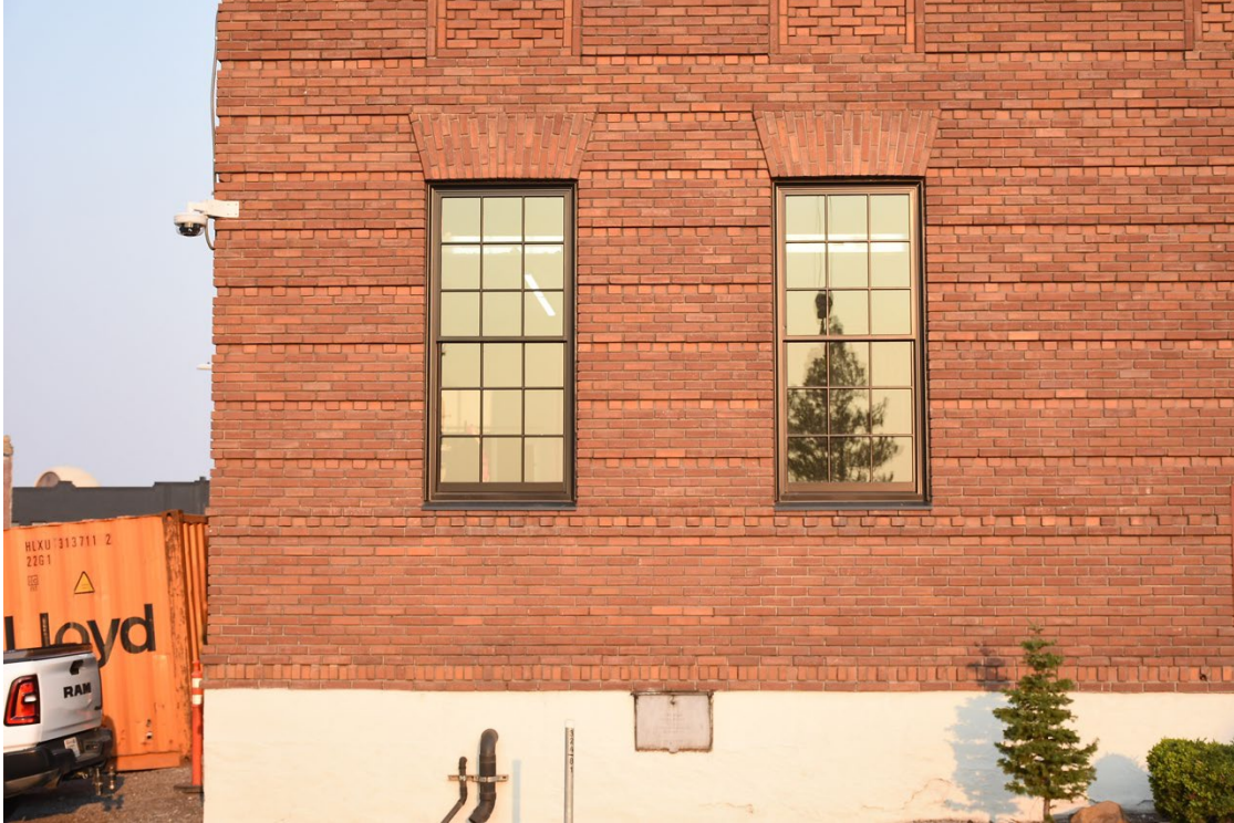
7. East facade, south end windows reopened - looking west
