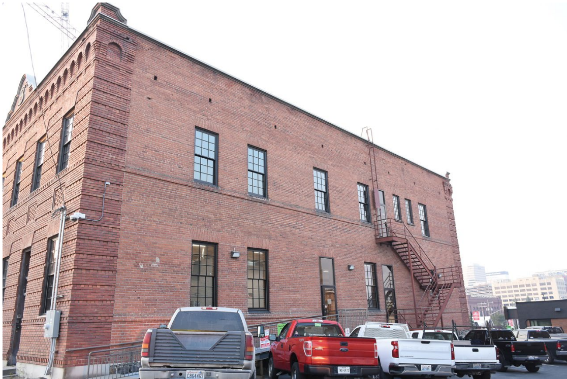
3. Northwest corner - looking southeast
