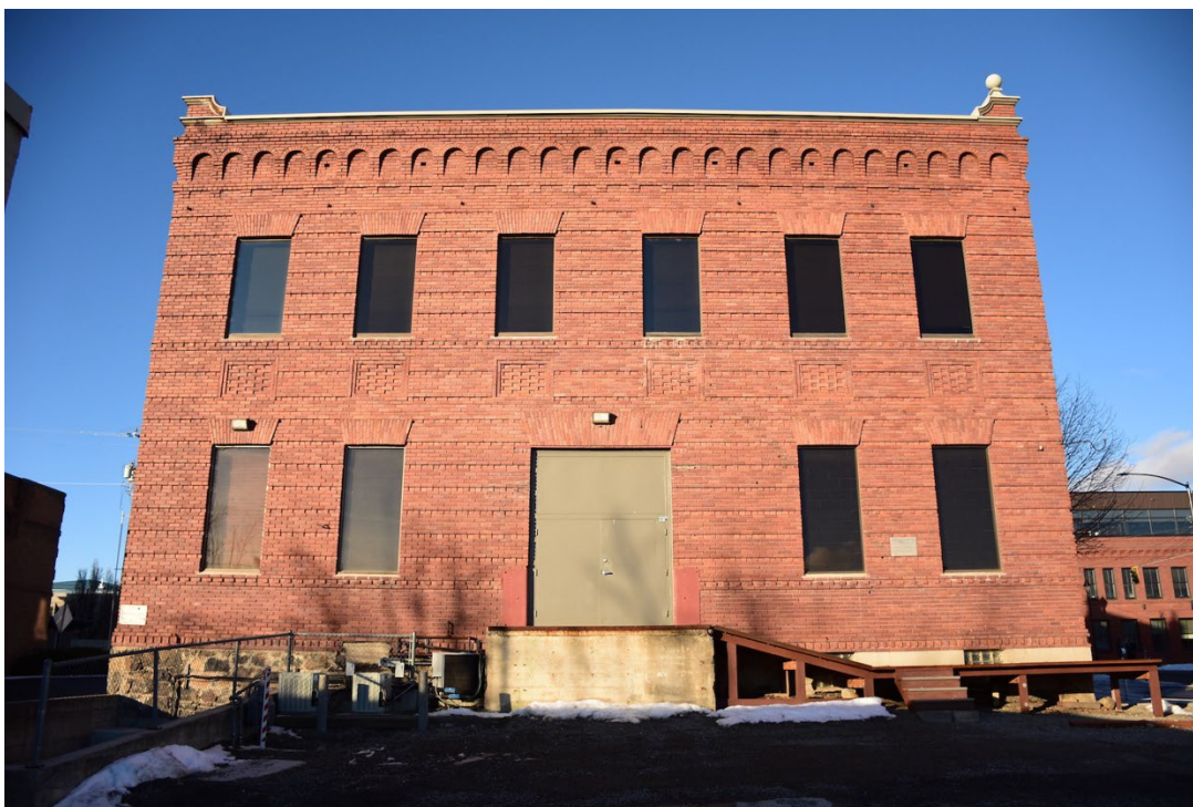
#4. South (rear) facade, looking north
