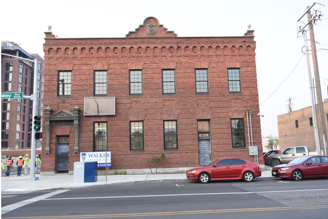
1. Front (North) Facade - Looking south
