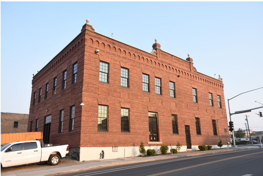
4. Southeast corner - looking northwest
