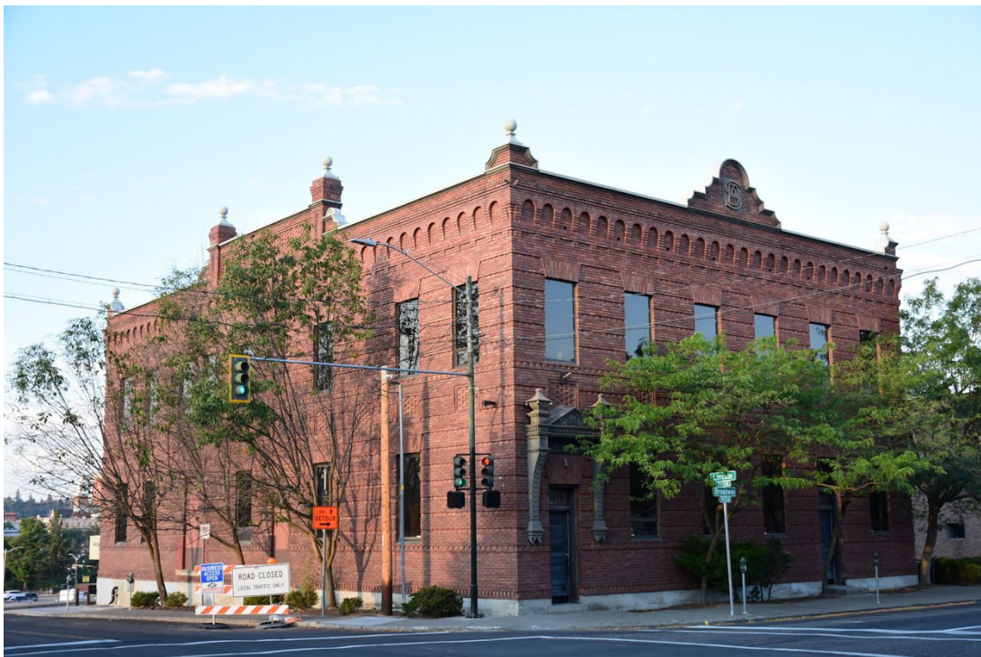
#2. Northeast corner - north and east facades, looking southwest
