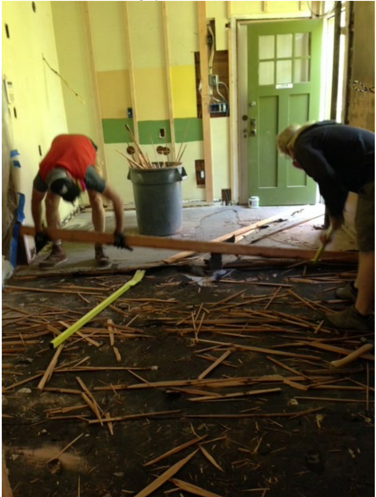
3floors.JPG – Three old flooring layers removed
