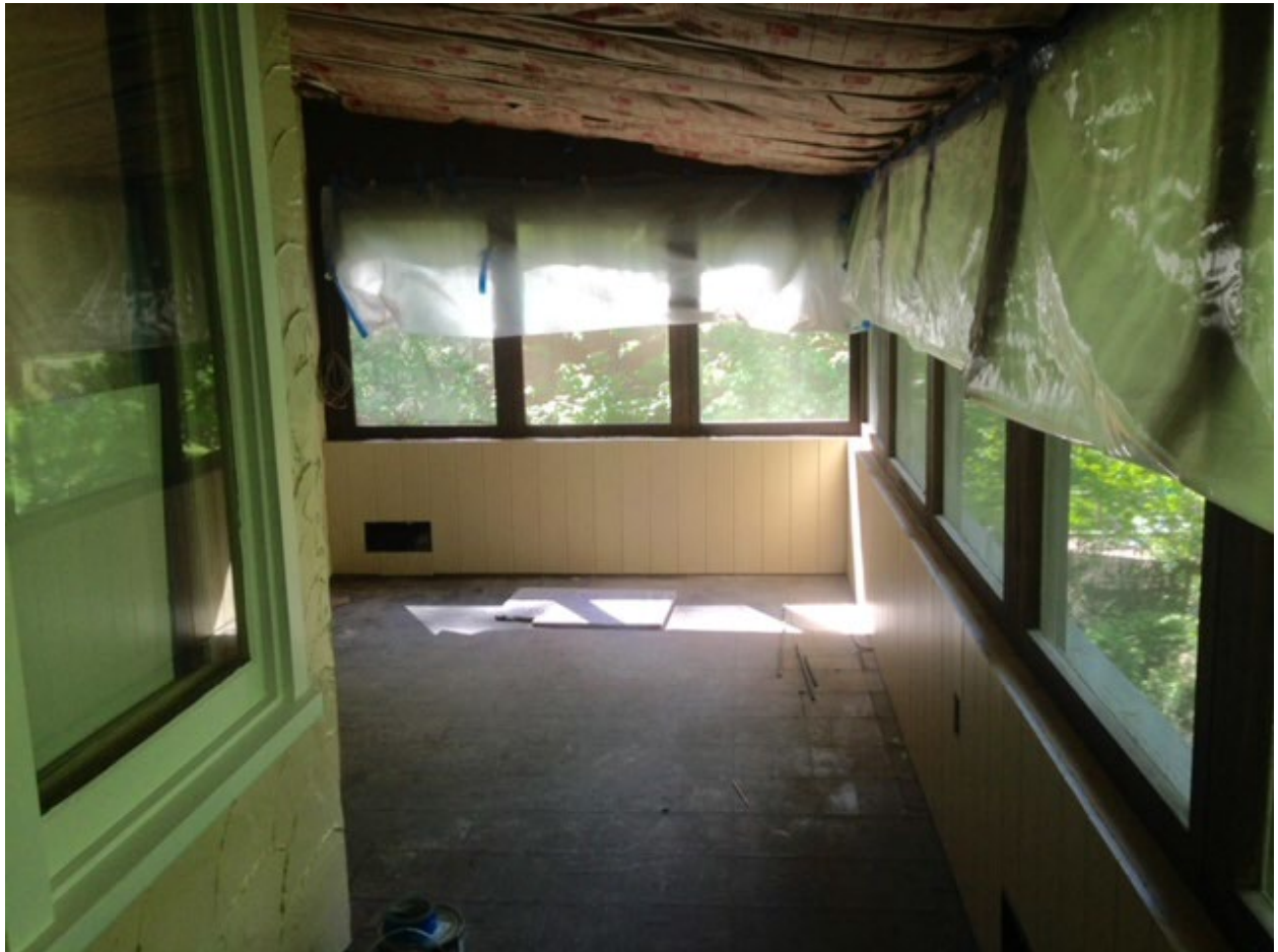
NWporch.jpg -Porch with new insulation before new floor
