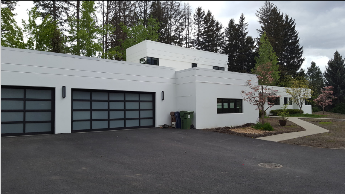
Photo 9: View of north façade of Thompson House in 2020
