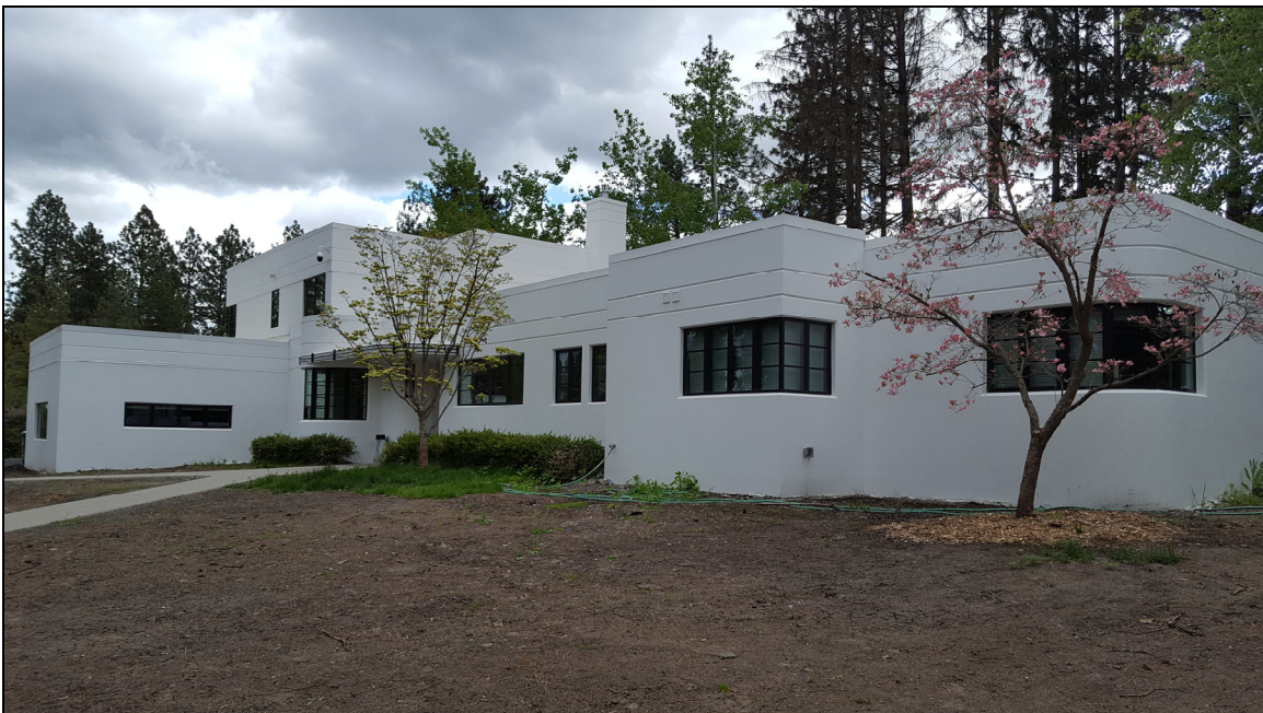
Photos 1 and 2: North façade of Thompson House in 2020, looking southeast
