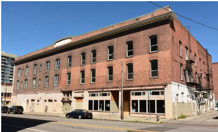
Figure 4: Jefferson - Southwest corner and west facade, looking northeast
