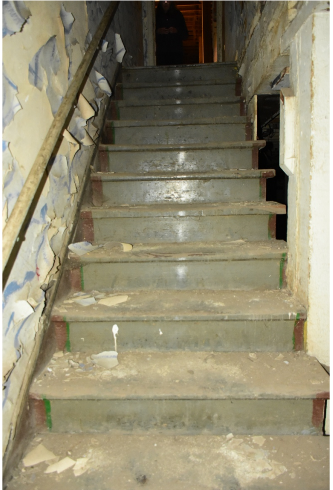
6b. Jefferson - Basement stairway from west side to first floor
