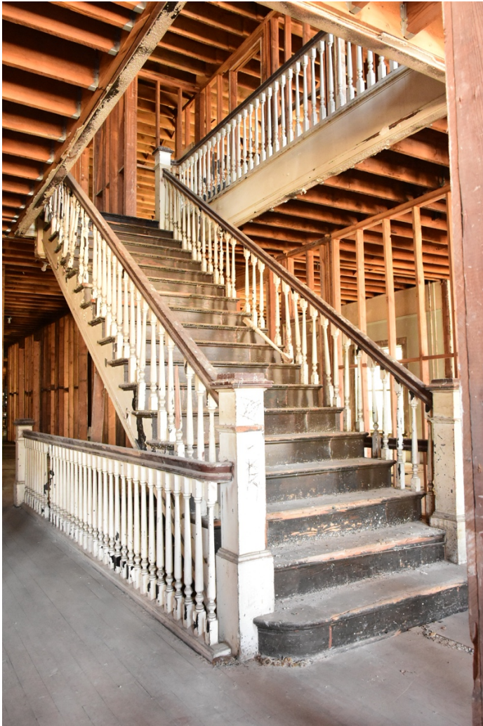
21. Norman 2nd floor, looking southwest at central stairwell.
