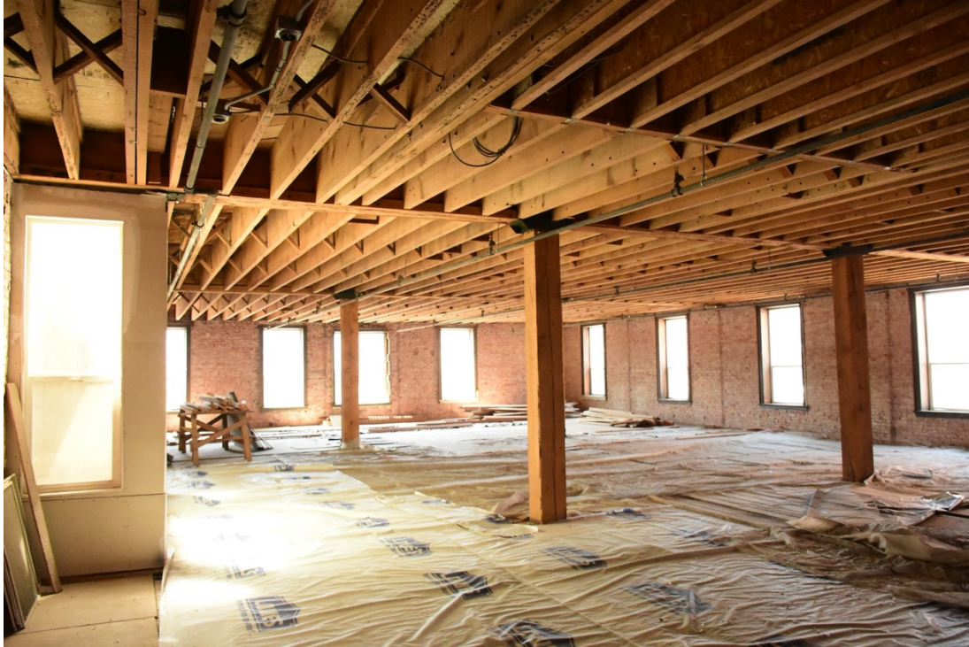
9. Jefferson 2nd floor, looking southwest from elevator/stair lobby
