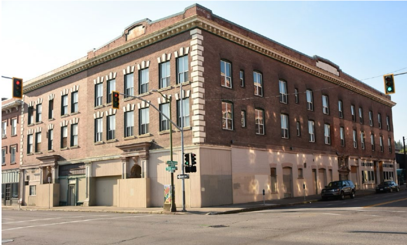
Figure 1: Norman-Jefferson - Northwest corner, looking southeast
