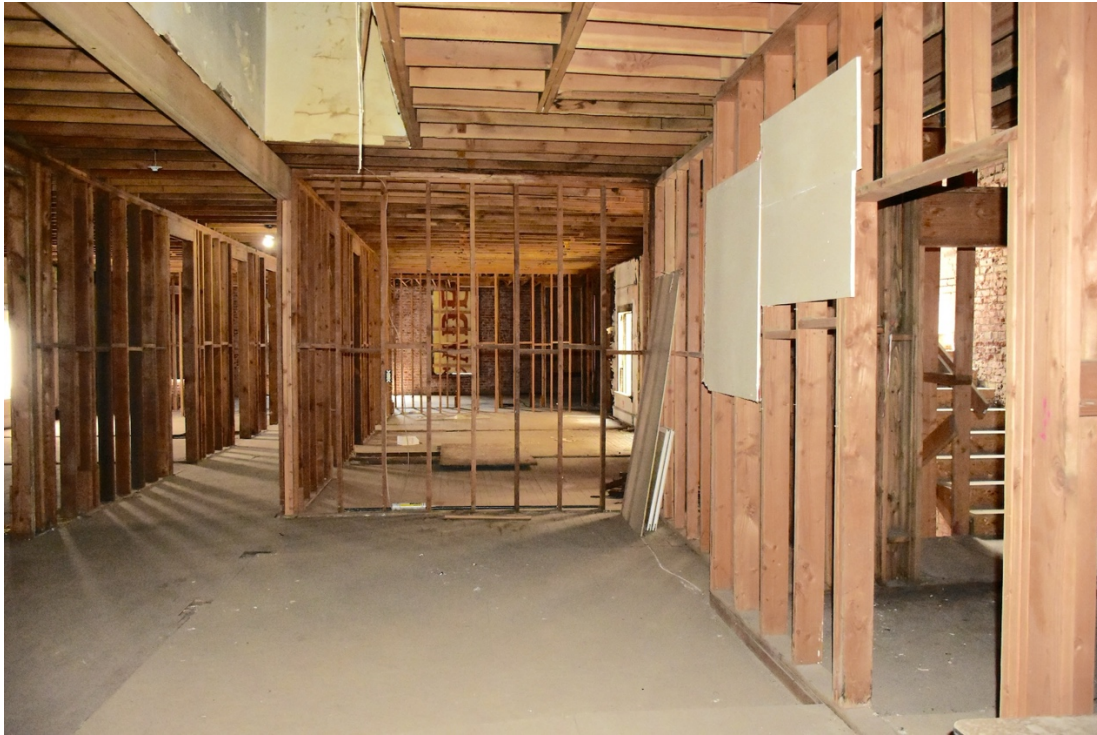
17. Norman 3rd floor, west side, looking south at elevator/stair lobby and original framing
