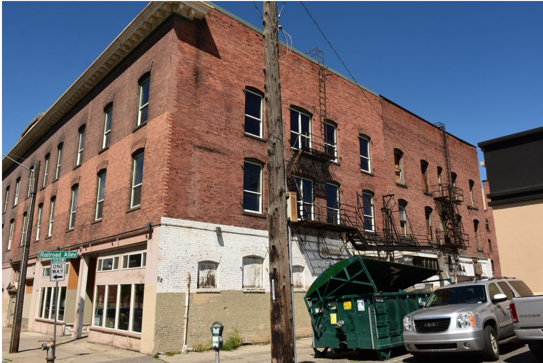
7. Jefferson-Norman - Rear (south) facade, looking northeast
