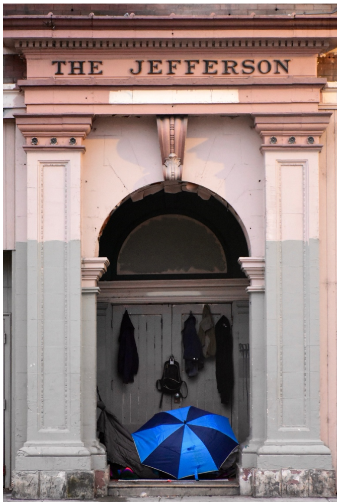
15. The Jefferson main entrance on 1 st Avenue, looking south
