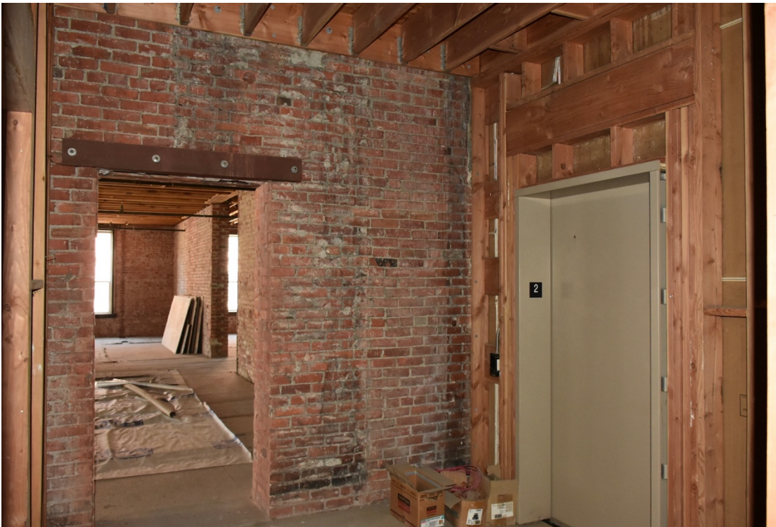
8. 2nd floor elevator/stair lobby, looking northwest toward Jefferson
