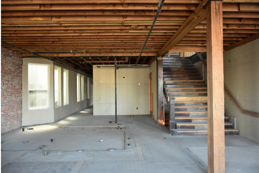
13. Jefferson 3rd floor - north section, looking south at midsection wall from stairwell
