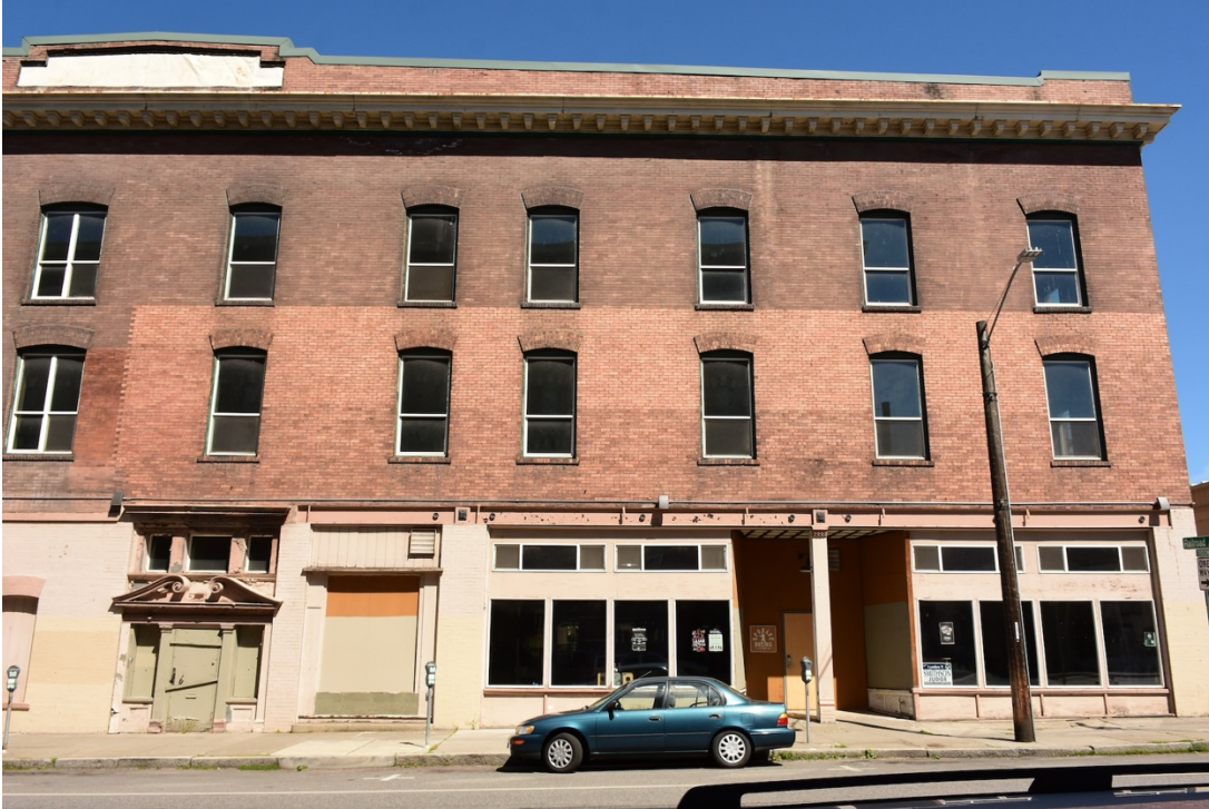
11. Jefferson - west facade, south section, looking east
