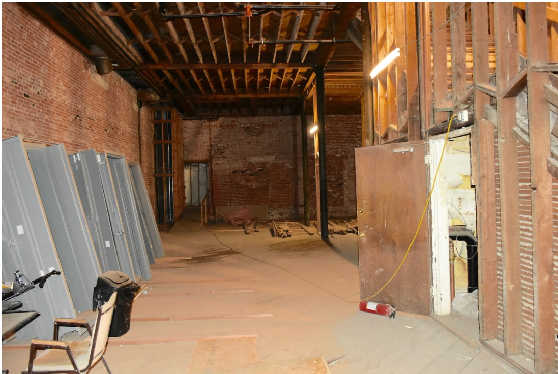
3. Jefferson First Floor - north section, looking south along east wall
