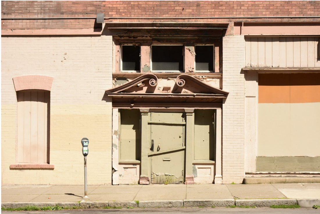
13. Jefferson - West facade, main entrance, looking east
