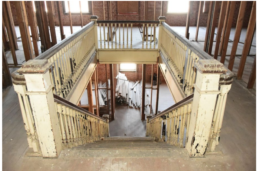
Figure 11: Norman 3rd floor, looking north at central stairwell
