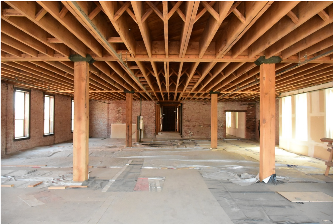
10. Jefferson 2nd floor south section, looking north from south wall
