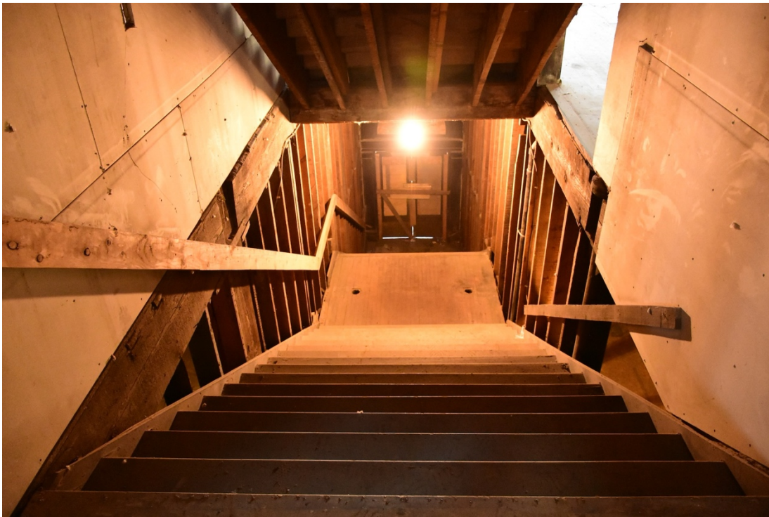
12. Jefferson central stairs 2nd floor to 1st floor
