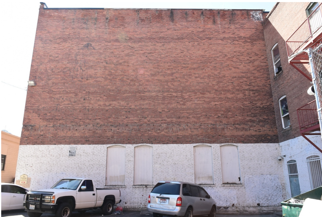
8. Norman - East facade, looking west
