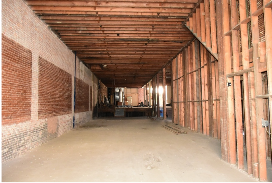
25. Norman 1st floor, looking south along east wall
