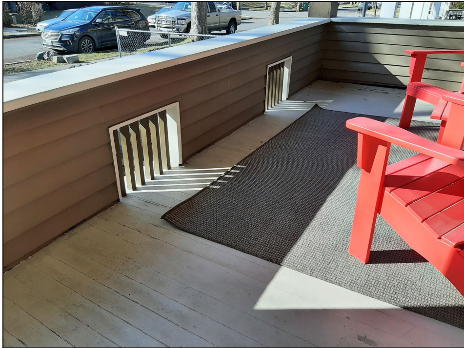
Photo 3 2022 photo of scupper detail on front porch
