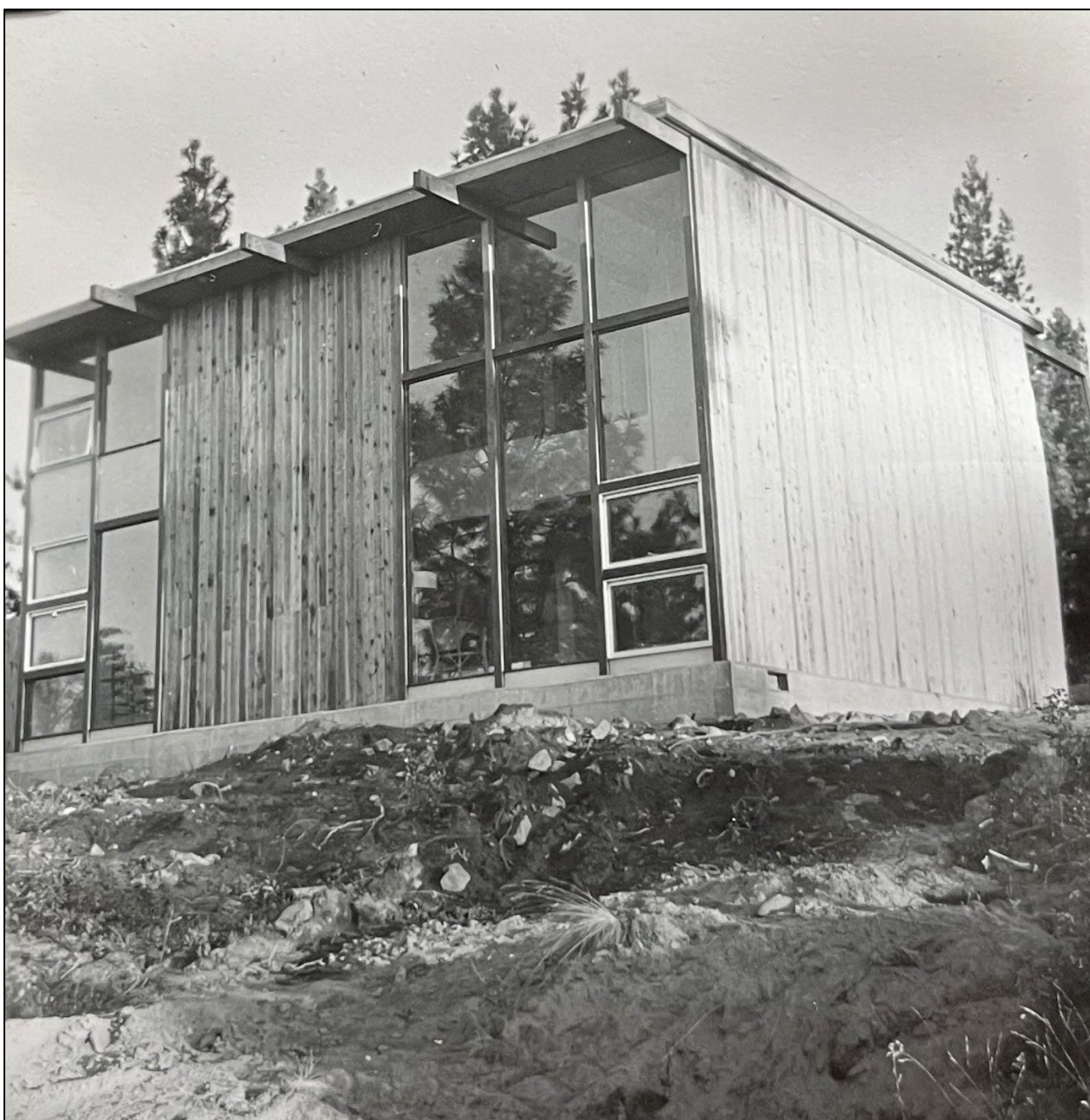
Figure 10: Phillips House post-construction photo, 1956
