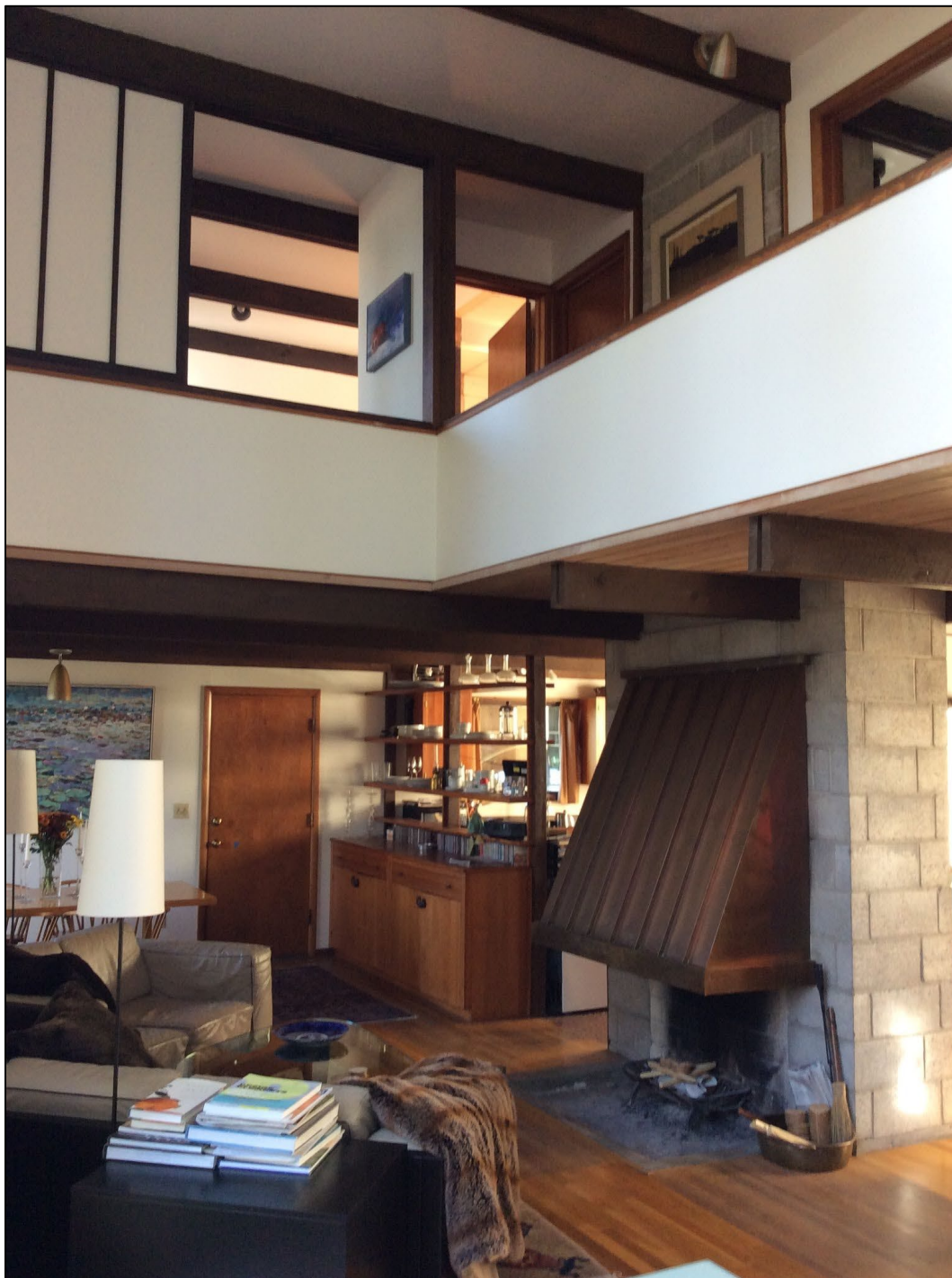
Figure 13: Photo showing Phillips House prior to renovation, 2018
