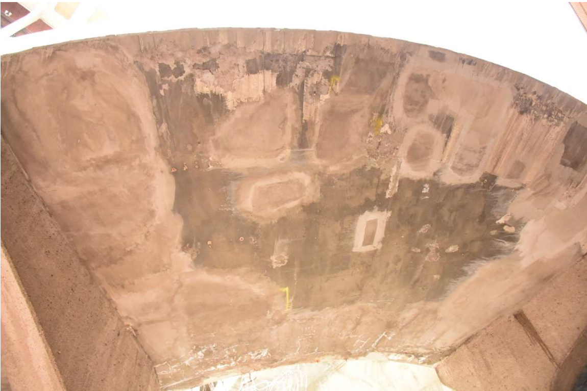
15. Southeast corner repair of underside of spiral exit ramp, looking east (6/2023)
