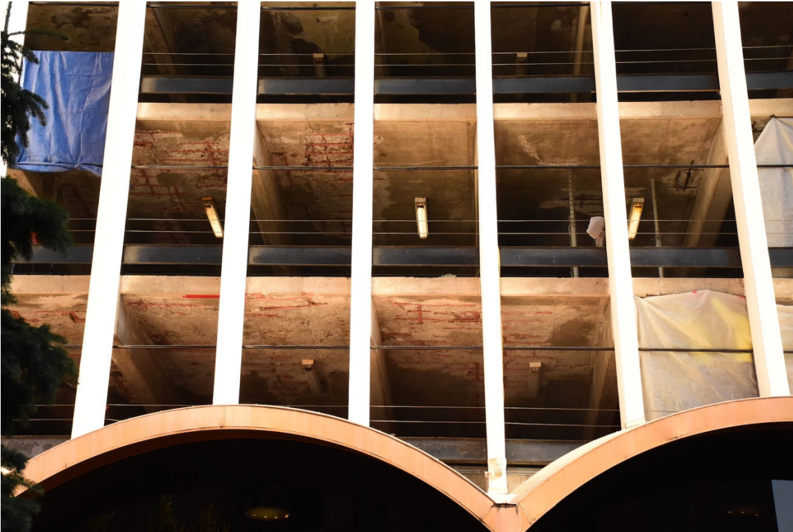
20. South facade - floors 3 and 4 west of tower- spalling concrete, looking north (9/2021)
