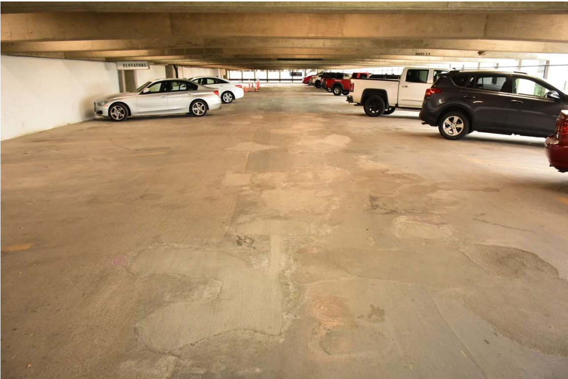
55. Brown level (floor 5) - floor repaired, looking west (9/2023)
