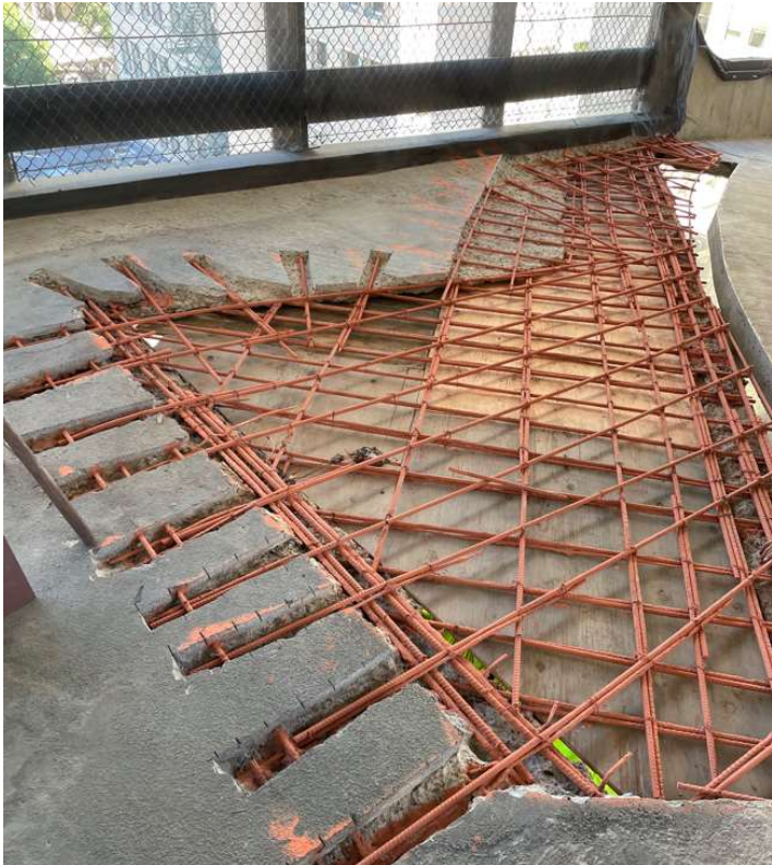
68. Yellow Level (top) lower exit -rebuild juncture with spiral ramp, looking southeast (6/2022)
