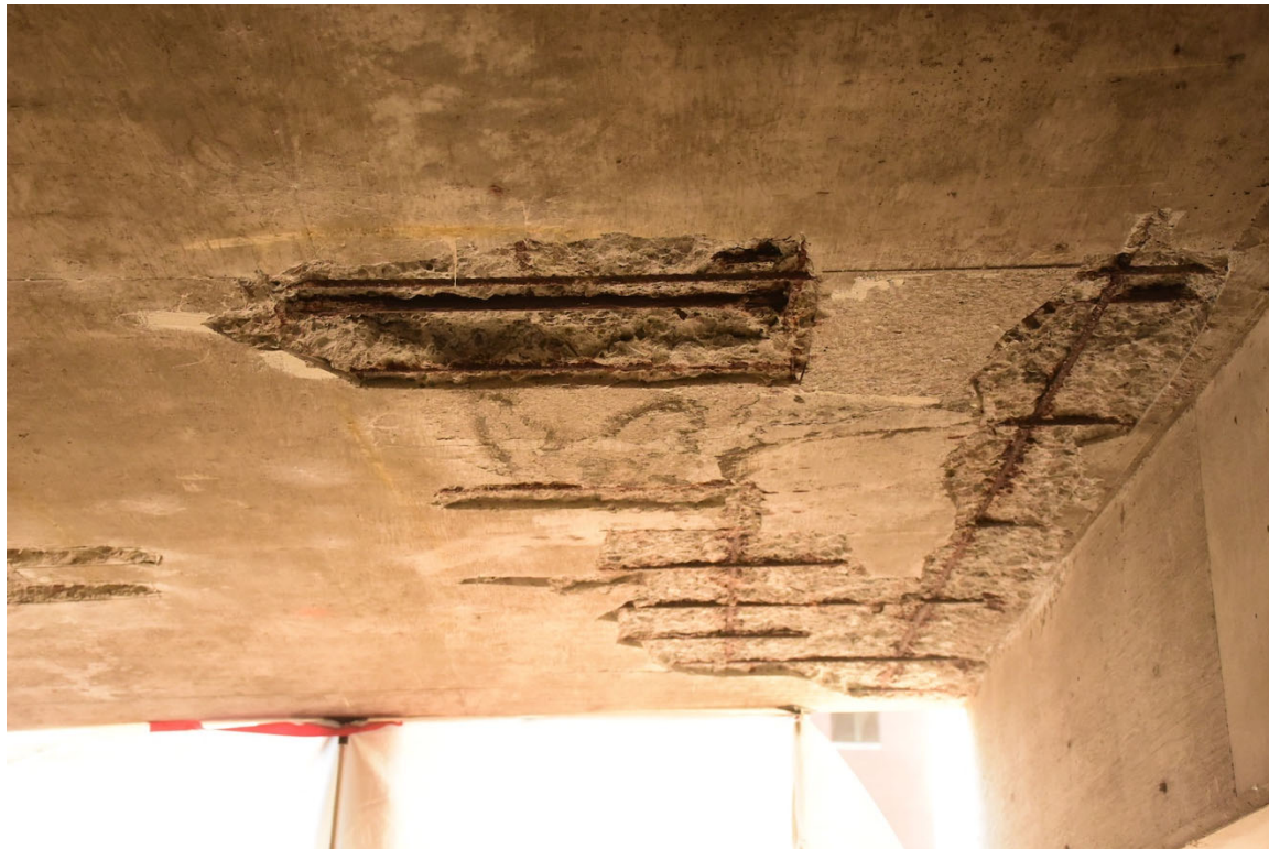
41. Red level ceiling (bottom of ramp) - condition of concrete and rebar, looking south (9/2021)
