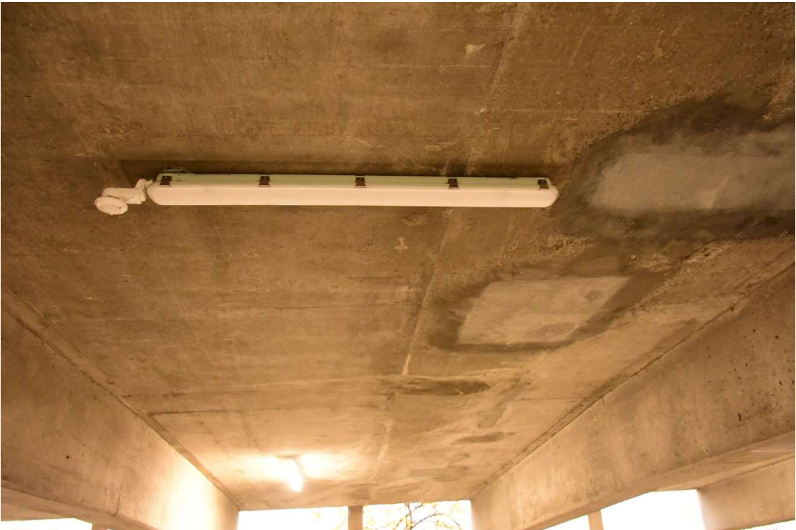
51. Blue level ceiling repair and new light fixture, looking north (10/2023)
