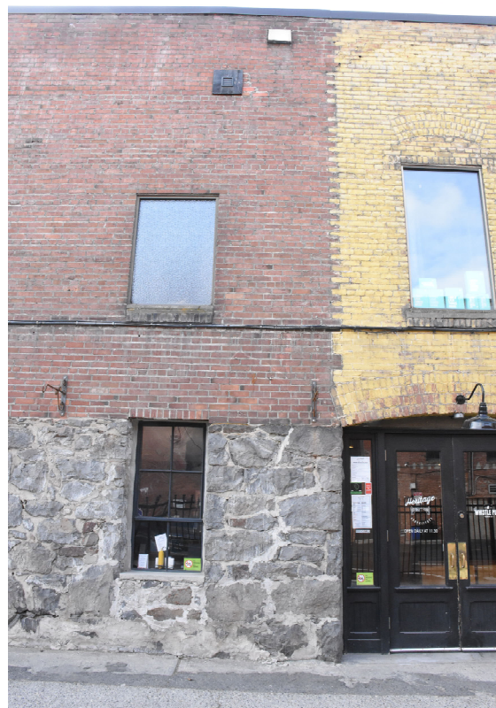
10. North facade - wall juncture (1910 & 1907)
