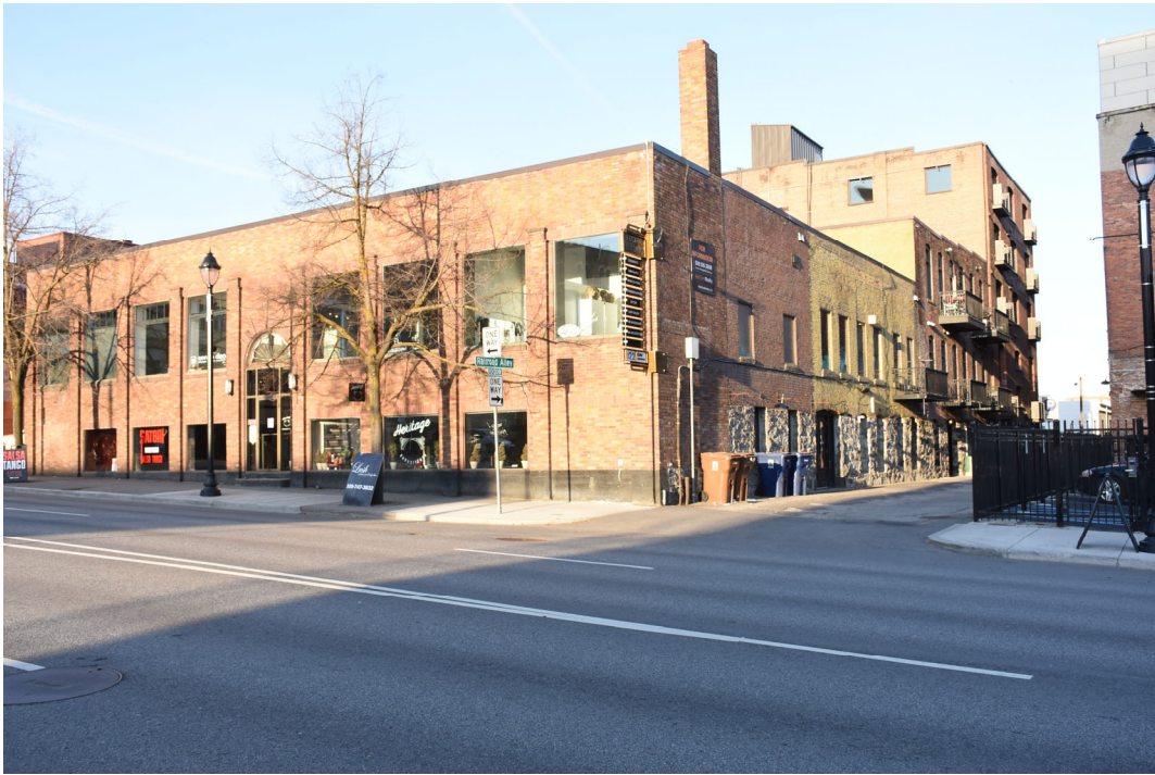
3. Northeast corner, and context along Railroad Alley Avenue
