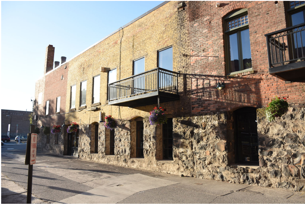
7. Northwest corner, looking SE along Railroad Alley (juncture with Washington Machinery on west)
