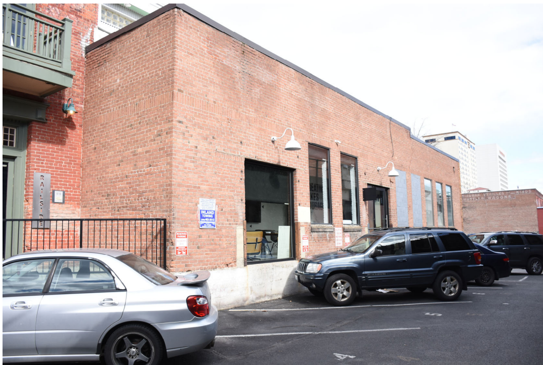
6. Southwest corner, looking northeast along BNSF viaduct alley
