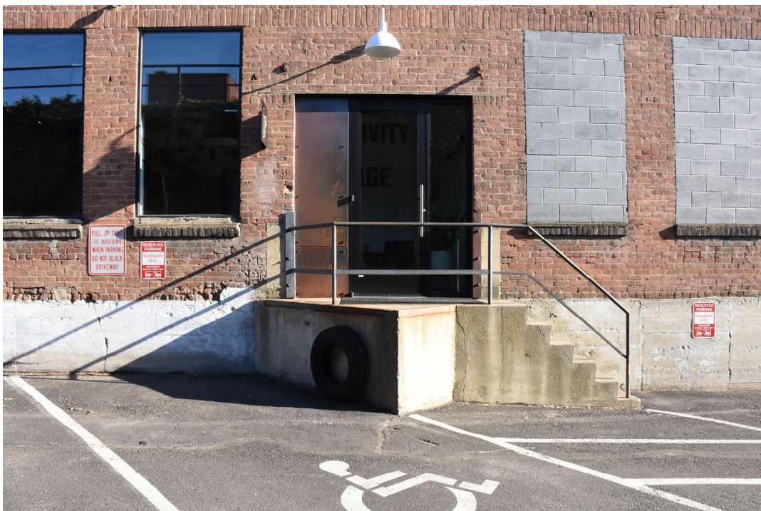
14. South facade - detail of side entry (former loading door and dock) and window bays
