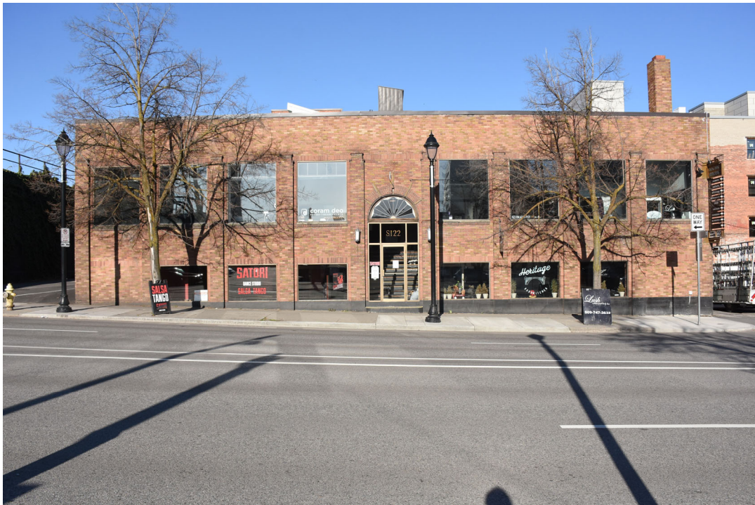
4. Front Facade along Monroe Street, looking west
