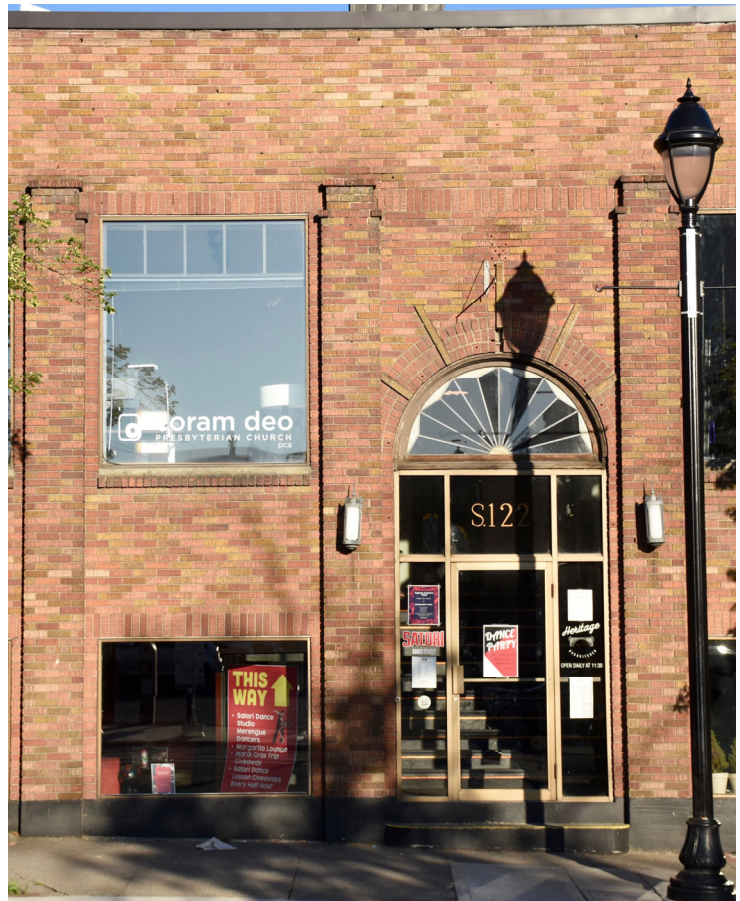
12. Front facade - detail of window bay, pilasters, and main entry
