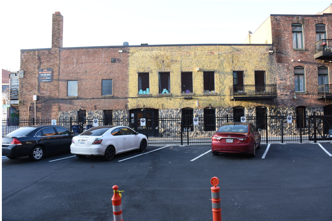
8. North facade along Railroad Alley (Washington Machinery on west), looking south
