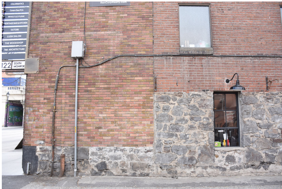
9. North facade-northeast corner showing wall juncture (1928 & 1910)
