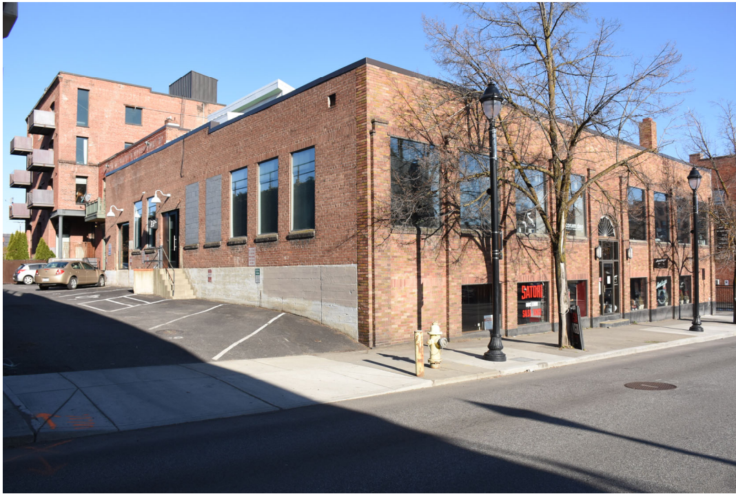
5. Southeast corner and context along BNSF viaduct alley, looking northwest
