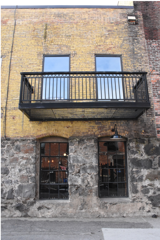
11. North facade - wall detail and juncture with Washington Machinery building
