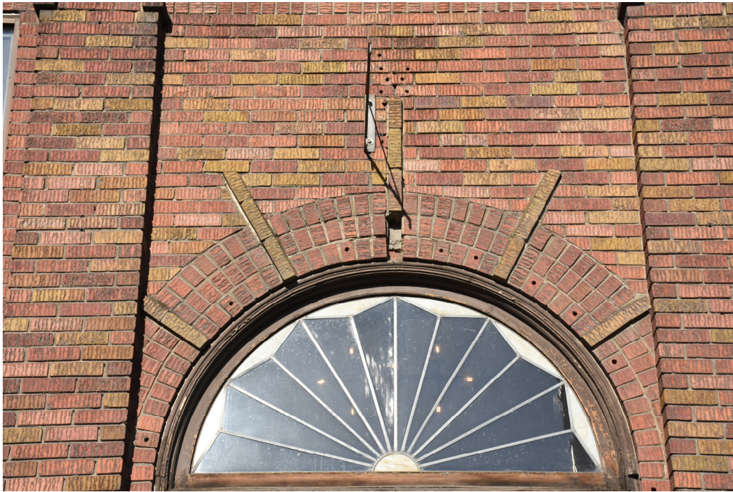
13. Front facade-main entry, detail of sunburst transom
