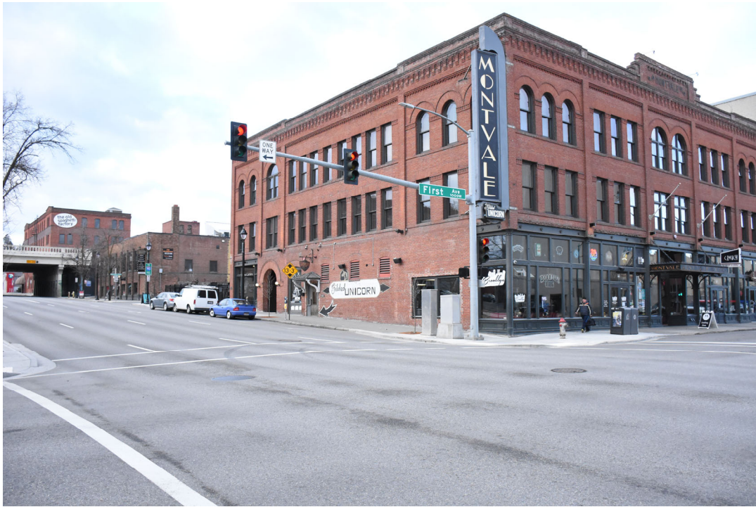
1. Context along Monroe Street, looking southwest
