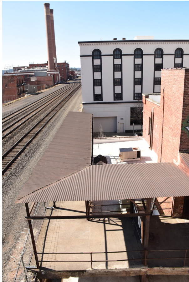
8. Roof top of warehouse - rail loading platform, looking west
