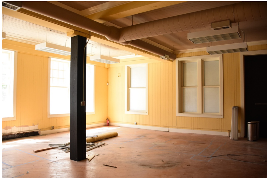
14. First floor office suite-northwest corner, looking northwest
