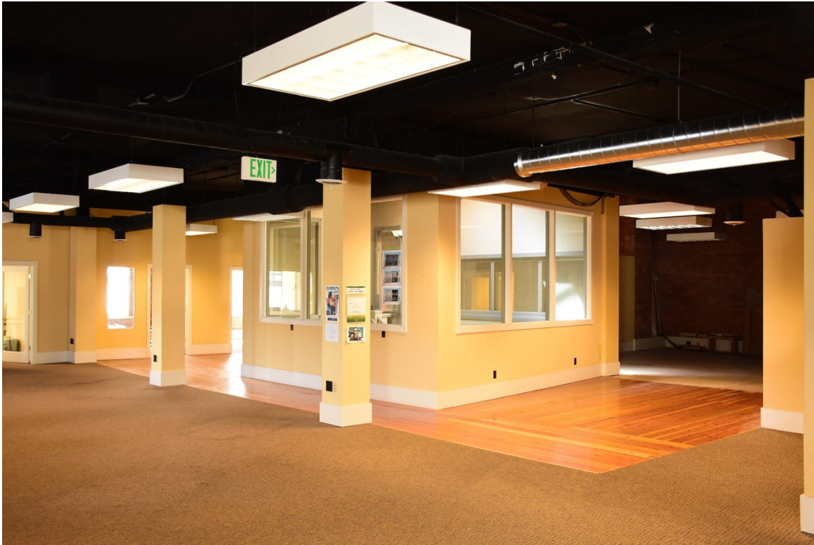
20. First floor Europa Restaurant, looking south toward Southwest corner entry (S125 Wall)
