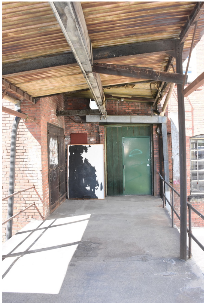
24. Rooftop loading platform entering tower and south wall, looking north
