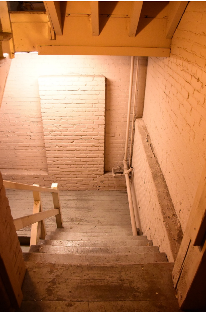
23. Original back stairs in northeast corner
