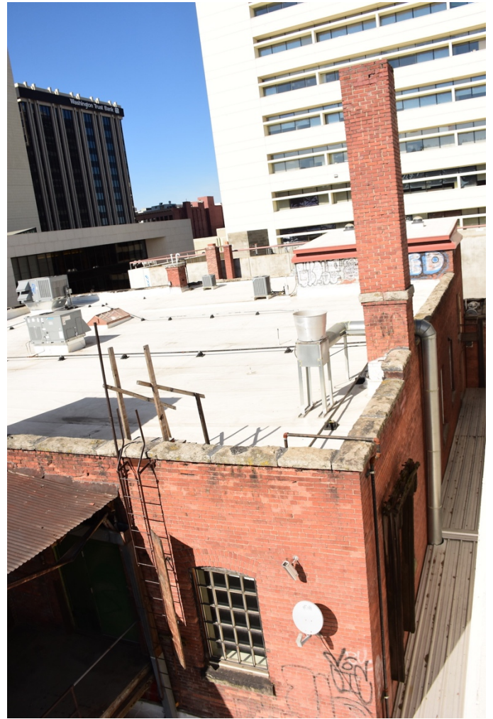
10. Southeast corner - east facade, looking north
