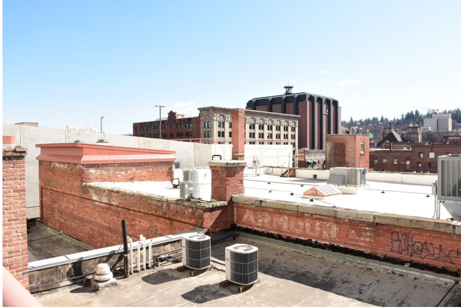
6. Southwest corner - front facade, looking northeast
