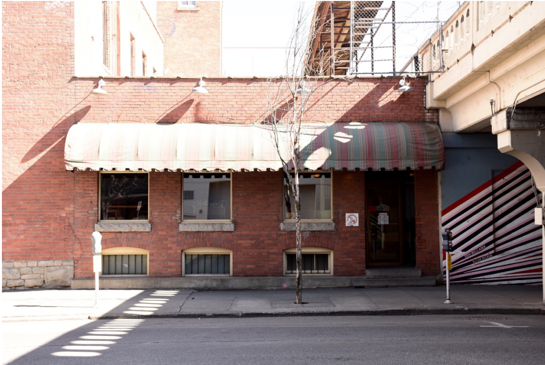
4. Cold storage building - front facade, looking east
