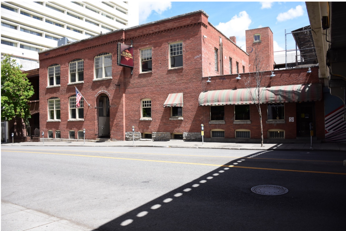
5. Front facade of warehouse building, looking east
