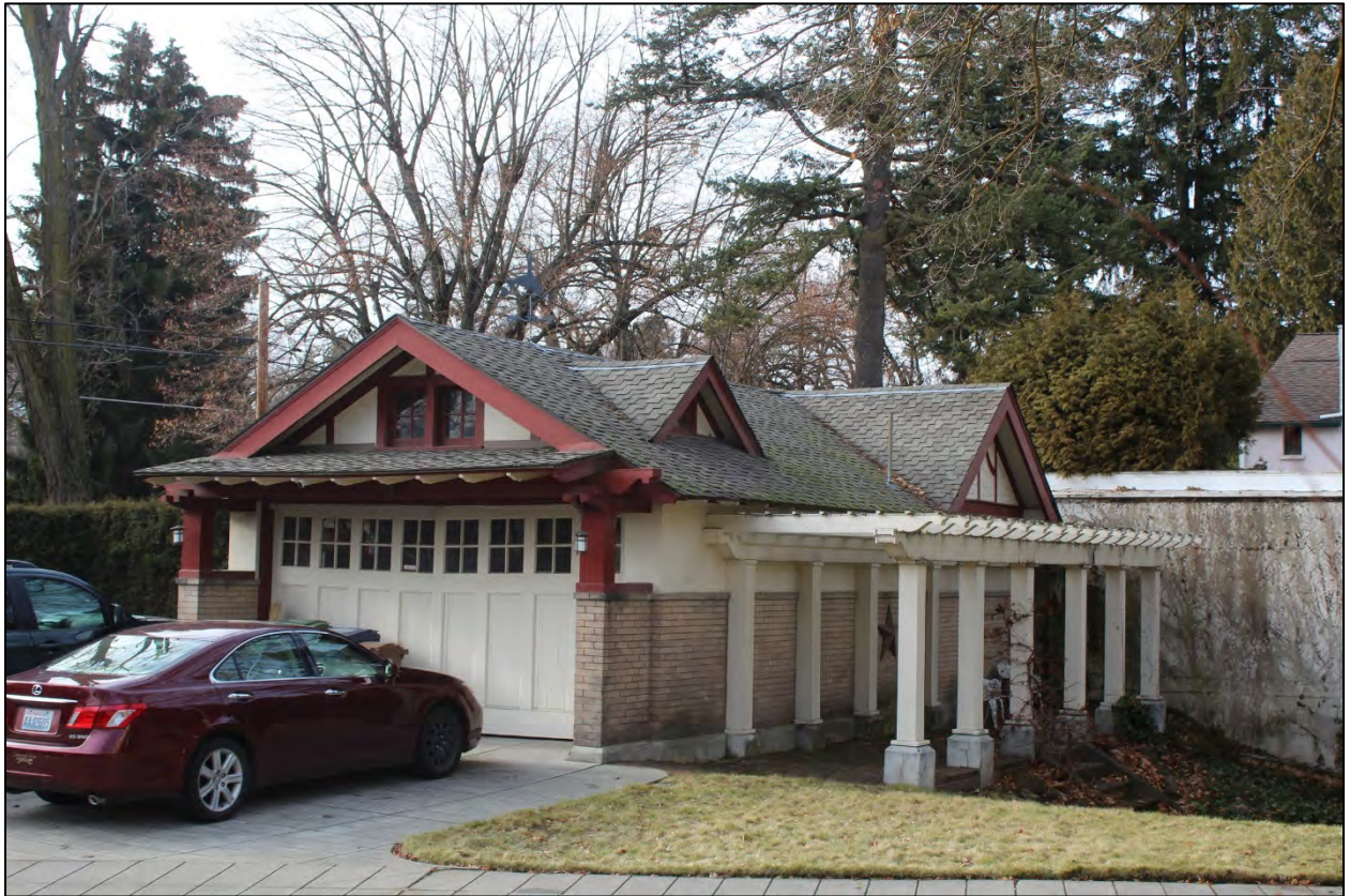
Photo 9 of 21: Front (east) and north side facades of garage
