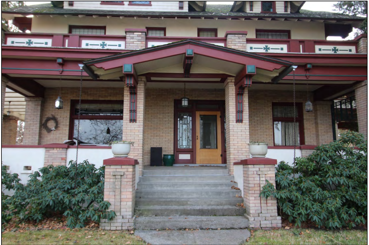
Photo 1 of 21: Front (north-northeast) façade, looking south
