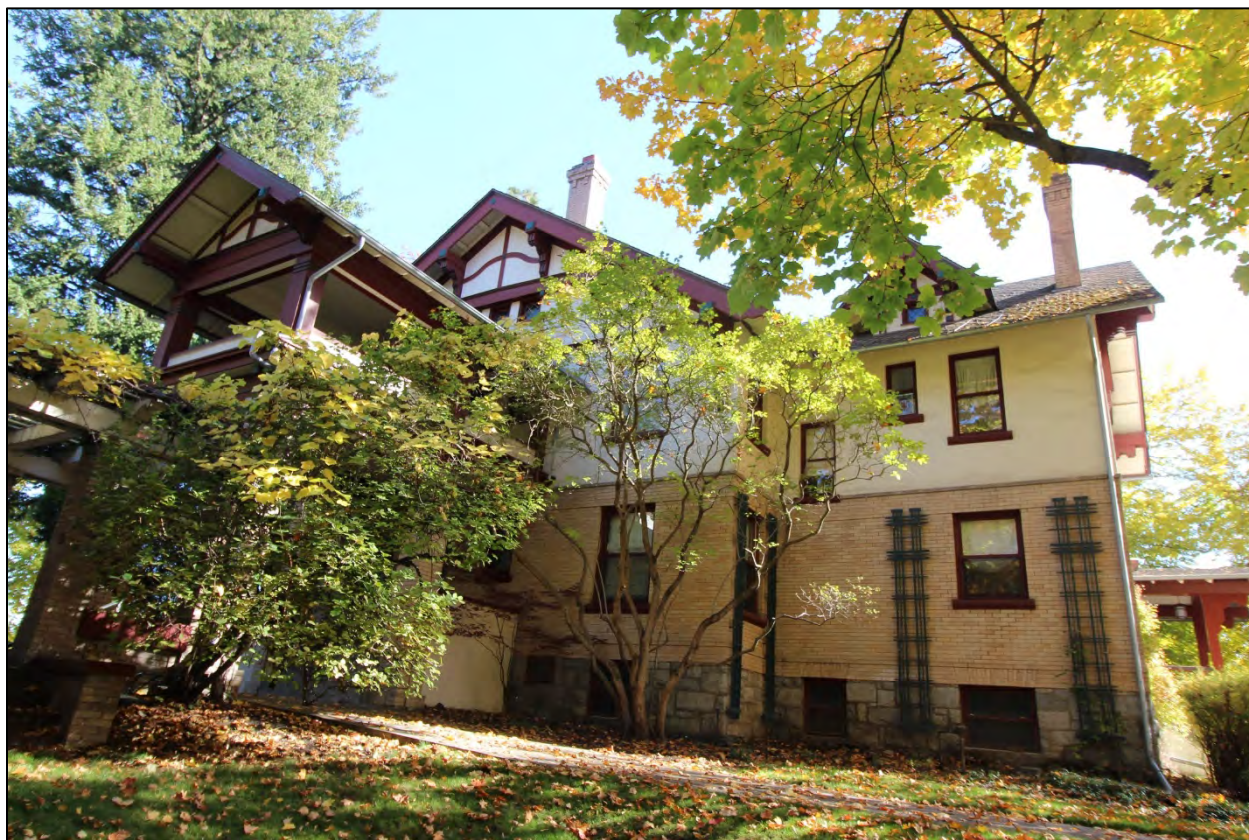
Photo 3 of 21: West side façade, looking east
