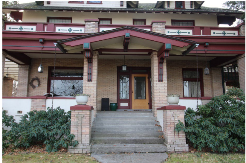
2 Front porch detail, north elevation
