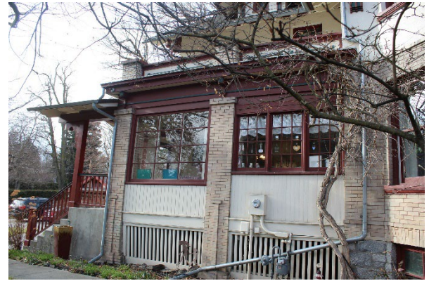
6 Enclosed sunroom - east elevation
