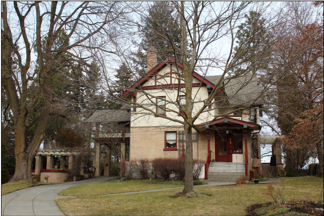
Photo 6 of 21: Rear (south) façade, looking north
