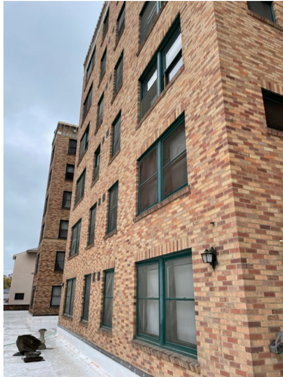
2| EXISTING WINDOW CONDITION
