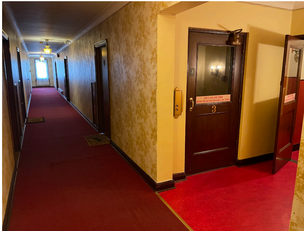
2| EXISTING TYPICAL STAIR + STAIR LOBBY
