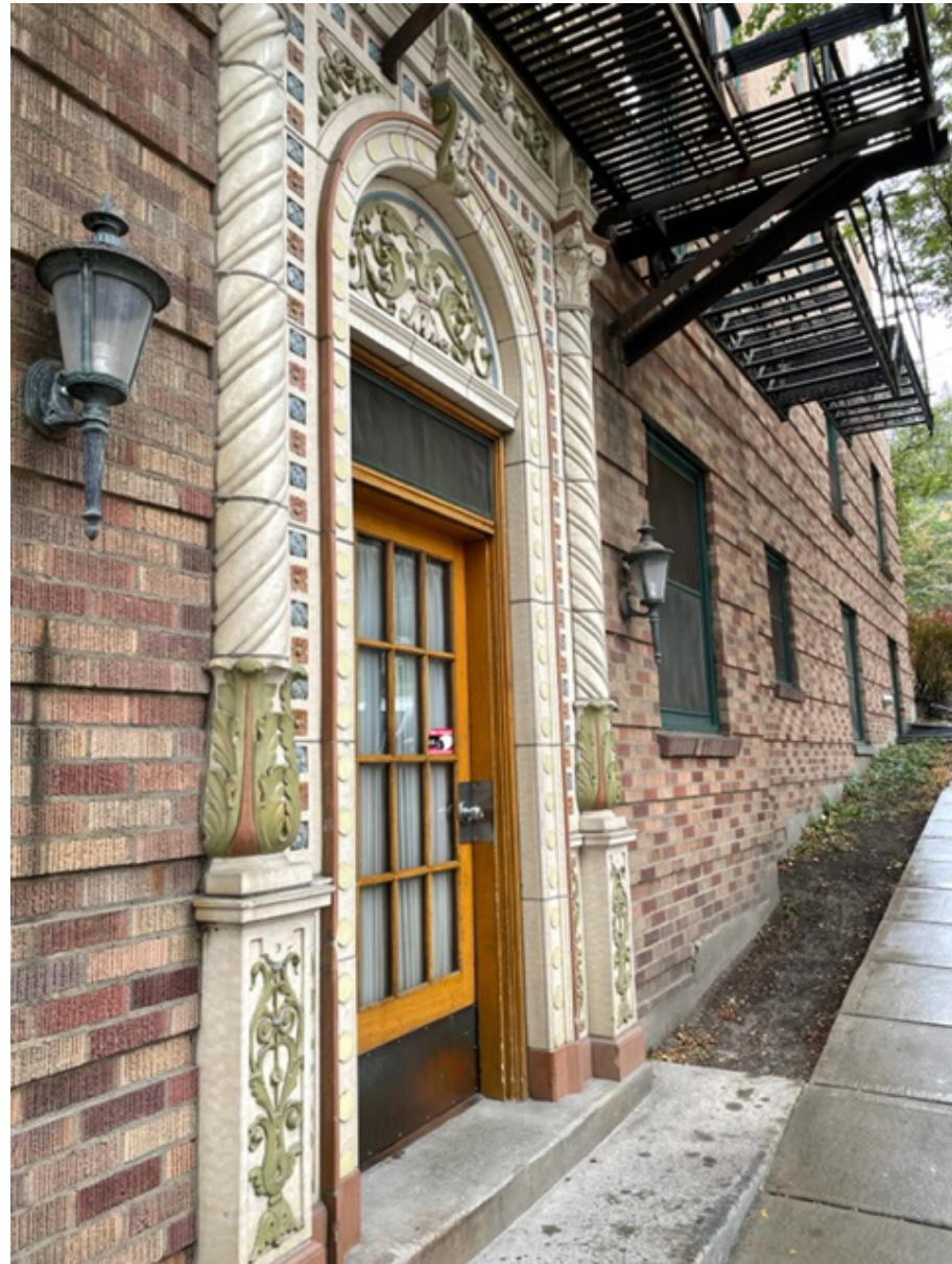
1| EXISTING DOOR CONDITION
