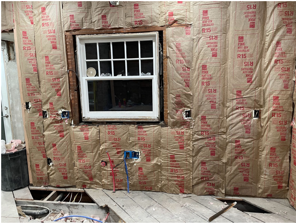
Figure 3: Kitchen of Adams House in 2023, facing south, DURING remodel. Replacement 10/1 single-hung window and new insulation visible.
