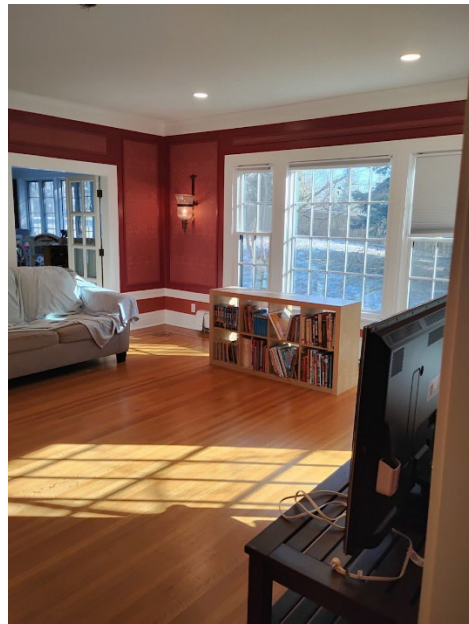
Family Room Trim – Repaired & Repainted
