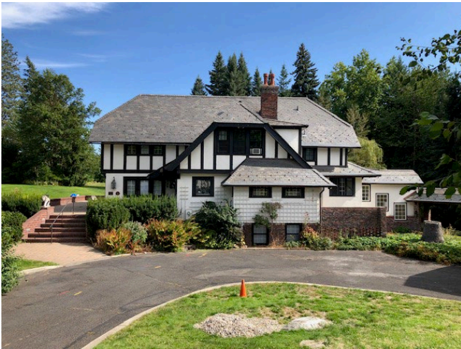
House Exterior /Drainage Before
