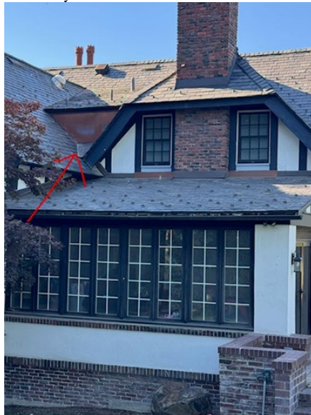
Roof Repair – Flashing: around Chimney; Below Primary-Bath Windows; East BD Bath
