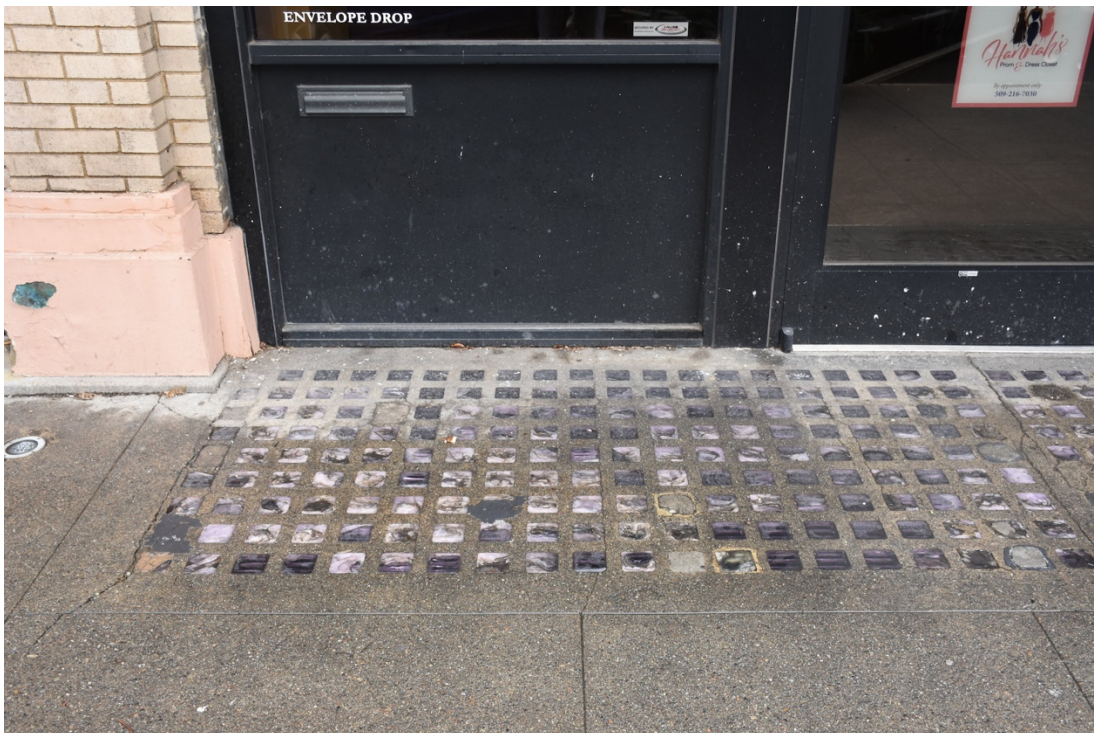
18. Sidewalk Vault Lights, looking east toward north bay entrance
