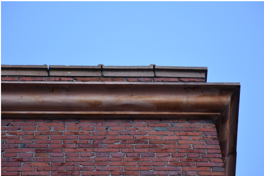
16. South Façade, east corner-showing cornice course and terra cotta coping, looking north
