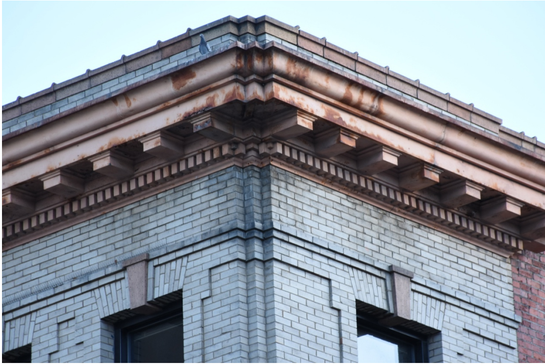
13. Southwest Corner - cornice and parapet coping
