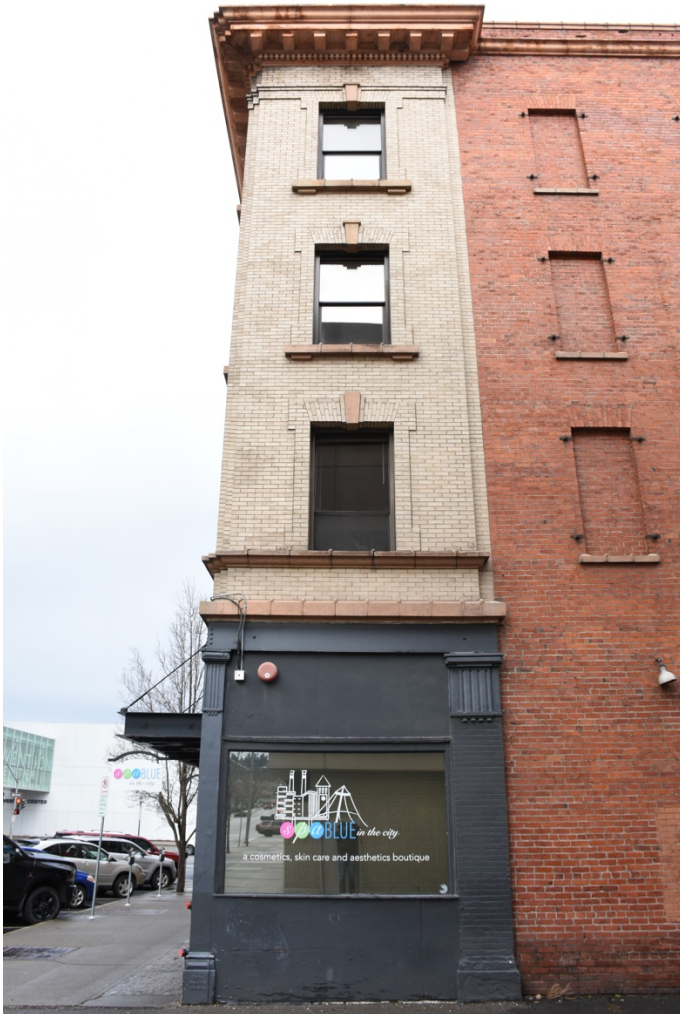
9. South Façade - Southwest corner detail showing cornice return and windows, looking north
