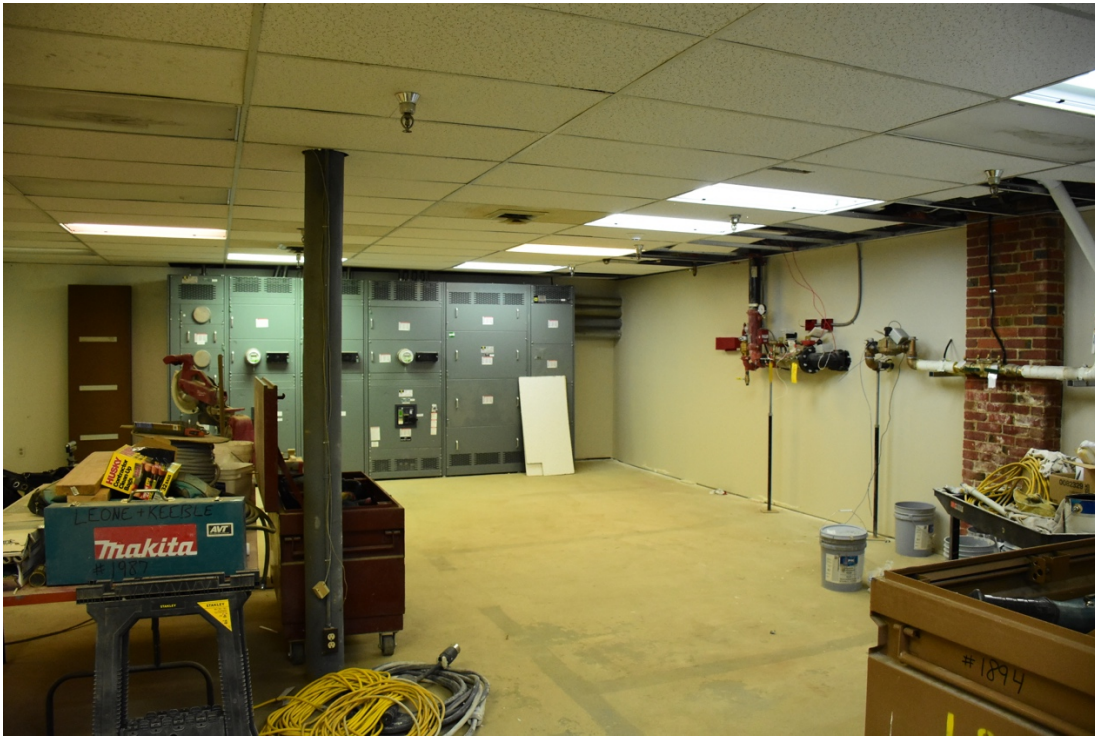
80. Basement, looking southwest at rebuilt west wall (sidewalk vault filled in) and electrical
