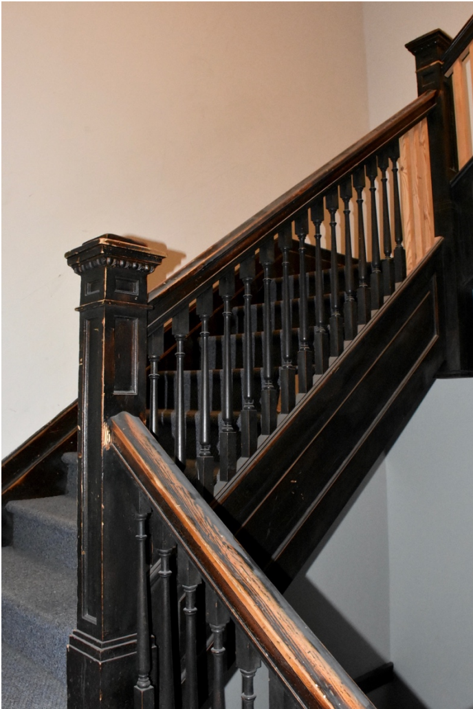
47. Historic Stairs to third floor, spindles replaced
