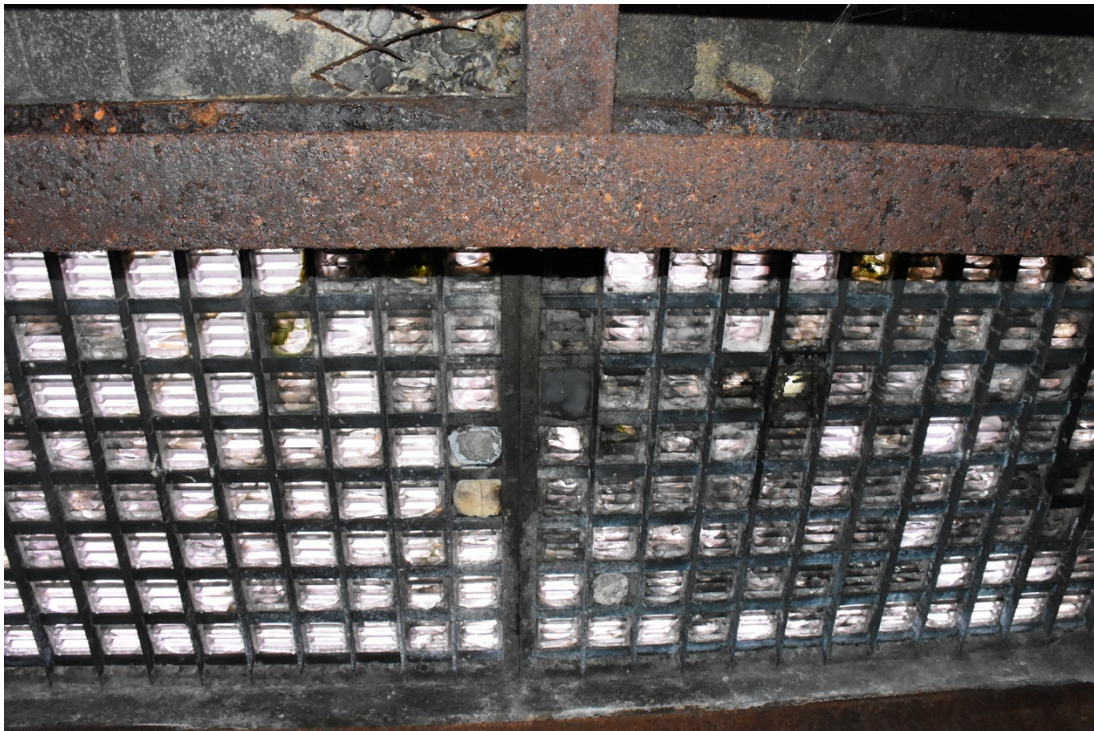
44. Basement Sidewalk Vault, looking east at vault lights
