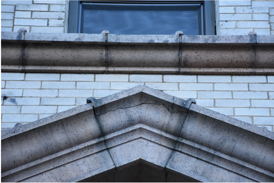
17. Front Façade - SRO hotel entrance pediment showing crack
