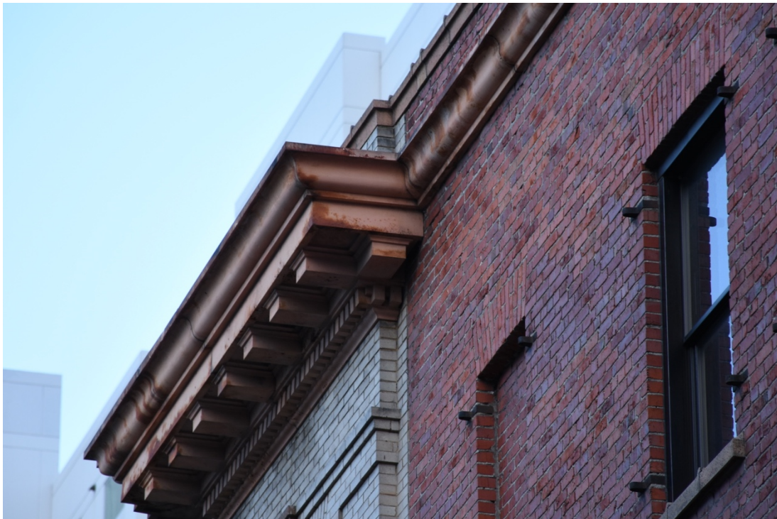
14. Southwest Corner - cornice return, parapet coping
