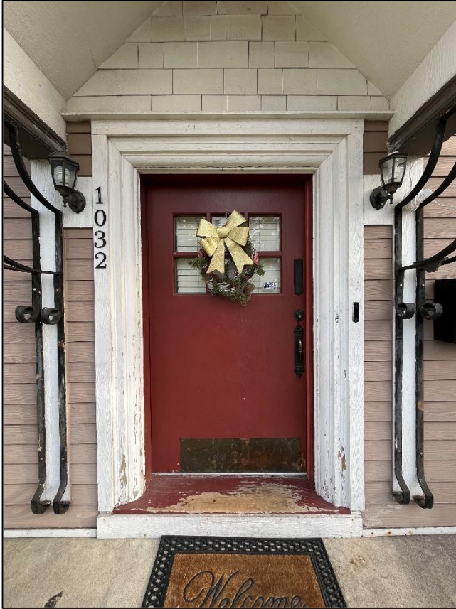
Cook-Abele House front door, 12/15/2023. Photo taken by Logan Camporeale SHPO.
