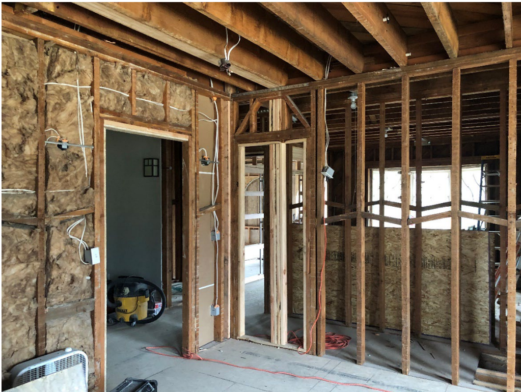
CONSTRUCTION: 2 nd Floor - Bedroom 4
