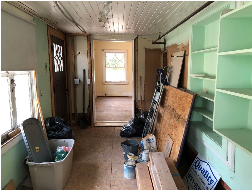
BEFORE: 2 nd Floor – Upstairs Kitchen
