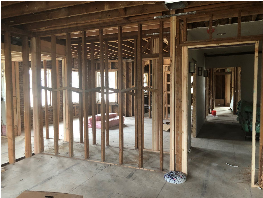
CONSTRUCTION: 2 nd Floor - Bedroom 3
