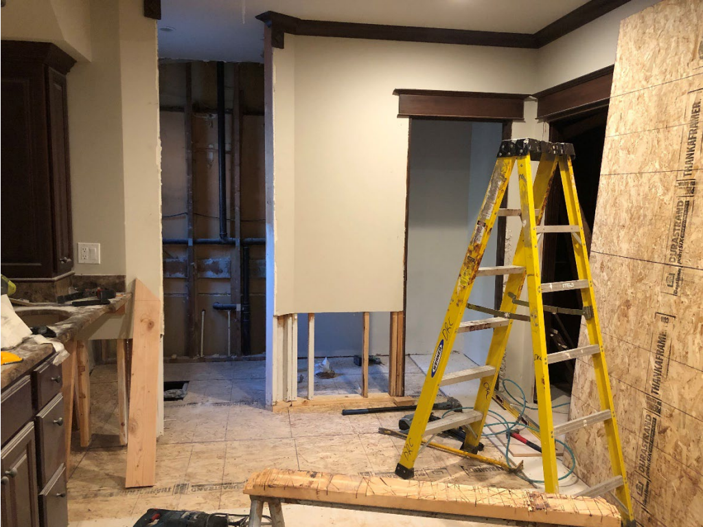
CONSTRUCTION: 1 st Floor – Master Suite
