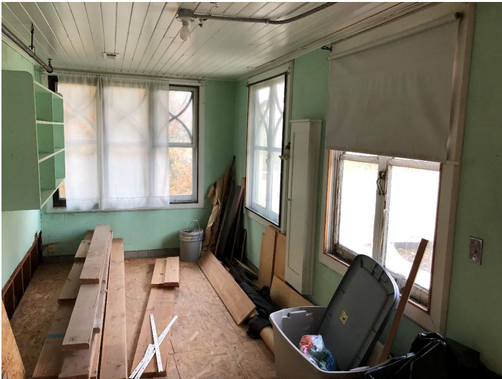
BEFORE: 2 nd Floor – Upstairs Kitchen
