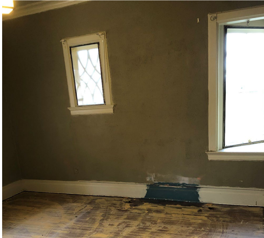
BEFORE: 2 nd Floor - Bedroom 1
