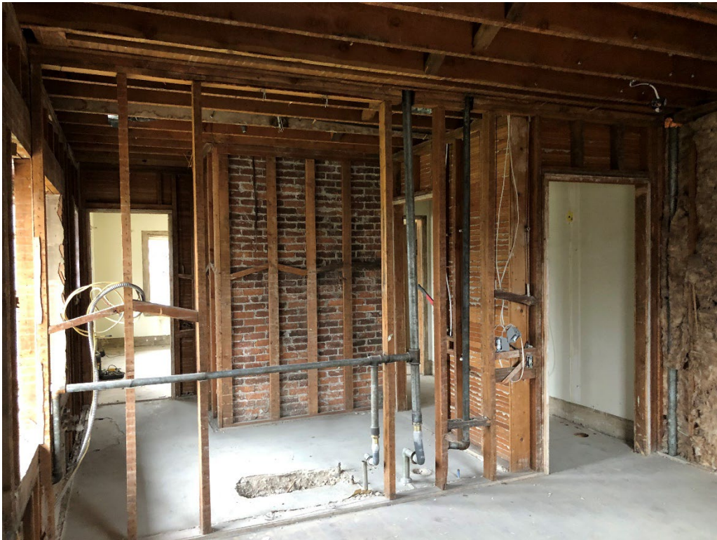
CONSTRUCTION: 2 nd Floor - Bedroom 1
