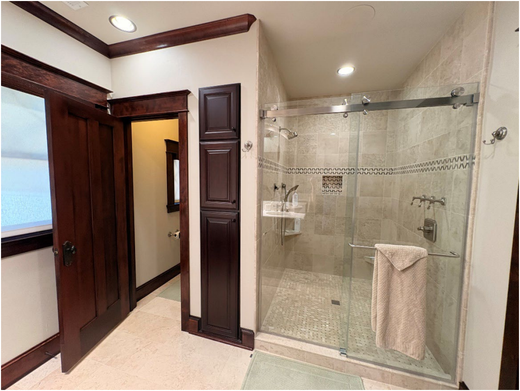
AFTER: 2 nd Floor - Bathroom 2
