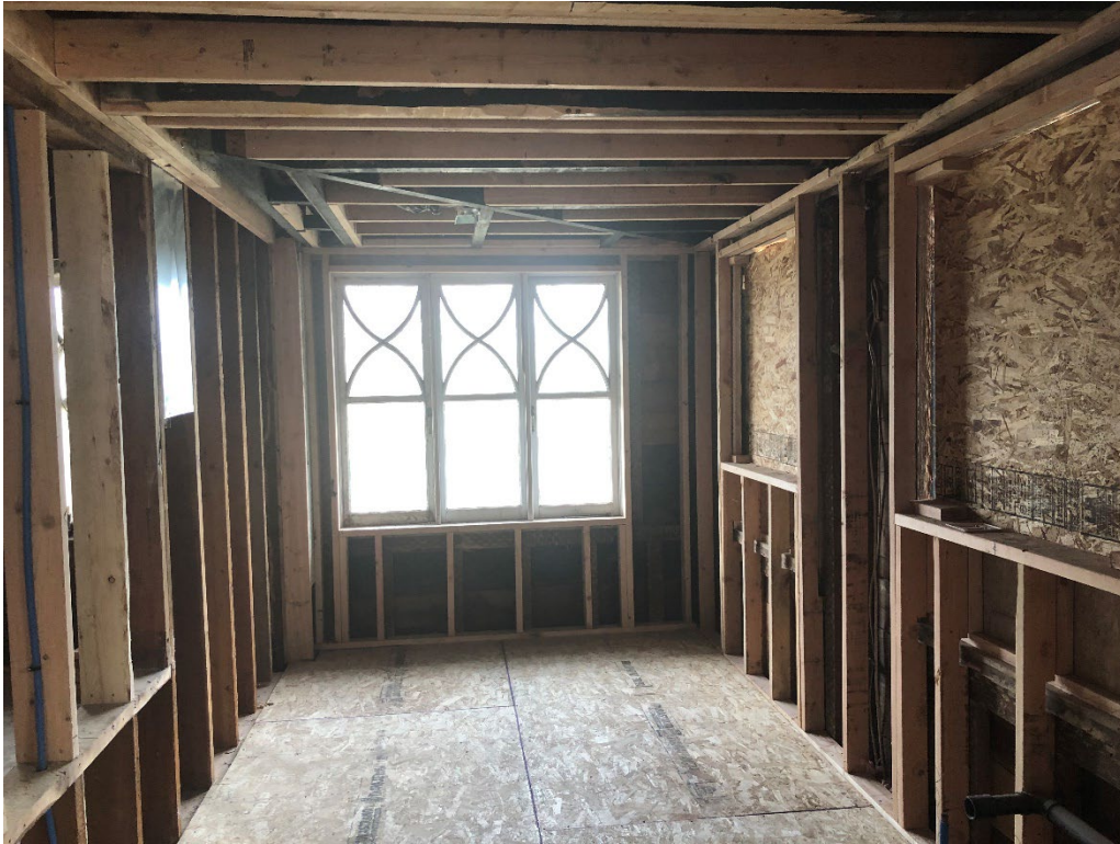
CONSTRUCTION: 2 nd Floor – Upstairs Kitchen
