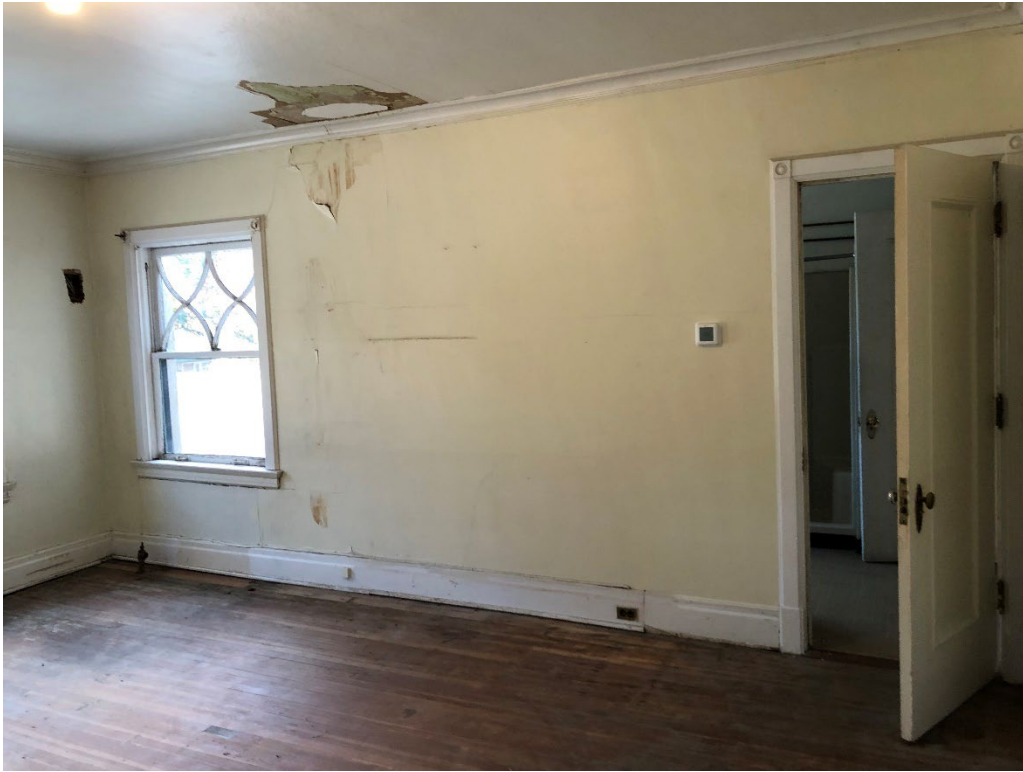
BEFORE: 2 nd Floor - Bedroom 4
