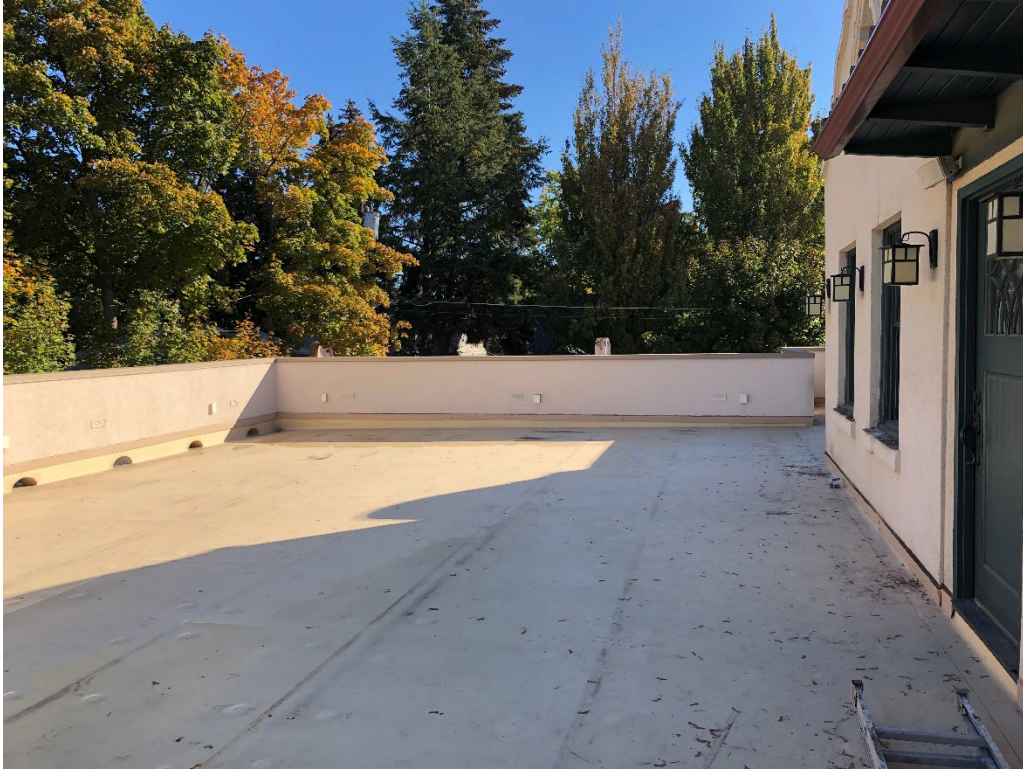
BEFORE: 2 nd Floor Deck
