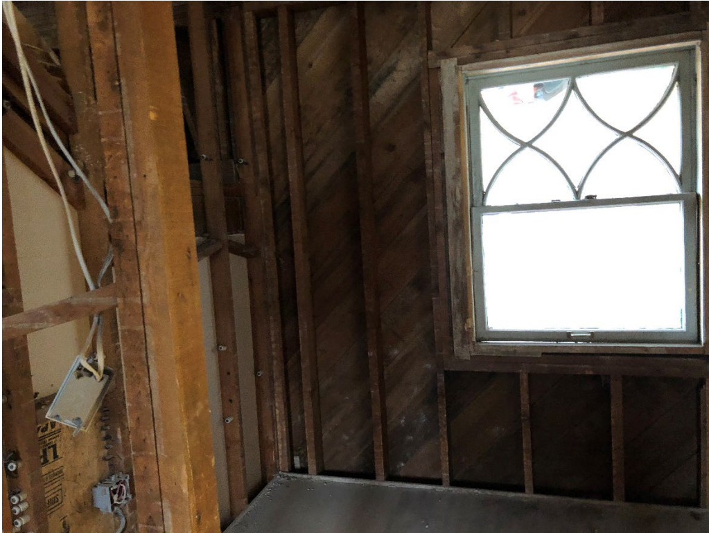
CONSTRUCTION: 2 nd Floor - Laundry Room
