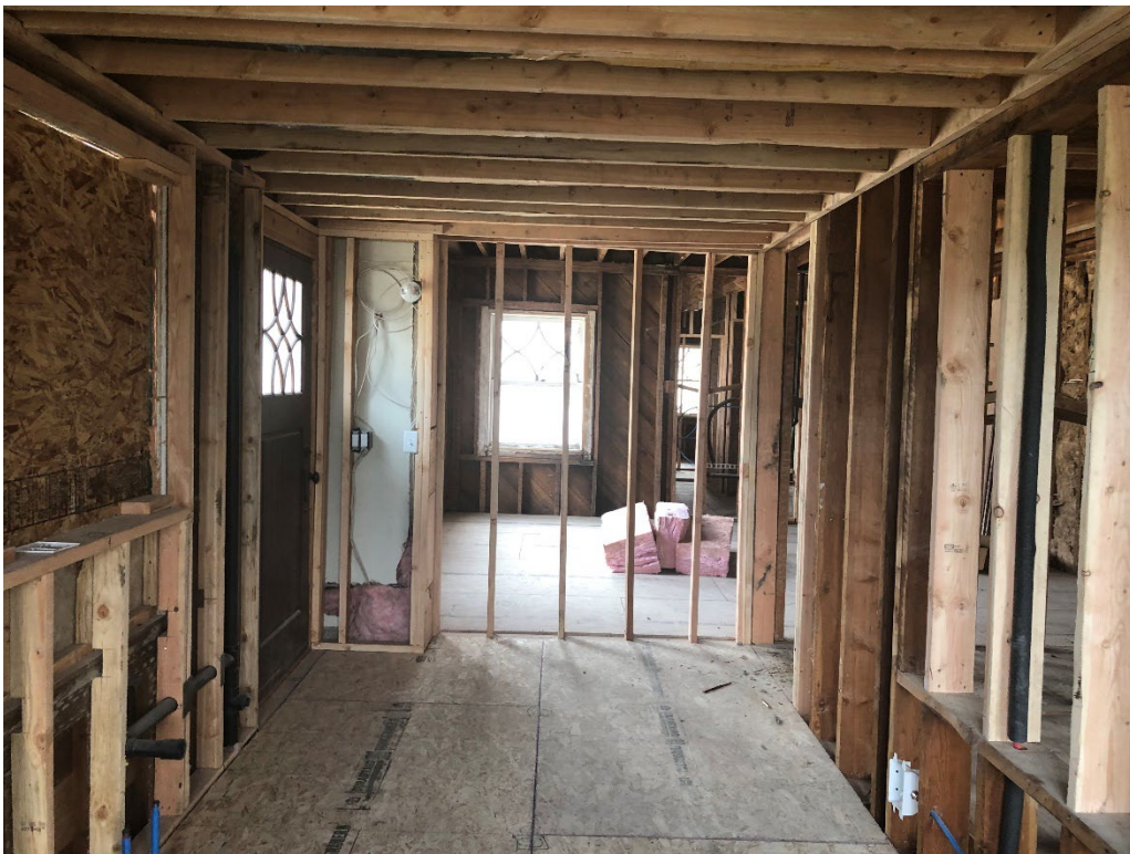
CONSTRUCTION: 2 nd Floor – Upstairs Kitchen
