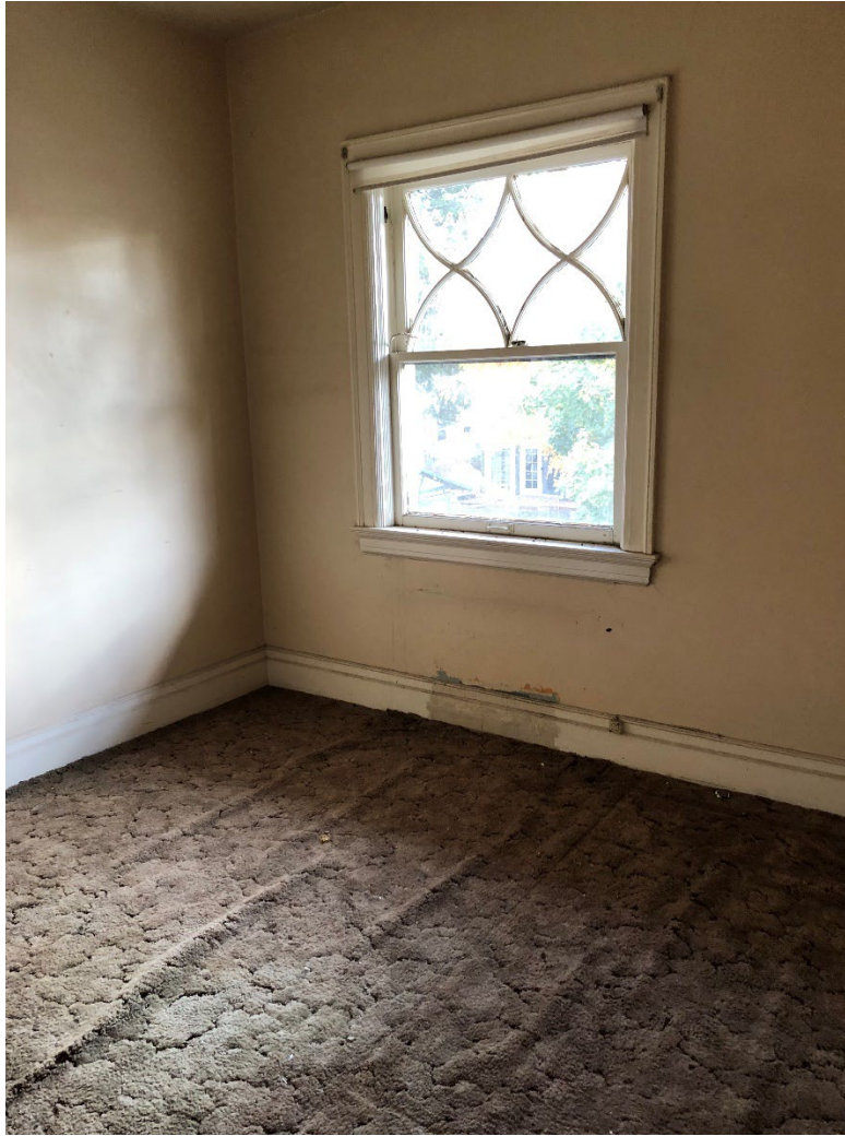
BEFORE: 2 nd Floor – Upstairs Closet
