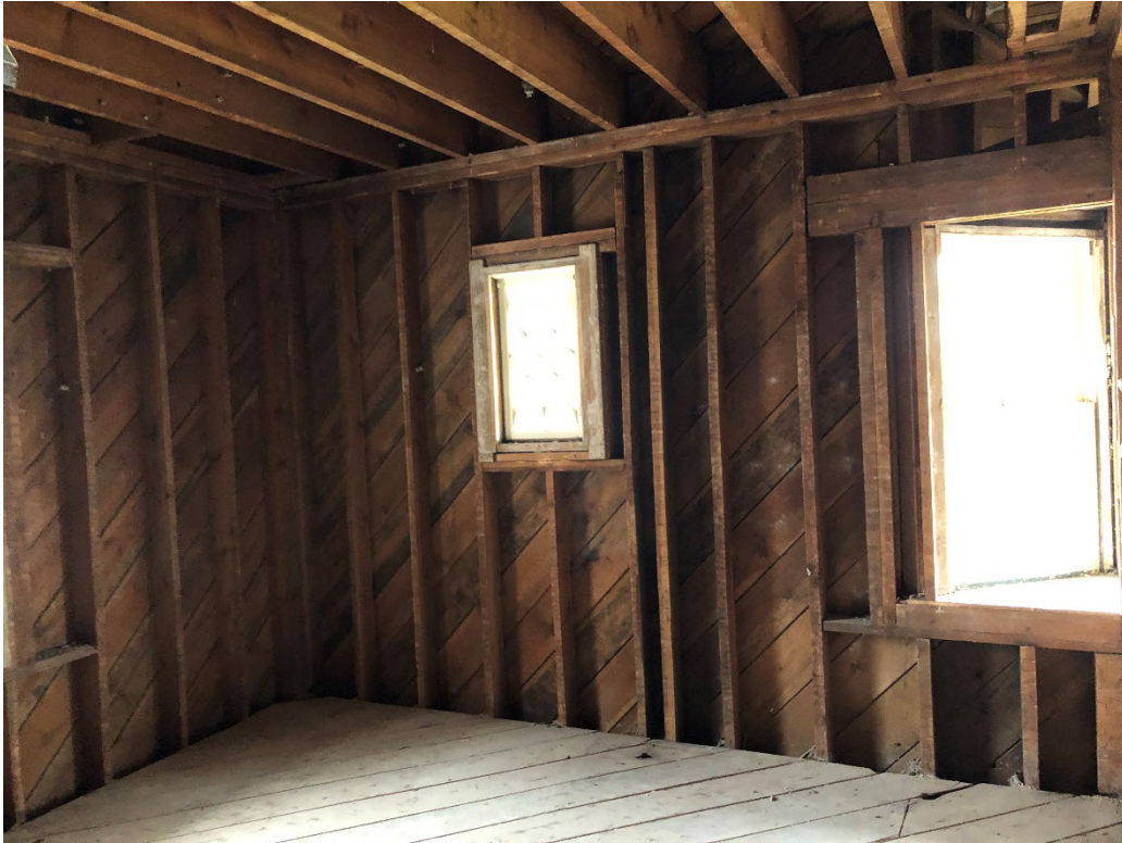
CONSTRUCTION: 2 nd Floor - Bedroom 1
