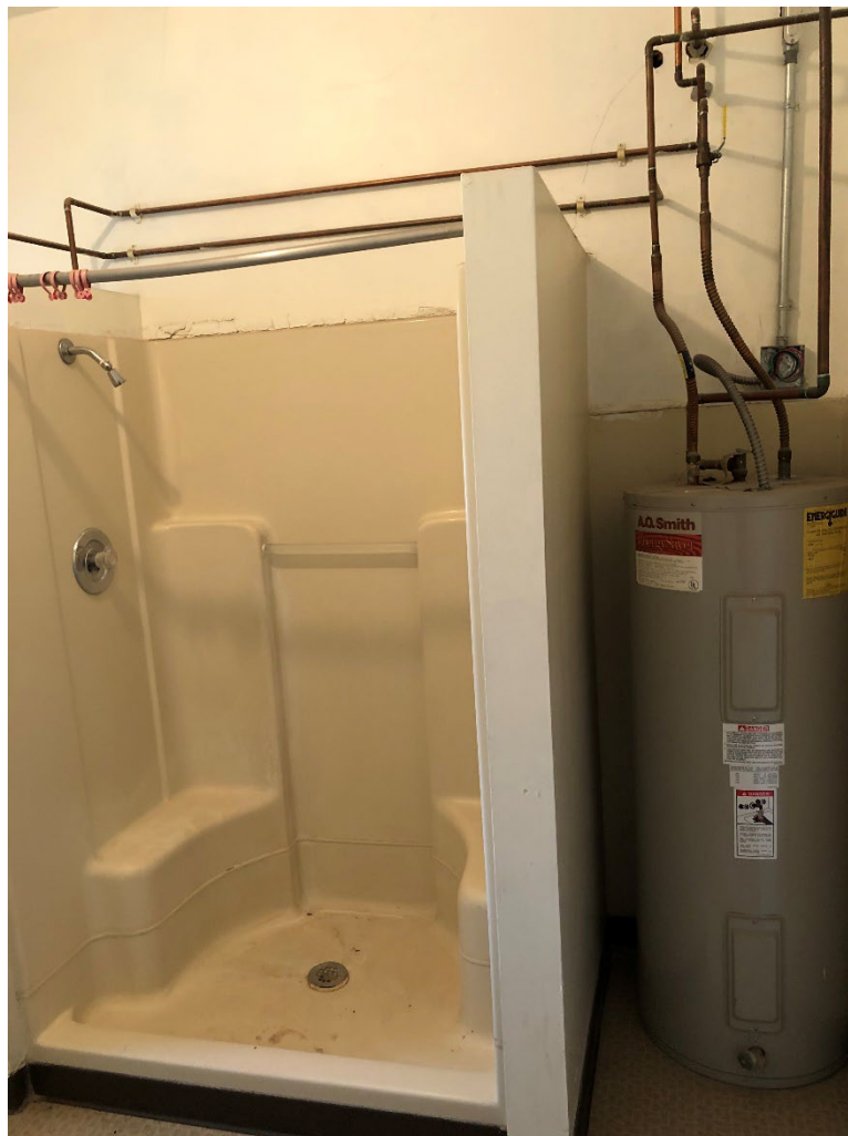
BEFORE: 2 nd Floor - Bathroom 2
