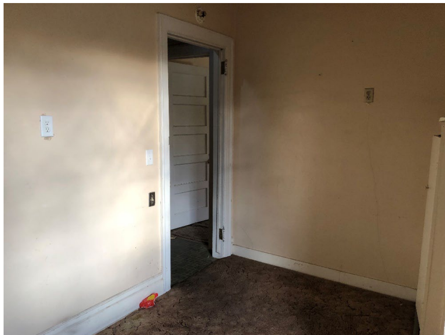
BEFORE: 2 nd Floor – Upstairs Closet
