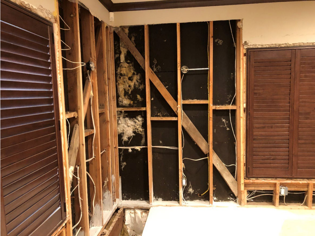
CONSTRUCTION: 1 st Floor – Master Suite
