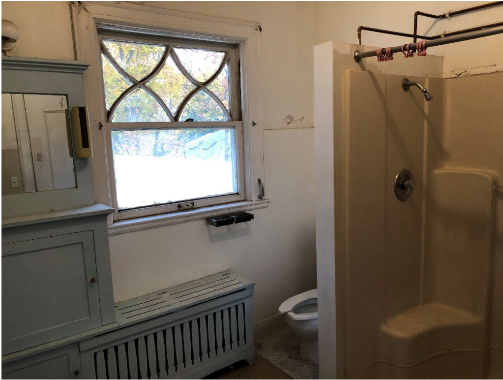
BEFORE: 2 nd Floor - Bathroom 2
