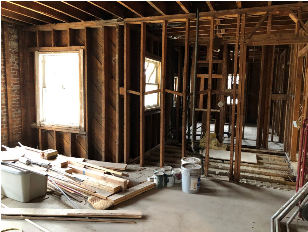
CONSTRUCTION: 2 nd Floor - Bedroom 4
