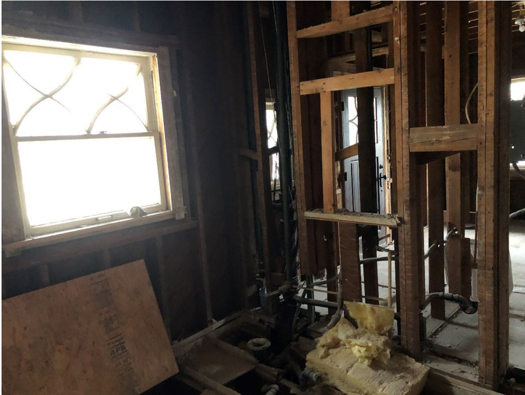
CONSTRUCTION: 2 nd Floor - Bathroom 2
