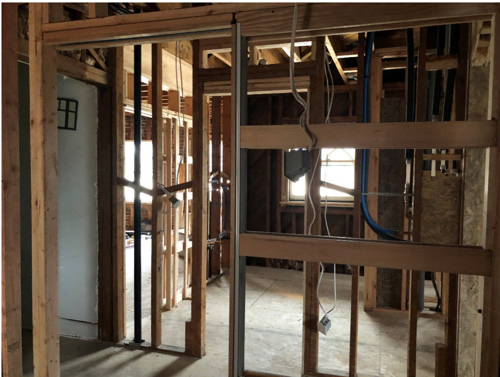
CONSTRUCTION: 2 nd Floor - Laundry Room
