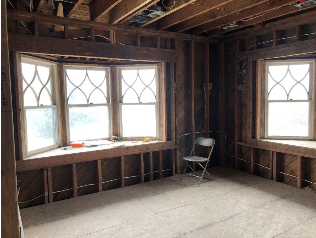
CONSTRUCTION: 2 nd Floor Bedroom 2
