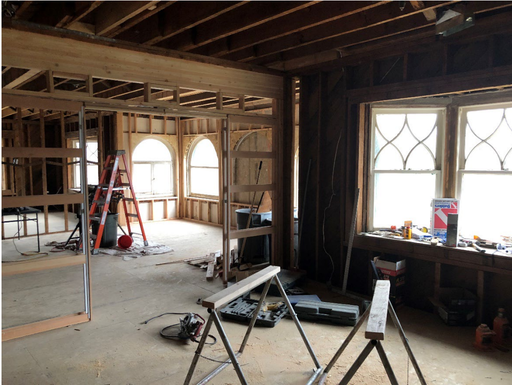
CONSTRUCTION: 2 nd Floor - Bedroom 3
