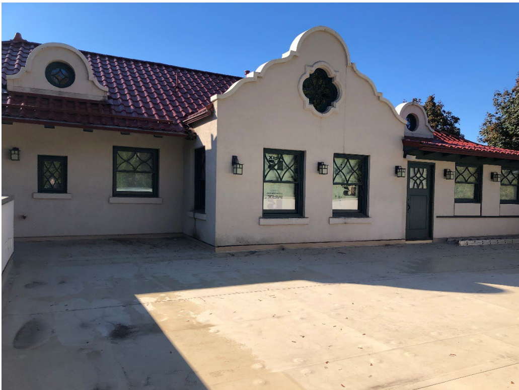
BEFORE: 2 nd Floor Deck
