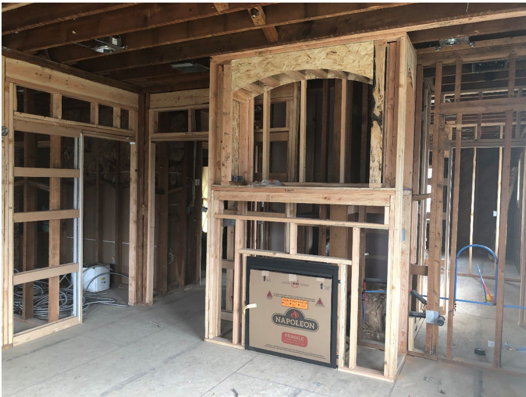
CONSTRUCTION: 2 nd Floor Bedroom 2
