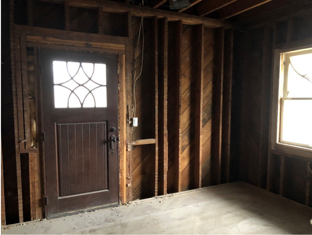
CONSTRUCTION: 2 nd Floor - Upstairs Closet
