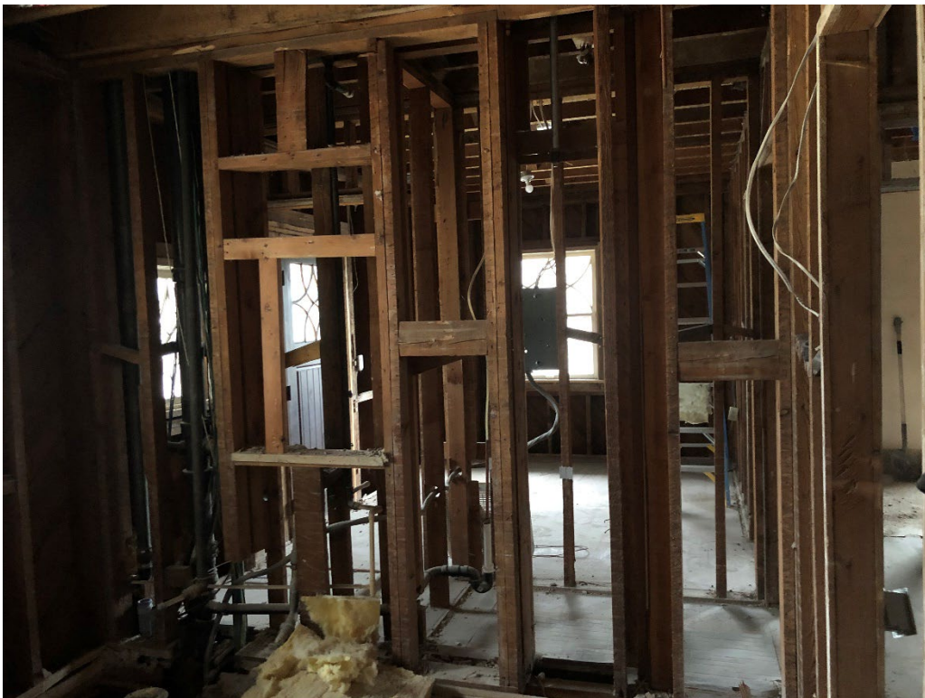
CONSTRUCTION: 2 nd Floor - Bathroom 2
