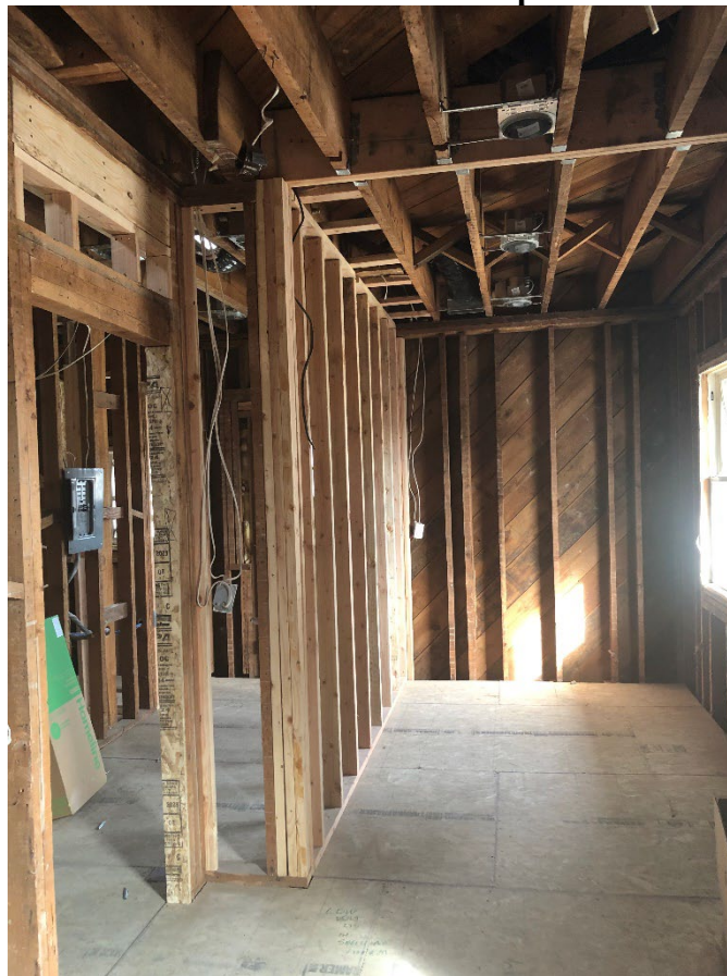
CONSTRUCTION: 2 nd Floor - Upstairs Closet
