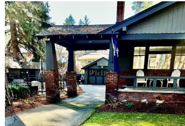
Figure 12: A roofed section of the driveway – a porte cochere – completes the entrance components of this bungalow. Stairs to the porch rise from the driveway as well as the front walk. Shoshone Place
