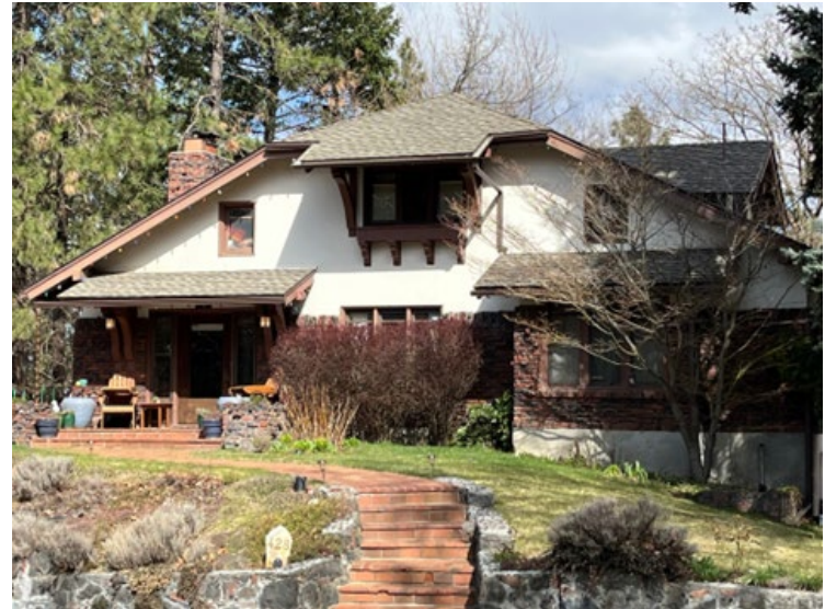
Figure 4: This bungalow has rough-textured clinker brick on the first story and stucco walls on the second.
