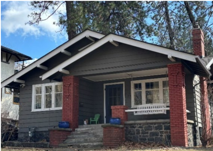
Figure 5: This bungalow is clad with cedar shingles above a cut-stone foundation. 457 Shoshone Place
