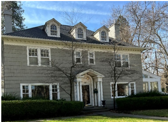
Figure 14: The historic windows with grouped windows separated by mullions and small panes defined by narrow muntins further the Colonial-Revival style of this residence. Dormers have arched window heads and curved muntins. Shoshone Place
