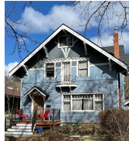
Figure 2: This residence displays three exterior materials above a stone foundation: lapped siding on the first story, board-and-batten siding on the second story, and half timbering at the attic level. 634 W 21st Avenue
