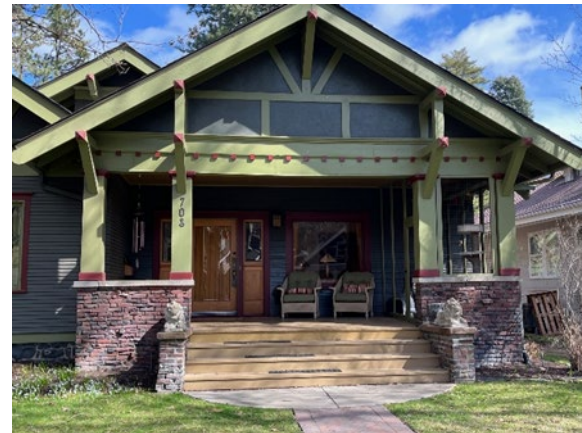
Figure 8: This bungalow porch has brick knee walls framing steps and serving as closed balustrade walls. Square wood posts support a lintel with a decorative dentil course. Brackets support the overhanging eaves of the porch roof. The wide door flanked by narrow windows is the entrance.
