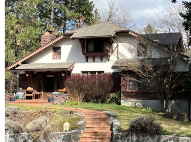
Figure 5: This bungalow has rough-textured clinker brick on the first story and stucco walls on the second.
