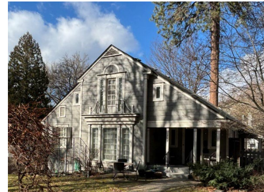
Figure 17: The fenestration of this façade features grouped windows with an elaborate surround below a view balcony with a door flanked with sidelights. W 21st Ave
