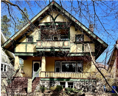
Figure 13: "View balconies" at the second-story levels of English/Craftsman residences and bungalows are another type of porch-like element in the district. Usually shallow, and perhaps recessed as this one is, these features had a balustrade and were accessed by doors from the interior. W 20 th Avenue
