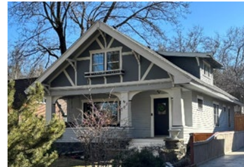
Figure 3: This bungalow displays half-timbering on the gable face and cedar-shingles on the dormer walls. 703 W 20th Avenue
