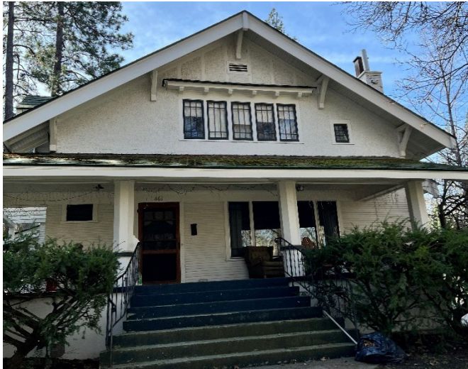
Figure 9: This full-façade porch has full-height octagonal columns supporting its shed roof. Brackets at the eaves and a shallow shed-roof to deflect rain from the upper level windows with original sash.
