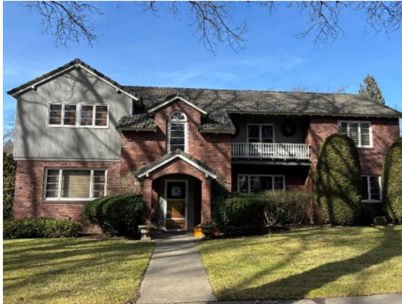
Figure 16: Window sash in this 1949 residence includes a picture window flanked by casement sash with horizontal muntins, sash that appears in a bank of four windows above. Oneida Place
