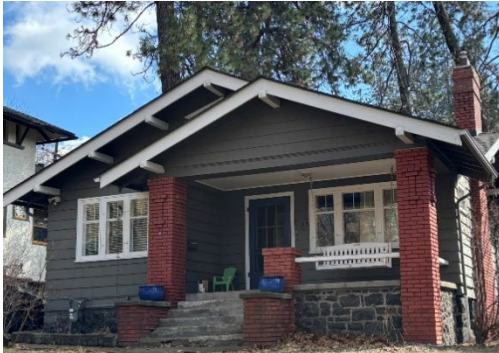
Figure 4: This bungalow is clad with cedar shingles above a cut-stone foundation. 457 Shoshone Place
