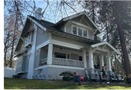
Figure 7: This English/Craftsman residence has several gabled roofs, including a roof dormer and porch steps roof, with angled brackets at the wide eaves. 2015 S. Oneida Place
