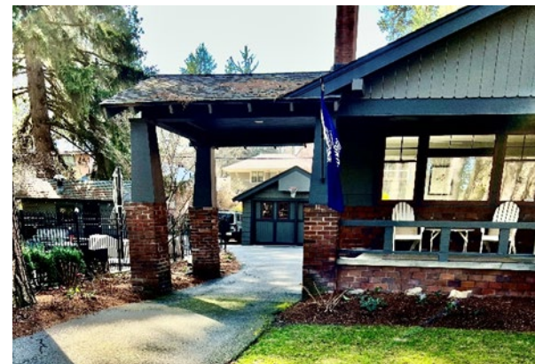
Figure 11: A roofed section of the driveway – a porte cochere – completes the entrance components of this bungalow. Stairs to the porch rise from the driveway as well as the front walk. Shoshone Place
