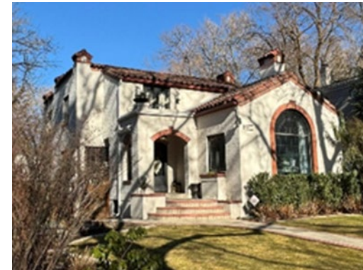
Figure 6: This Mission-Revival cottage with stucco walls has a complex gabled roofline clad with clay tile. 606 W 20th Avenue
