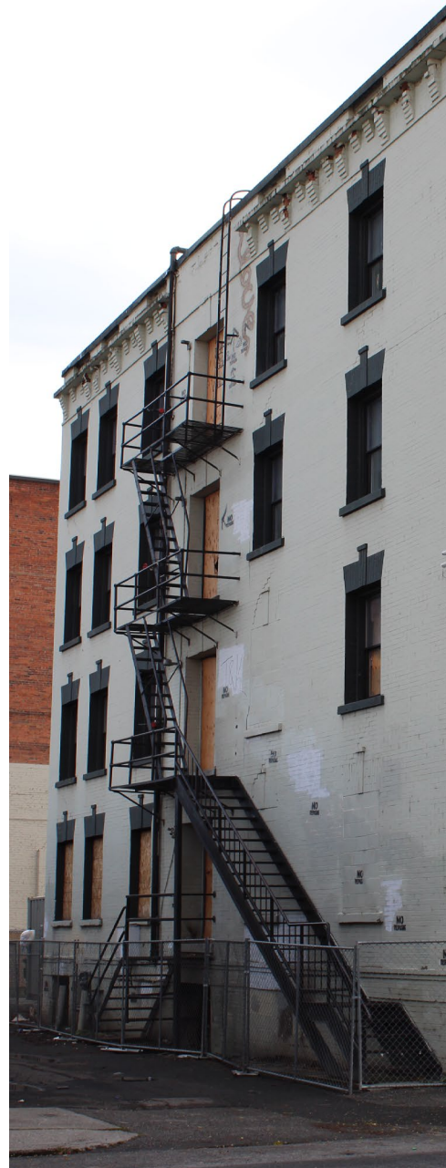
View of north elevation looking southeast showing windows blocked in by stairs for fire escape.
