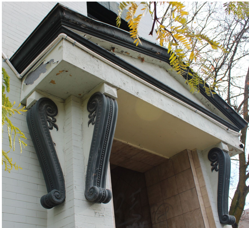
Detail of sheet metal consoles on the entrance.
