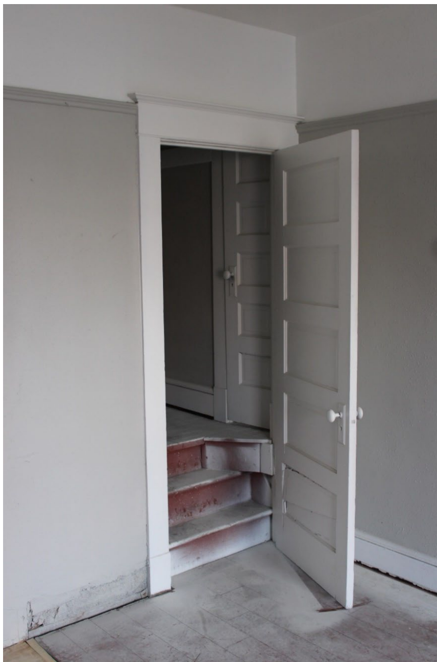
19. Detail of closet door in an apartment showing elevated floor and small door to bathroom.
