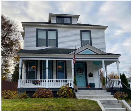
Primary Material Lap Siding
