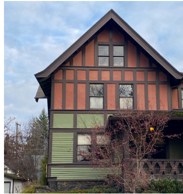
Secondary Material Smooth Fibercement Panel evokes stucco patterns of contributing buildings in the district
