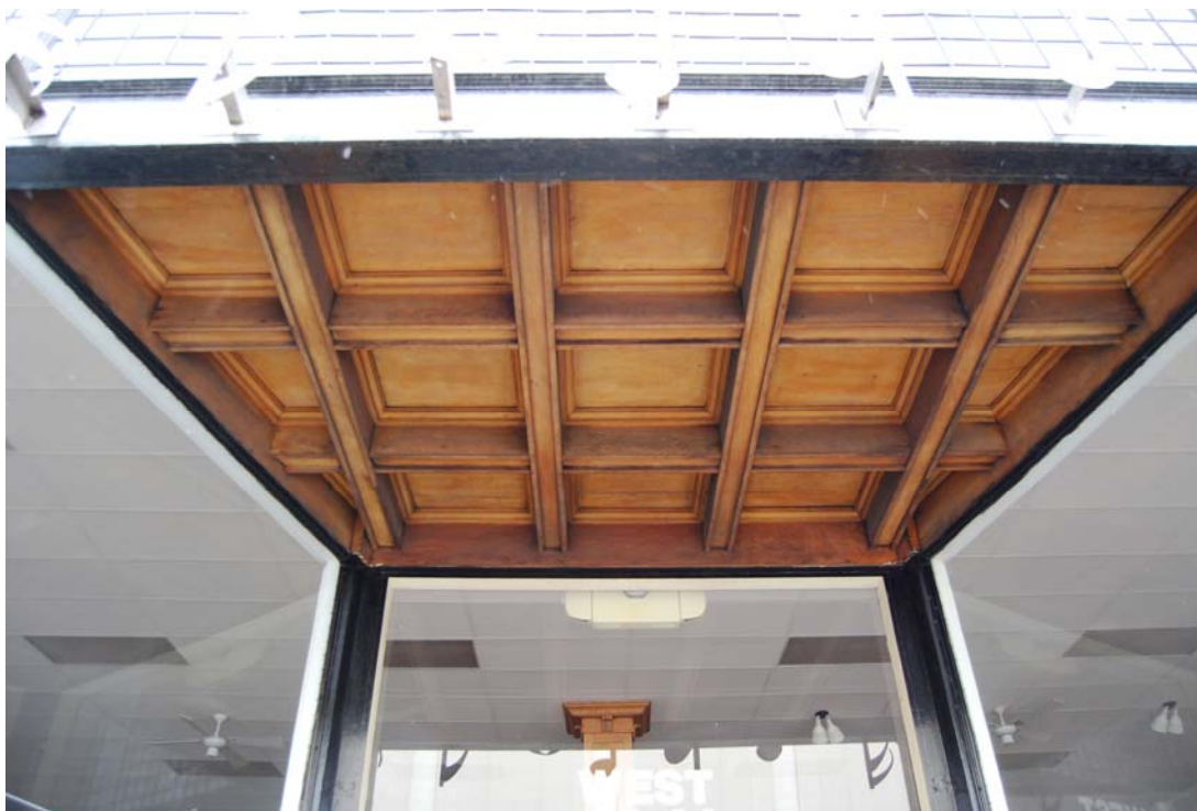
6. Coffered ceiling above main entry approach
