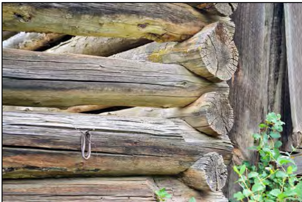
Figure 74. Barn, detail of corner notching at southwest corner of log section; view to the southeast.
