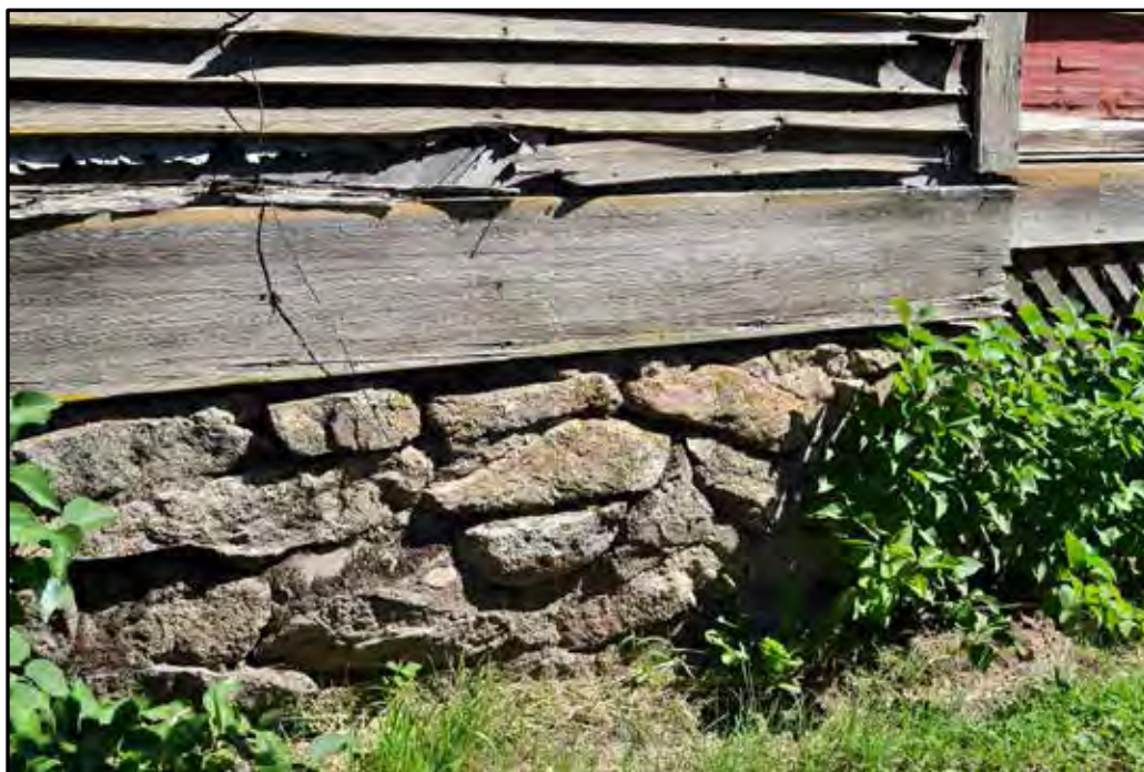
Figure 26. 1890s Farmhouse, detail of stone foundation on east section's south side; view to the northeast.
