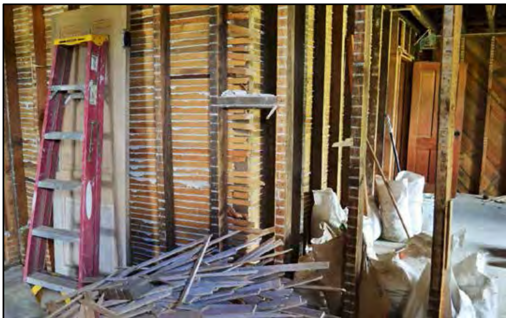
Figure 46. 1890s Farmhouse, second floor: Lath and plaster construction visible in probable bedroom (#9 on Figure 3), left, probable bedroom (#7), right; view to the southwest.
