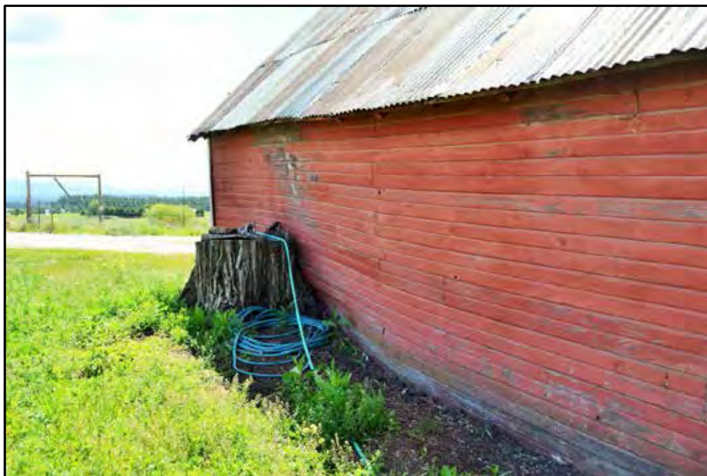
Figure 59. Garage, bowing of north wall due to growth of cottonwood tree; view to the southeast.
