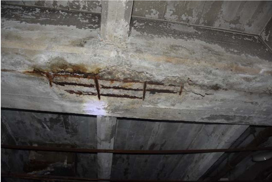
4. Basement ceiling showing spalling concrete and rusted rebar
