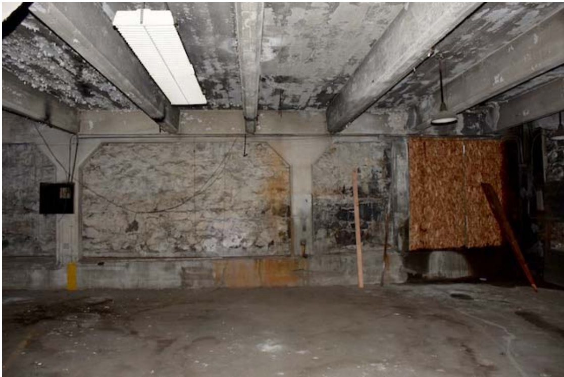
5. Basement garage, looking east - reinforced concrete post and beam, basalt rubble wall
