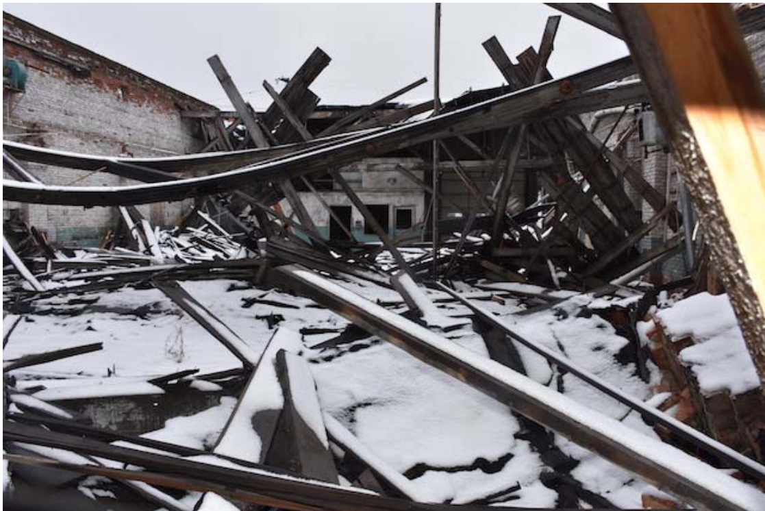
13. 1914 building - roof collapse, looking south from north wall
