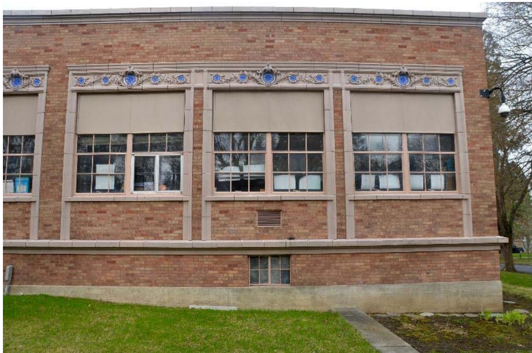
14. Detail of window bays on original east facade
