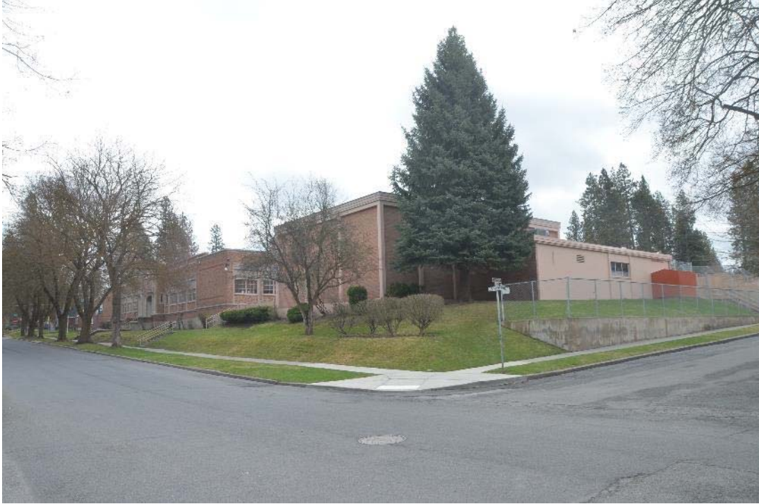
7. Northwest corner showing multi-purpose room, looking southeast
