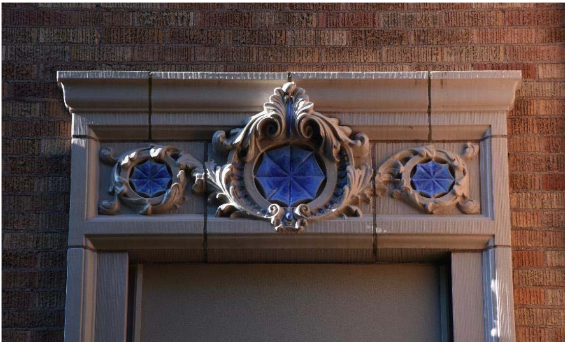
16. Window head detail front facade, looking south
