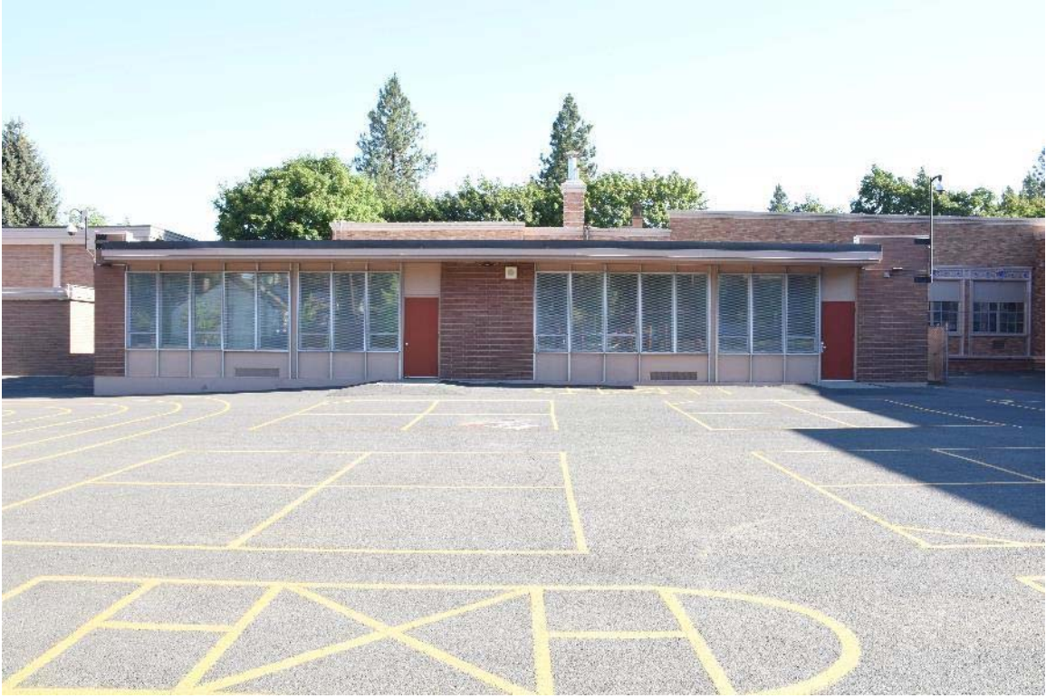
19. Looking north at south facade of 1961 addition
