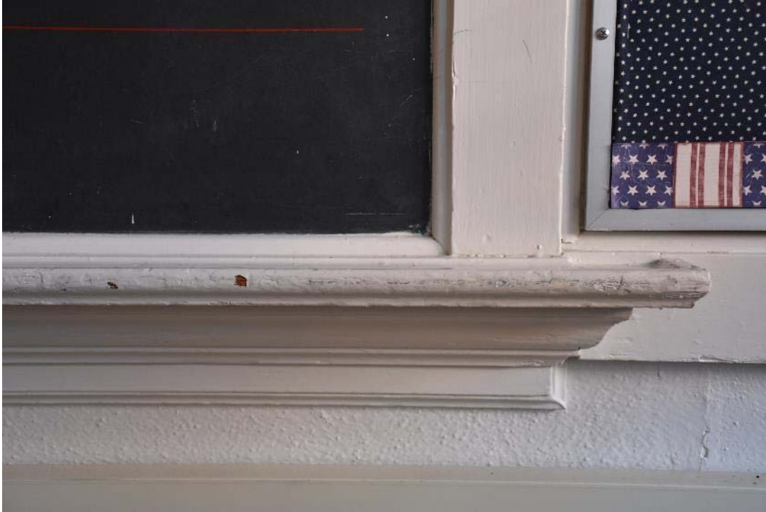
24. Detail - Original chalk rail in northwest corner classroom
