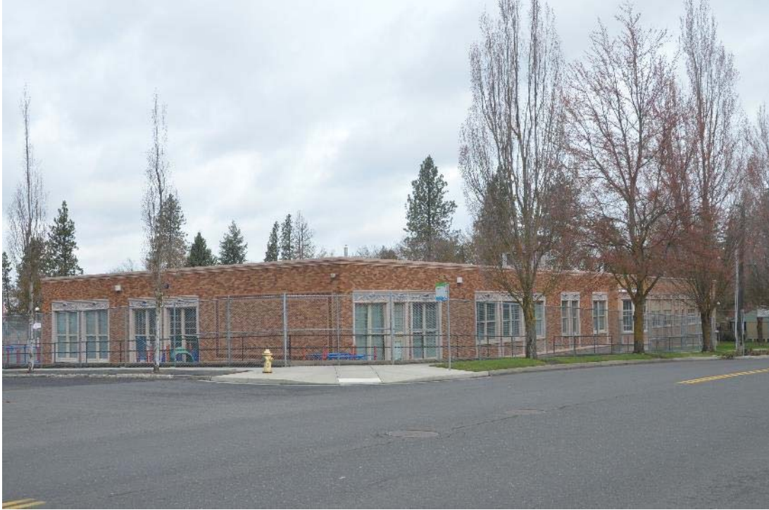
5. Southeast corner - east facade, looking northwest
