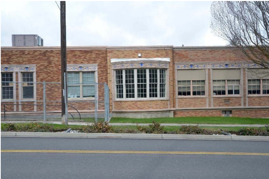
4. East facade - juncture of 1999 addition, 1941 addition, and original [153]-[154] looking west
