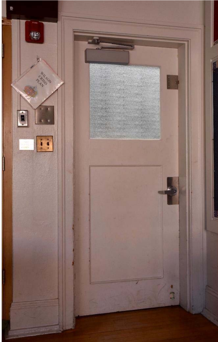
23. Detail - 161 Original door and moldings in northwest corner classroom
