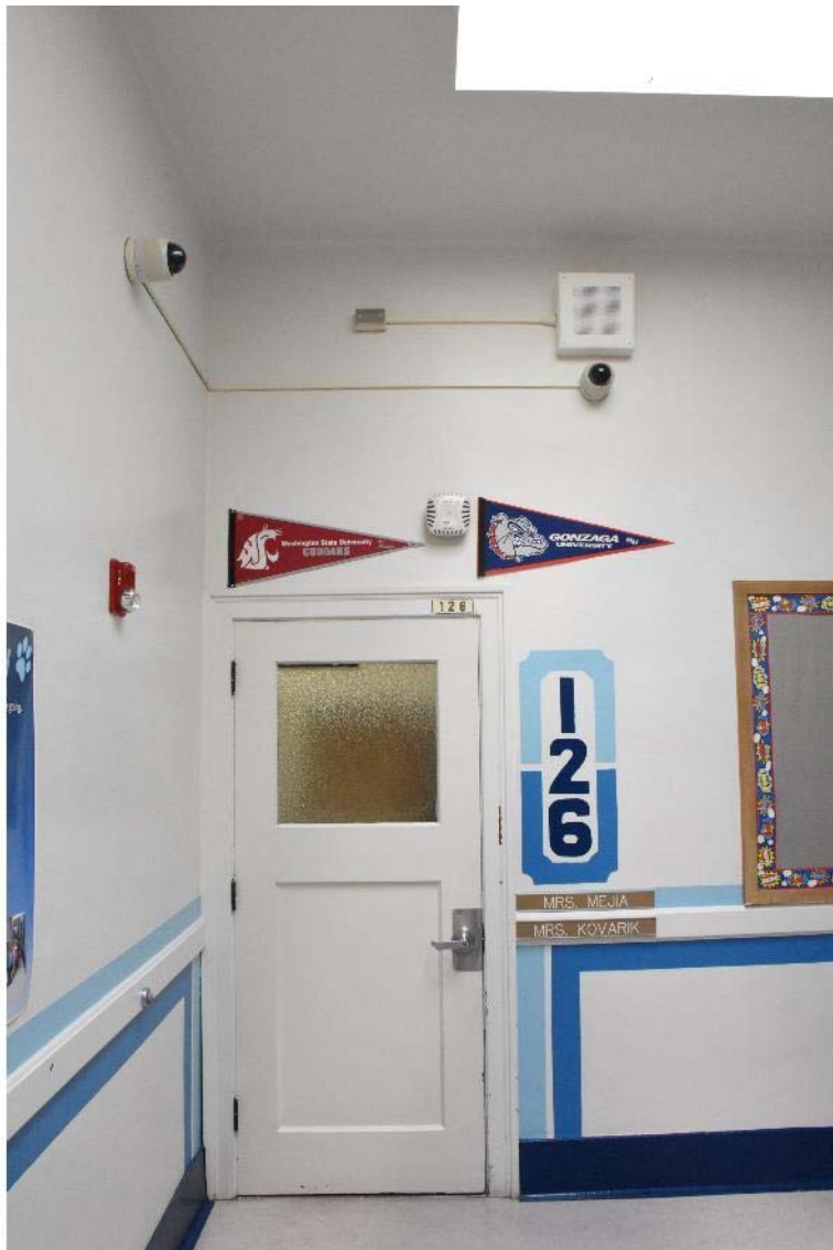
6. Door to original classroom 126 in northeast corner
