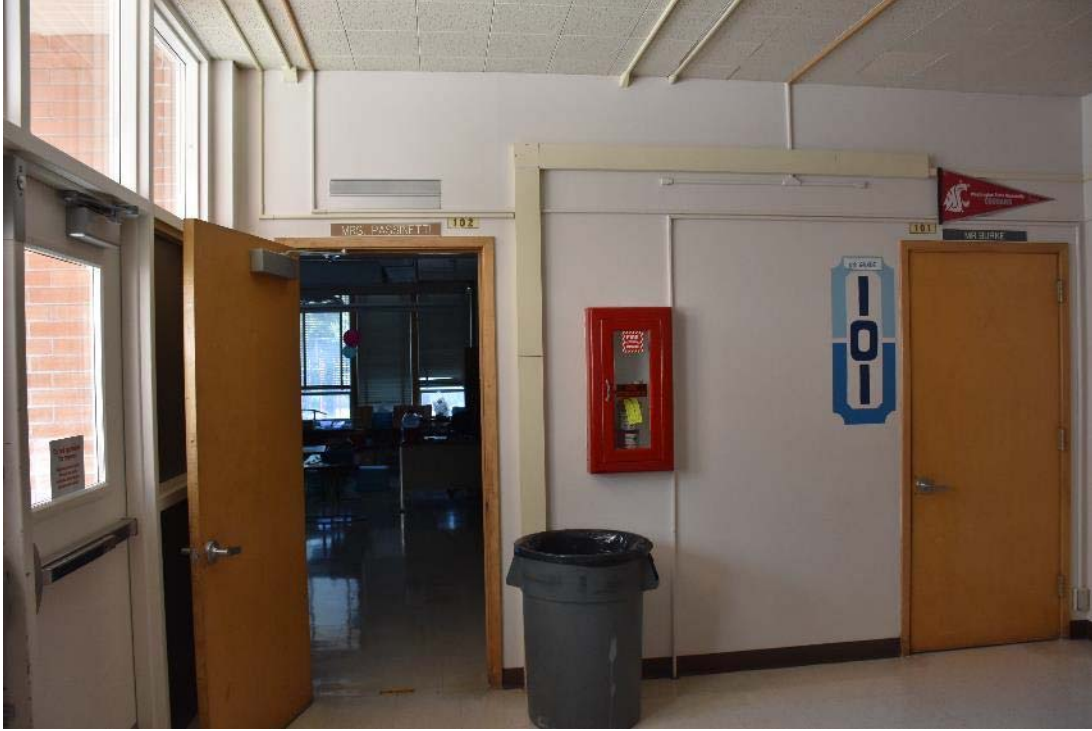
21. Entries to 1961 classroom wing, looking southwest
