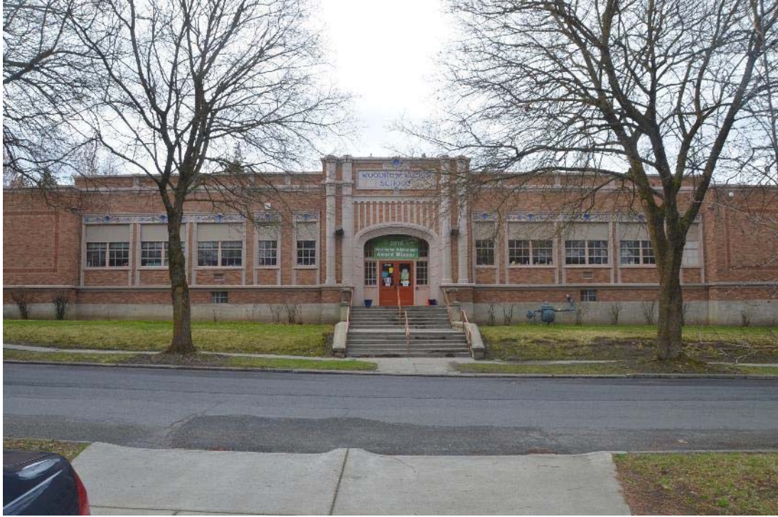
9. Front facade (north) showing main entry, looking south
