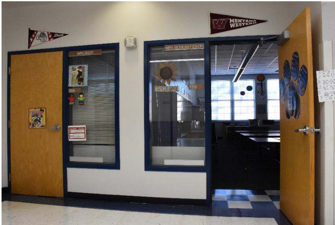
18. Looking west at entries to classrooms in 1999 wing
