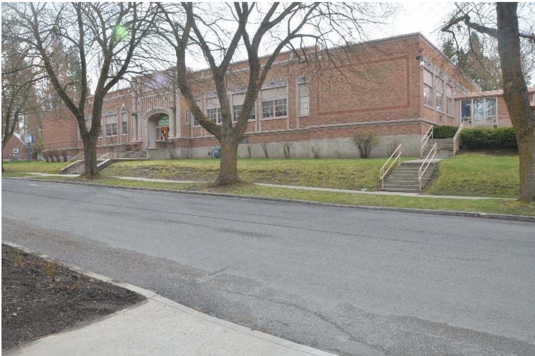
8. Front facade and corridor to multipurpose room, looking southeast
