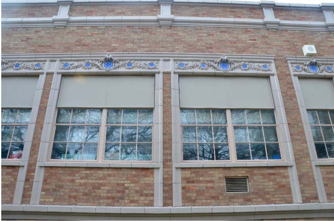
13. Detail of window bays on front facade, looking south
