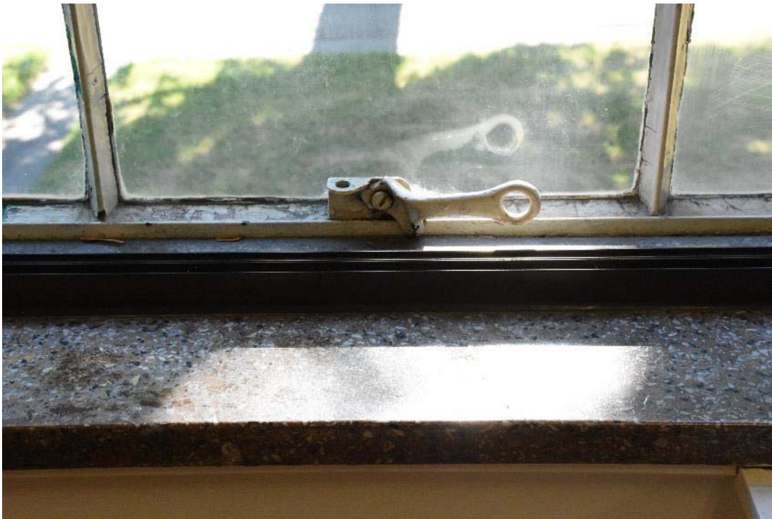
10. Detail - window latch, steel sash, and terrazzo sill
