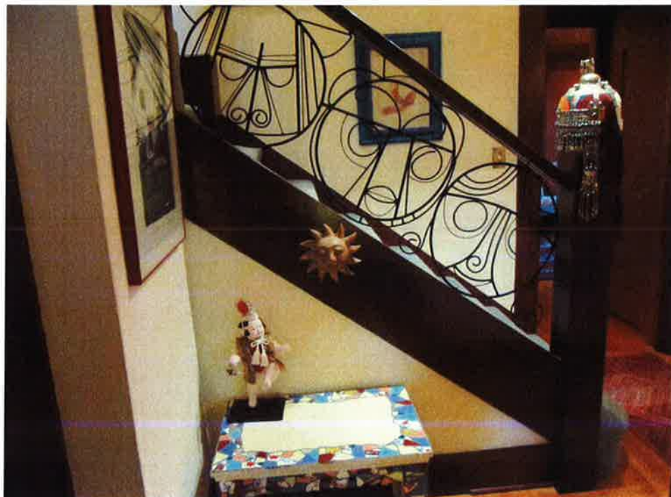
29 of 36 entry hall balustrade in 2013
