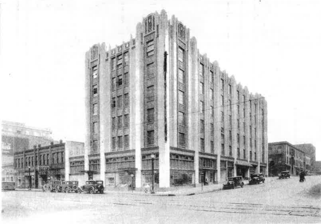
City Ramp Garage, Northeast corner, c.1930
