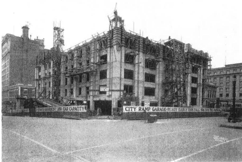
City Ramp Garage, Construction, c.1928
