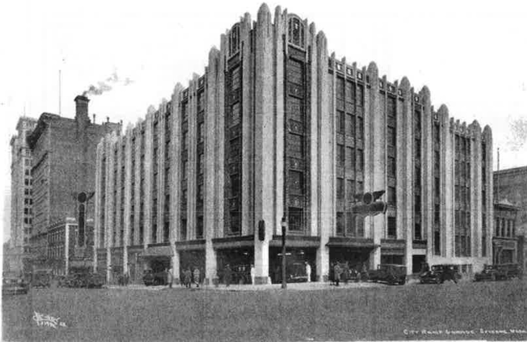
City Ramp Garage, Southeast corner, c.1930
