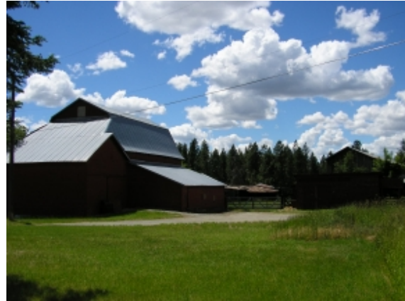
southwest- barn and outbuildings
