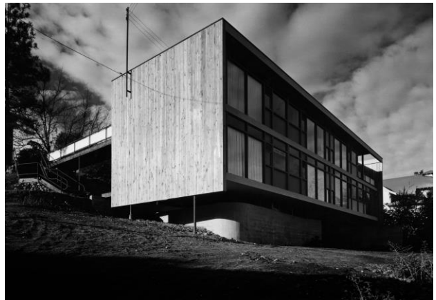
Photograph by Dearborn Masser. Year approximate. Northeast corner
