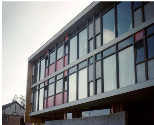
Photograph by Bruce Walker. Year approximate. Glass and panel curtain wall 1960
