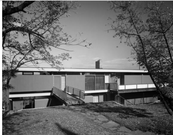
Photograph by Dearborn Masser. Year approximate. South facade
