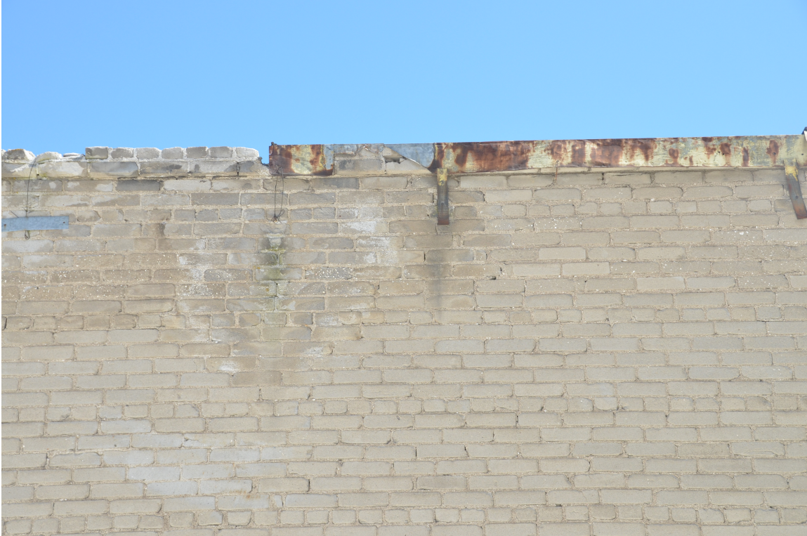
17. Parapet and Sheet Metal Coping on West Wall
