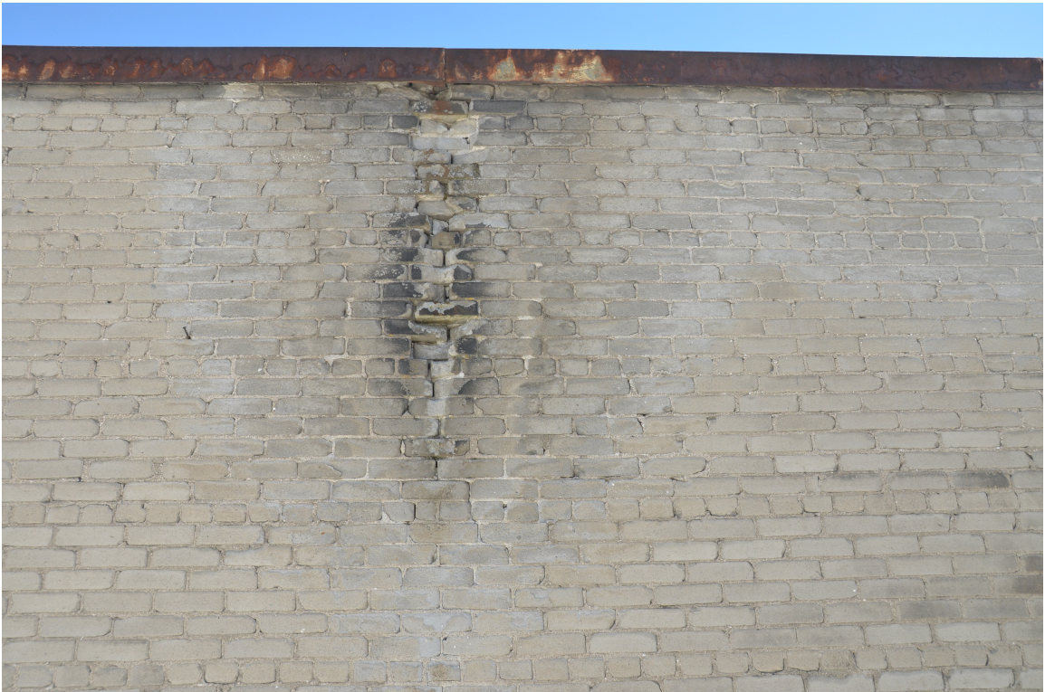
16. Parapet on West Wall Showing Brick Erosion and Rusted Sheet Metal Coping
