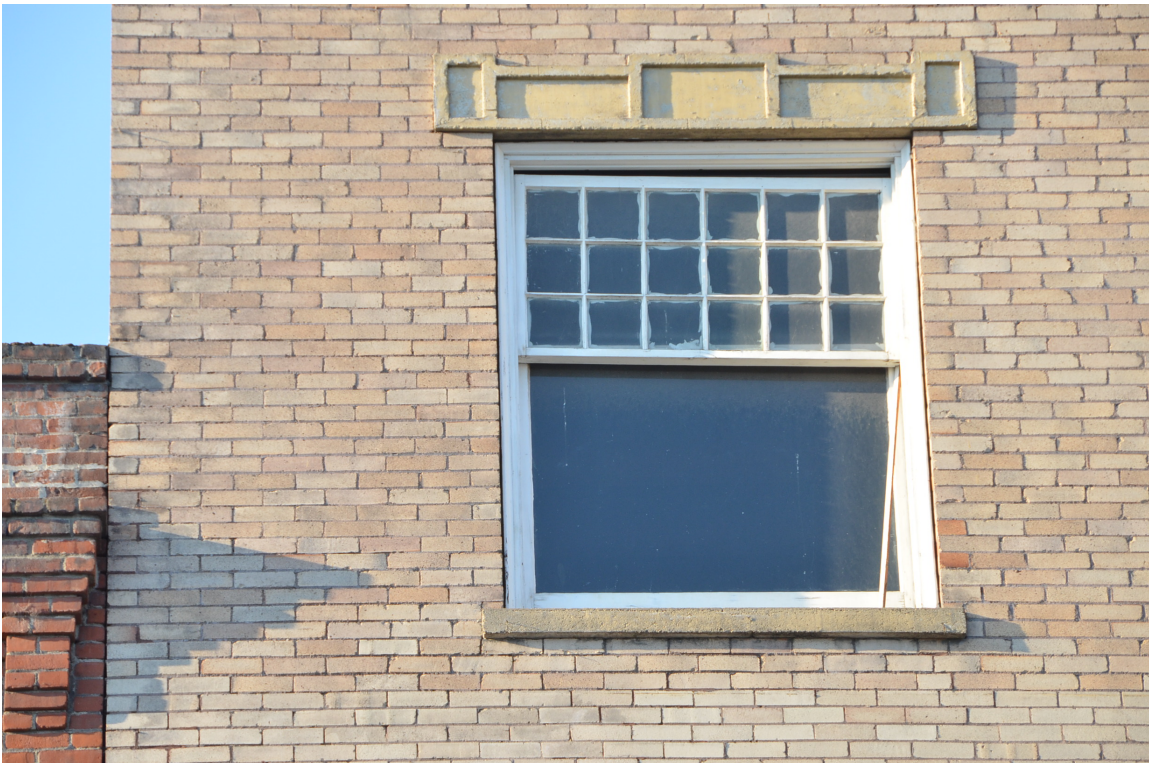
8. Front Facade 4th Floor Window Sash, Sill and Head
