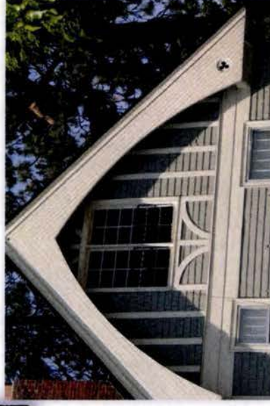
A barge board hides the eaves of this home at 2003 W. Third. Also note the string course that acts as a lintel above the windows and visually separates floors.
