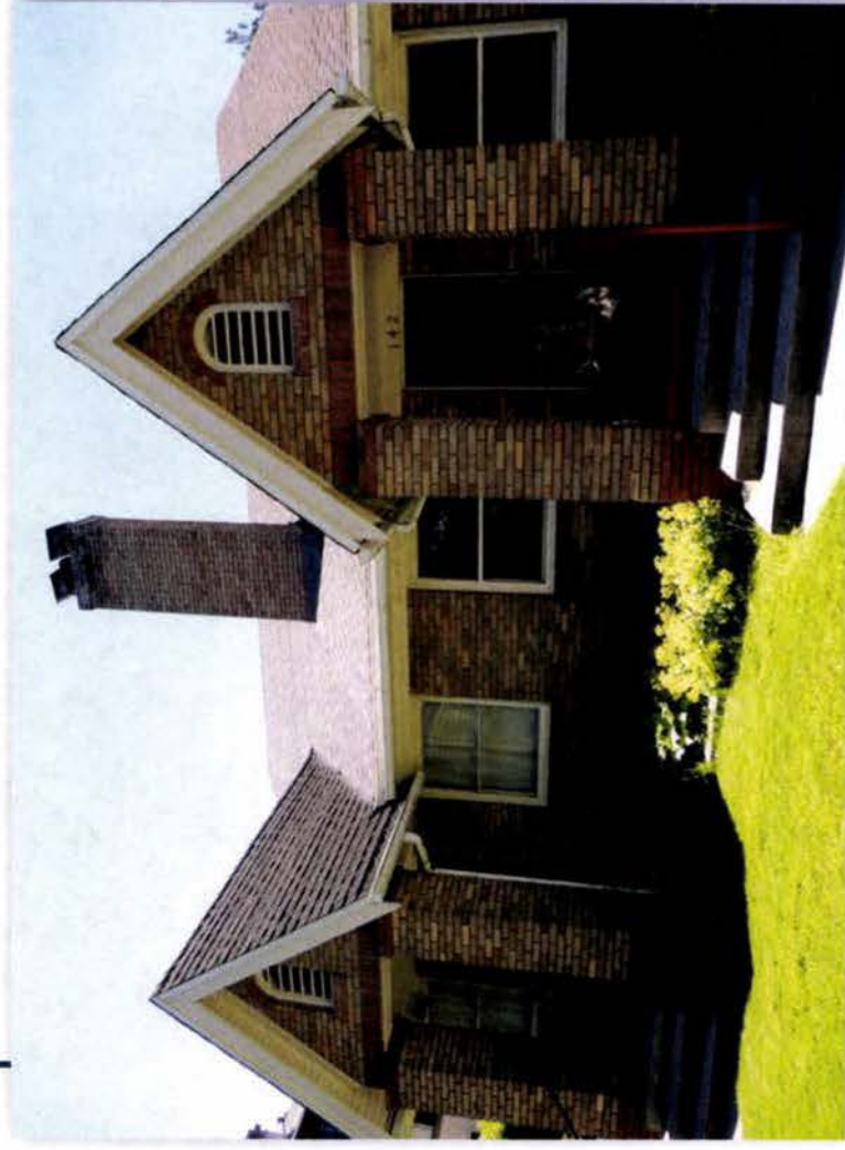
The duplex at 142-144 S. Poplar Street retain original wood 1:1 double hung windows.
