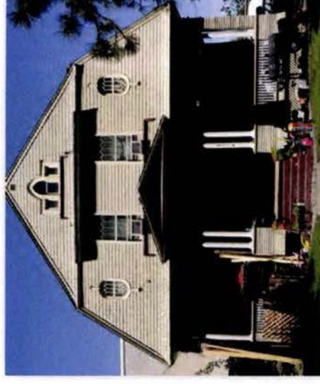
The house at 2114 W. First Avenue has a gambrel style roof.
