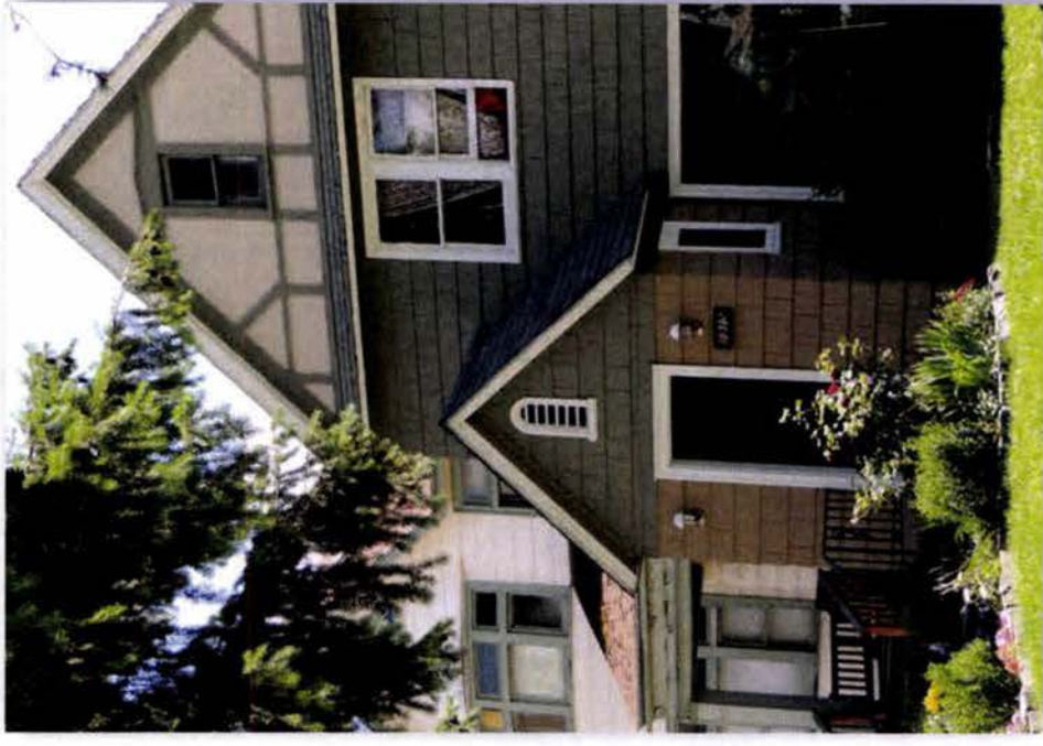
This home at 1915 W. Second was remodeled in 1936 and the original full-width front porch was removed and the entry portico was added.
