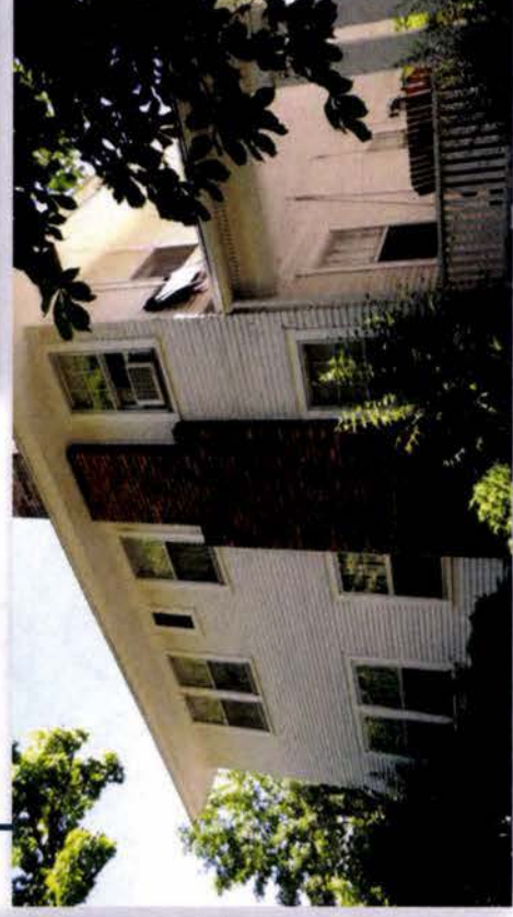
The house at 2328 W. Pacific Avenue shows a hip roof, boxed eaves, clapboard siding, dentil molding and the soffit under the front porch roof.
