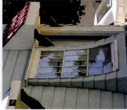
Brackets on the building at 1623 W. First
