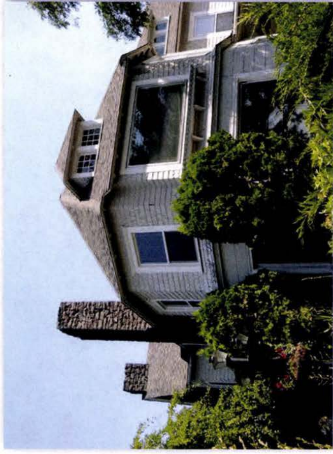
Top: 2218-2222 W. Fifth Ave: Dormer on a polygonal bay roof
