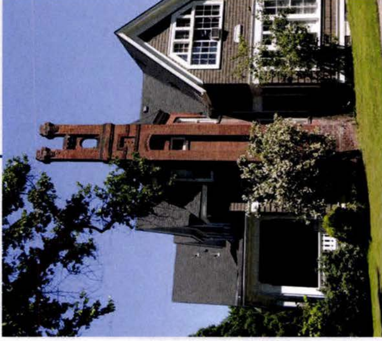
1725 W First Ave: The Glover House has probably the most distinctive corbeled exterior brick chimney in the district.
