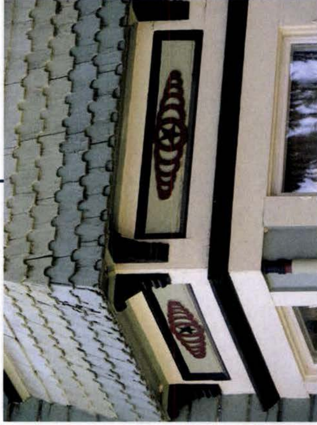
1631 W First Ave: showing decorative shingles, brackets and moldings.
