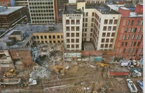
Workers load rubble from the Rookery Building into trucks on Tuesday as a crew removes the Mohawk Building's asbestos roofing.
