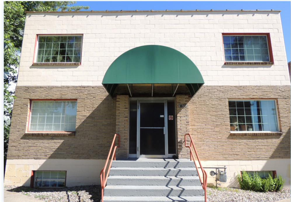
Windows at the small apartment building at 1908 W Second Avenue have been changed to internal grid vinyl sash. The impact of these inappropriate windows is heightened on such a small building.
