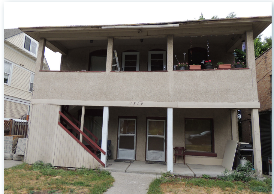
This multi-family apartment building at 1714 W Pacific is clad with stucco that has been applied over the original brick; that, combined with complete window replacement, has resulted in its non-contributing status.
