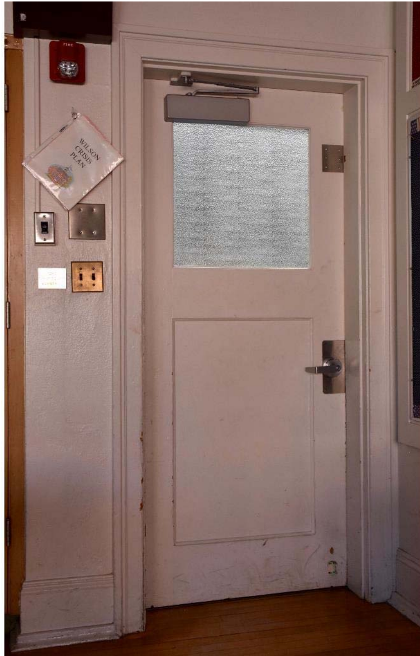
23. Detail - 1161 Original door and moldings in northwest corner classroom
