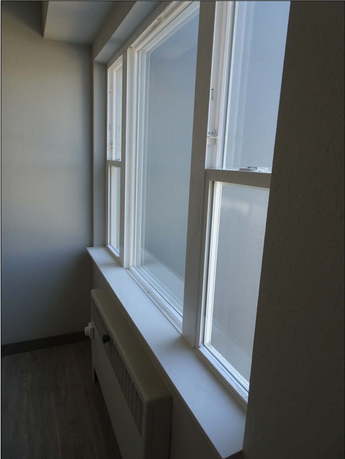
Typical apartment window and restored 1952 steam-heat wall radiator, looking northwest
