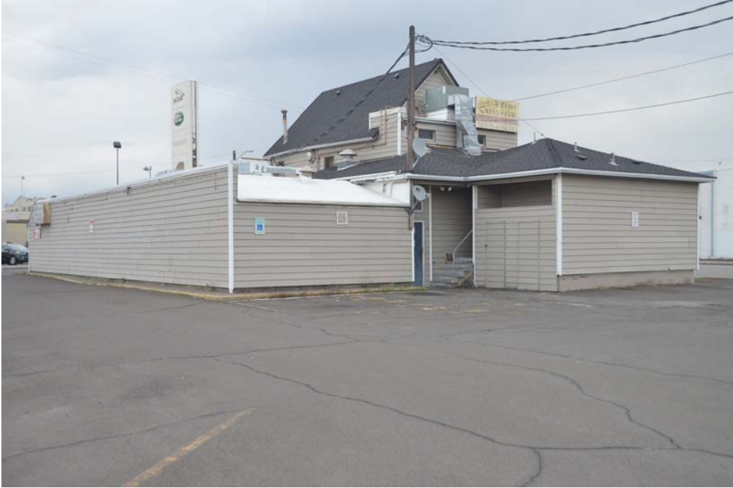
11. Southwest corner, looking northeast
