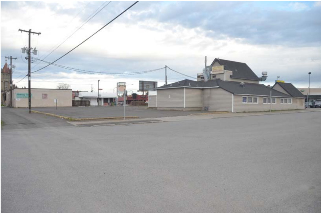
14. Southeast corner of site, Adams Street and alley
