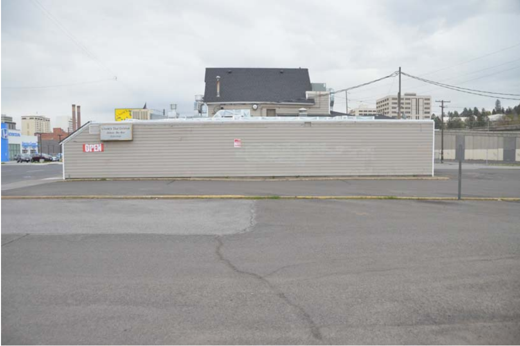
9. West facade, looking east
