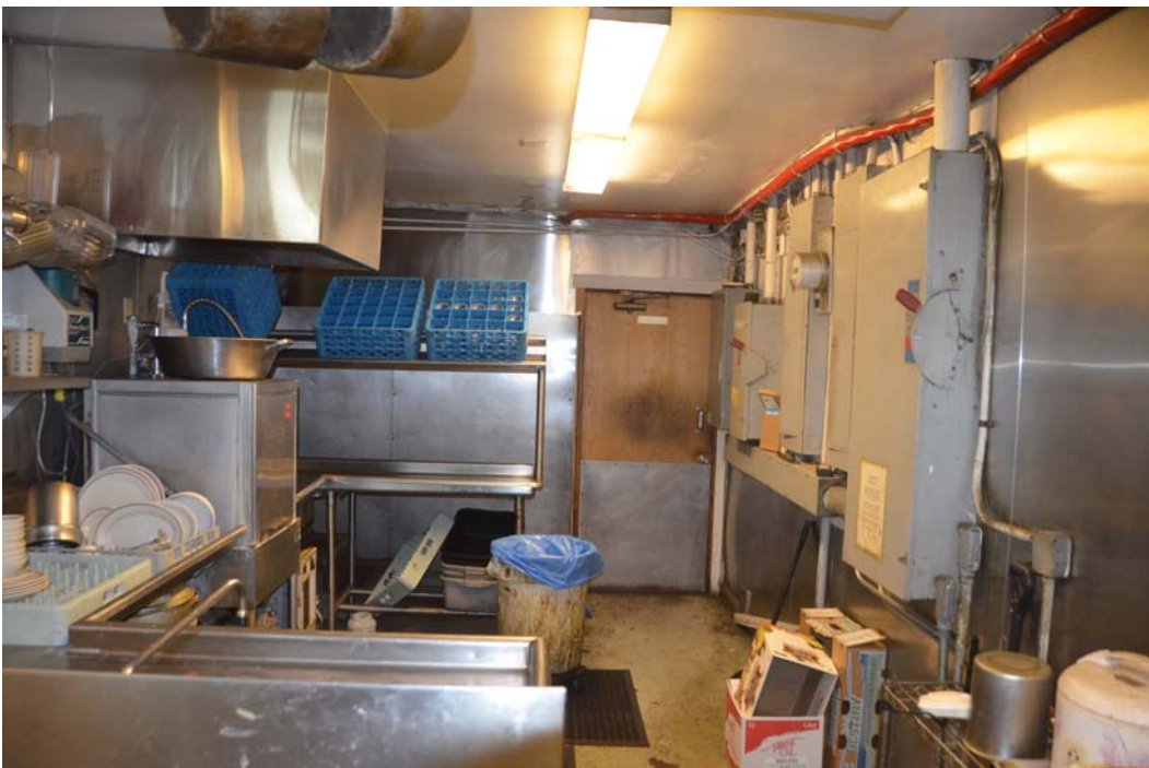
38. Kitchen southwest corner, dishwashing and electrical panels
