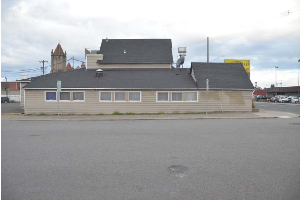
17. East facade, looking west
