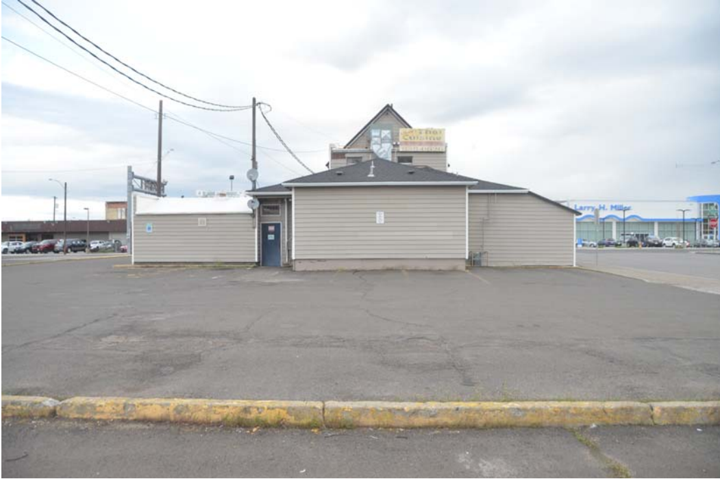
13. South facade (rear), looking north
