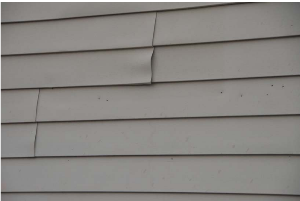
10. West facade, vinyl siding
