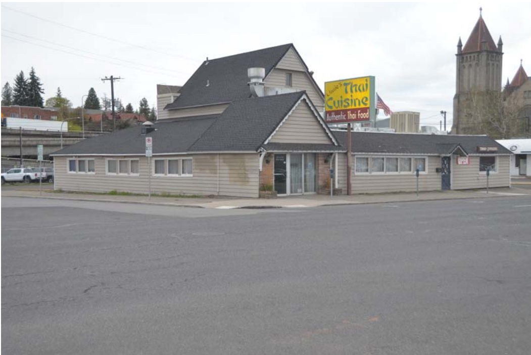
2. Northeast Corner, looking southwest
