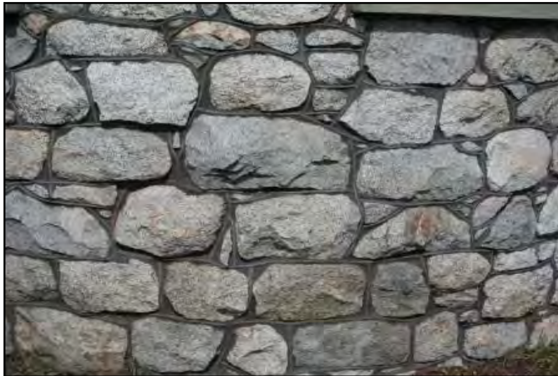
Figure 8: Convex beaded mortar joints in granite at 527 E. Nora Avenue, Spokane
