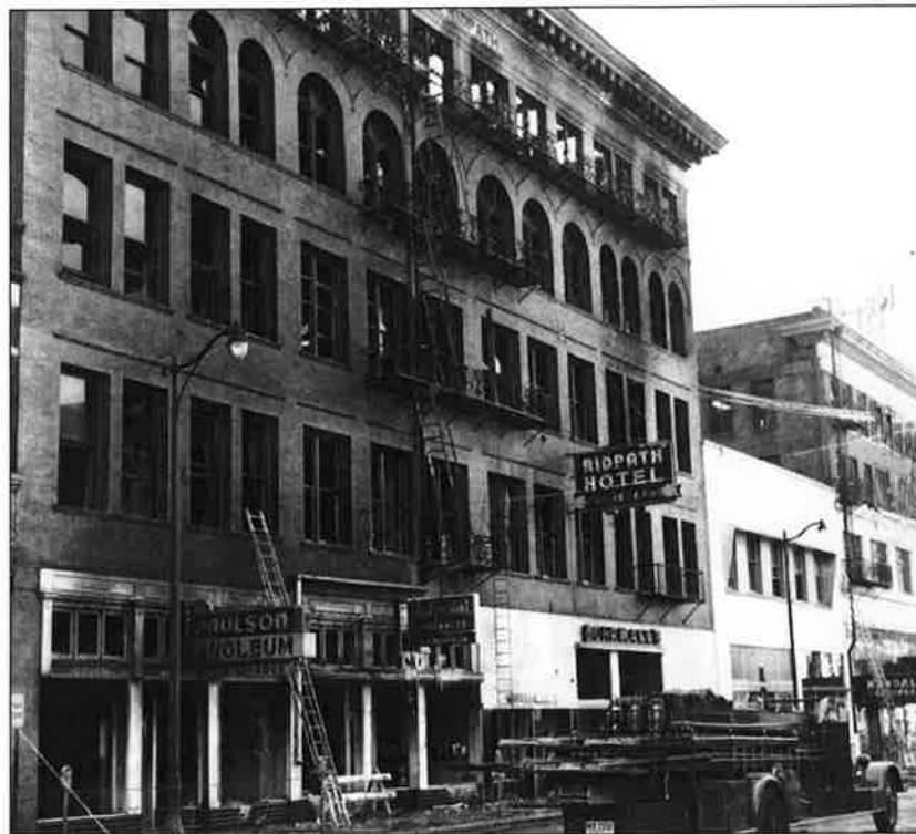
1950 photo of fire damaged Ridpath Hotel
