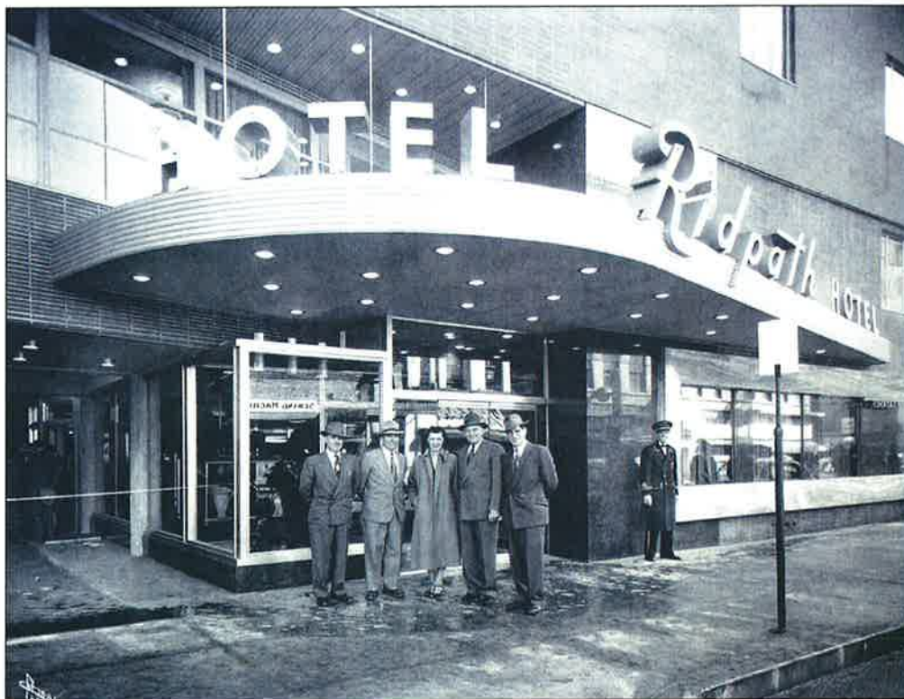
c.1952 photo of Ridpath Hotel, main entry facade
