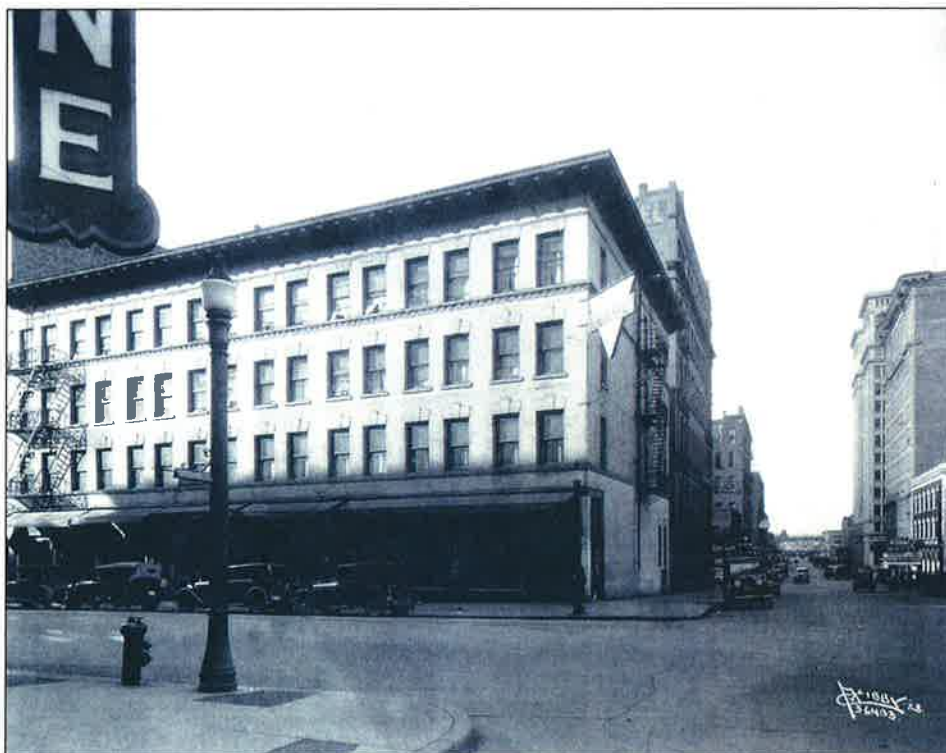
1925 photo of the East Wing /YWCA, south facade (later owned by the Ridpath Hotel in 1937)
