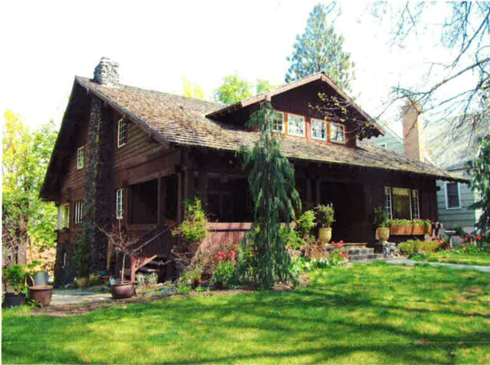
2 of 20: southwest corner of house in 2014
