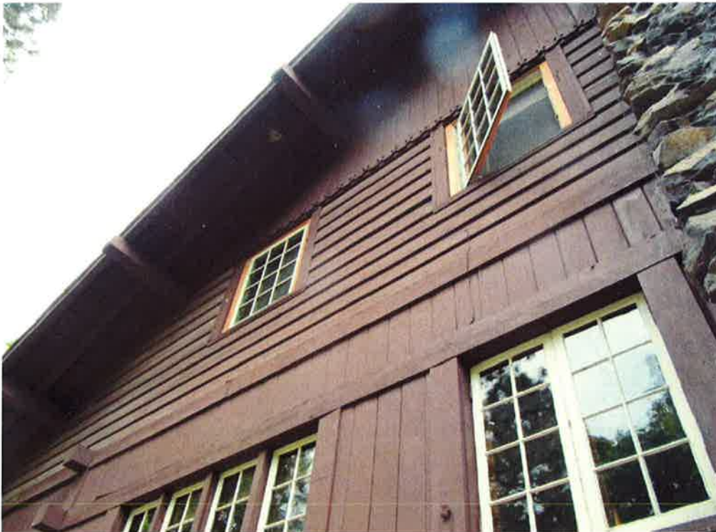
4 of 20: west gable peak detail
