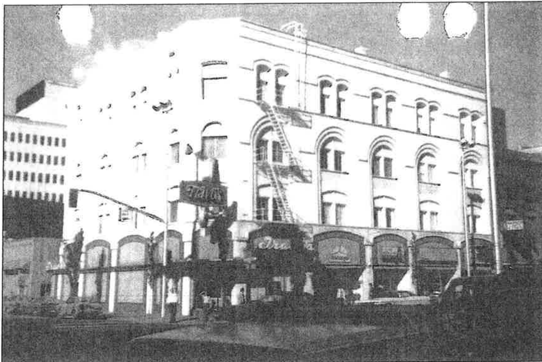
1963 photo of Germond Block, southwest corner façade
