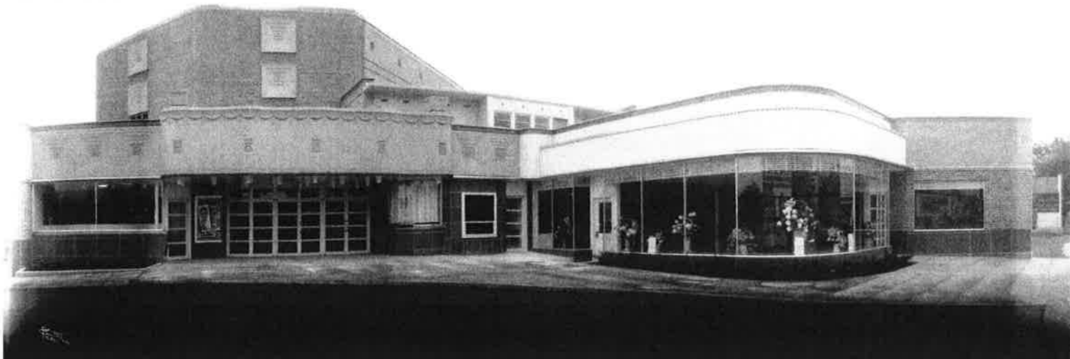
Circa 1945. Garland Theater. South (main) façade. View: Looking northeast. Source: Northwest Museum of Arts & Culture.
