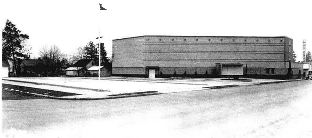
Circa 1945. Garland Theater. Northeast (rear), Northwest (rear), and west (side) facades. View: looking southeast. Source: Garland Theater.
