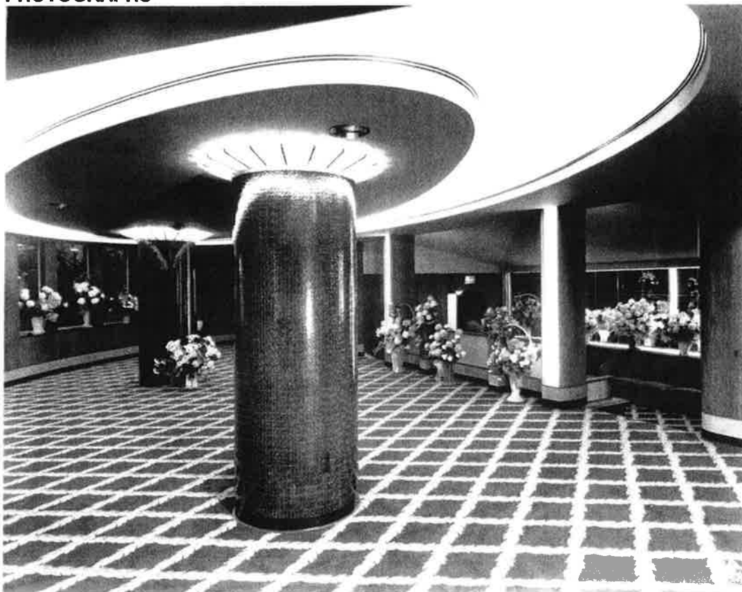
Circa 1945. Garland Theater. Foyer (southwest). View: looking north. Source: Garland Theater.
