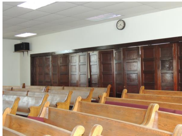
These large paneled doors, could be stretched out (like the picture) or be folded back like an accordion depending on the need. Photo taken May 29, 2015. Interior Doors 2015
