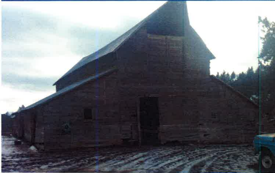
north side of barn
